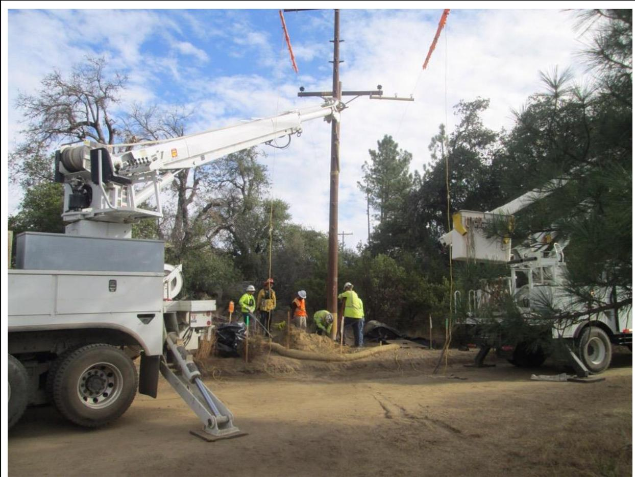
**Photo 1:** A construction crew observed setting a direct bury steel pole (C 442). Fiber rolls were present and functional in accordance with the project's Erosion Control Plan, SWPPP (MM HYD-1, MM BIO-7) and APM HYD-09.
