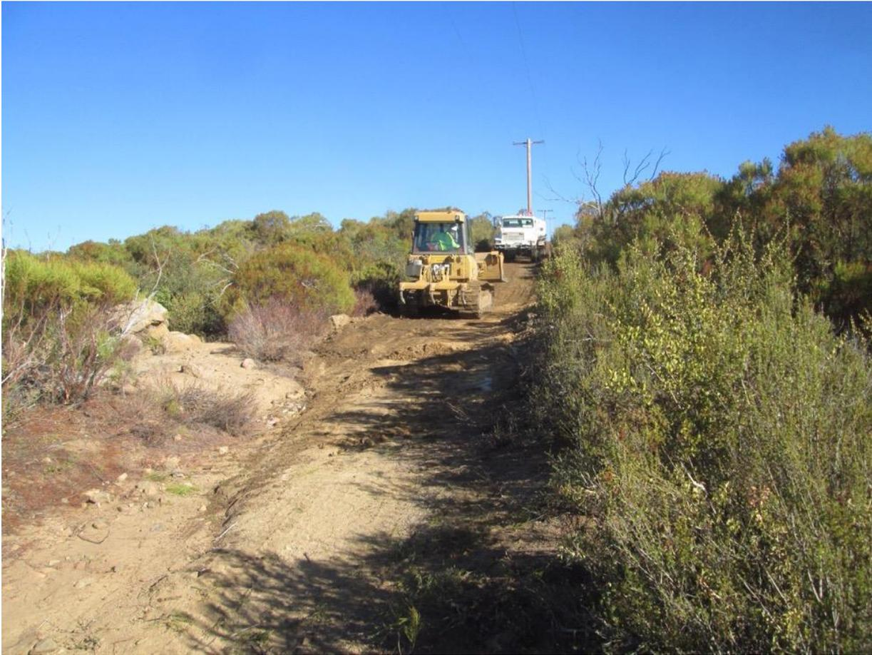
**Photo 4:** During the grading and maintenance of an existing access road between Poles P176961 to P176964 (C 442), a water tender was used to prevent dust emissions in accordance with APM AIR-02.
