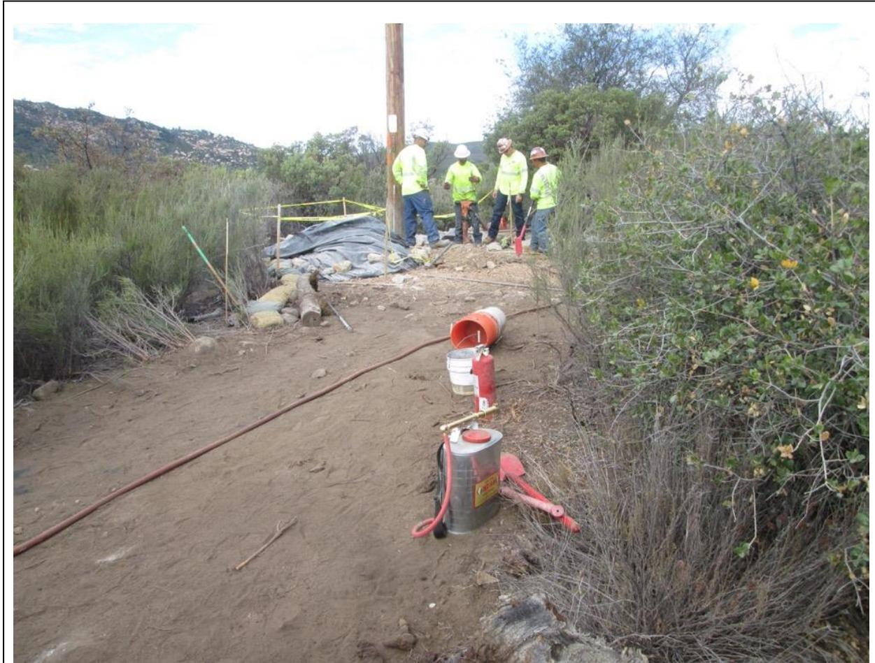
**Photo 2:** A construction crew observed trenching and installing ground rods at Pole P177017 (C442). The crew was observed staging the required 5-gallon backpack pump, round point shovel, Pulaski, and 2A10BC fire extinguisher, along with 100 gallons of water and pump hose (not pictured) in accordance with the Fire Prevention Matrix (off CNF land), CFPPP (MM FF-1 and APM HAZ-01), and APM HAZ-04.
