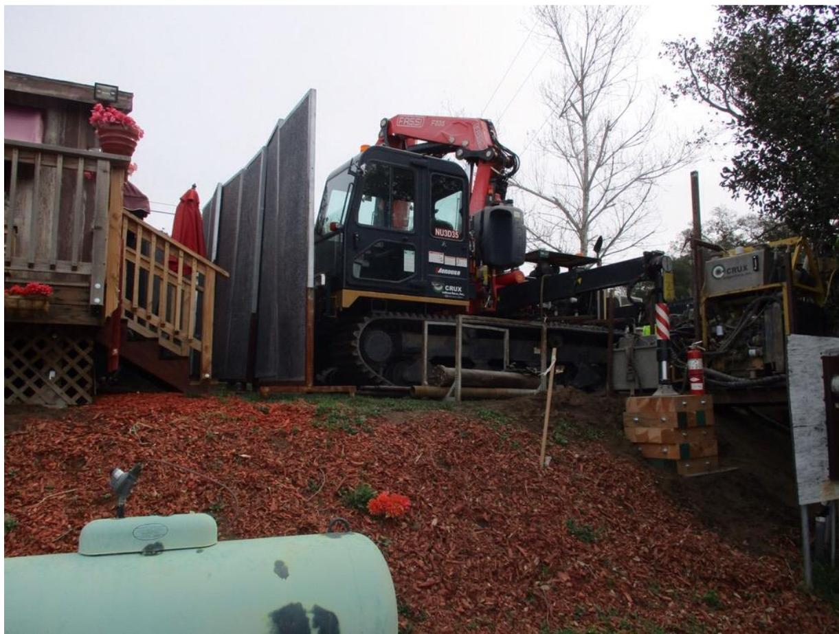
**Photo 5:** Noise barriers were observed being used during micropile drilling activities at Z118042 (TL 682) to minimize noise disturbance at an adjacent residence, in accordance with MM NOI-1.
