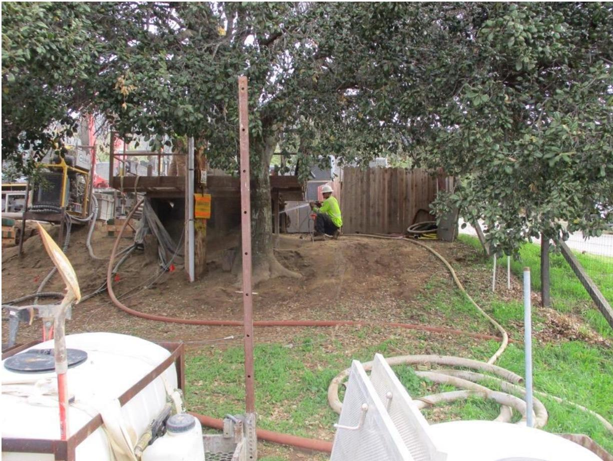
**Photo 1:** During micropile drilling at Z118042 (TL 682), a crew member was observed spraying water in a drill hole to reduce dust in accordance with APM AIR-02.
