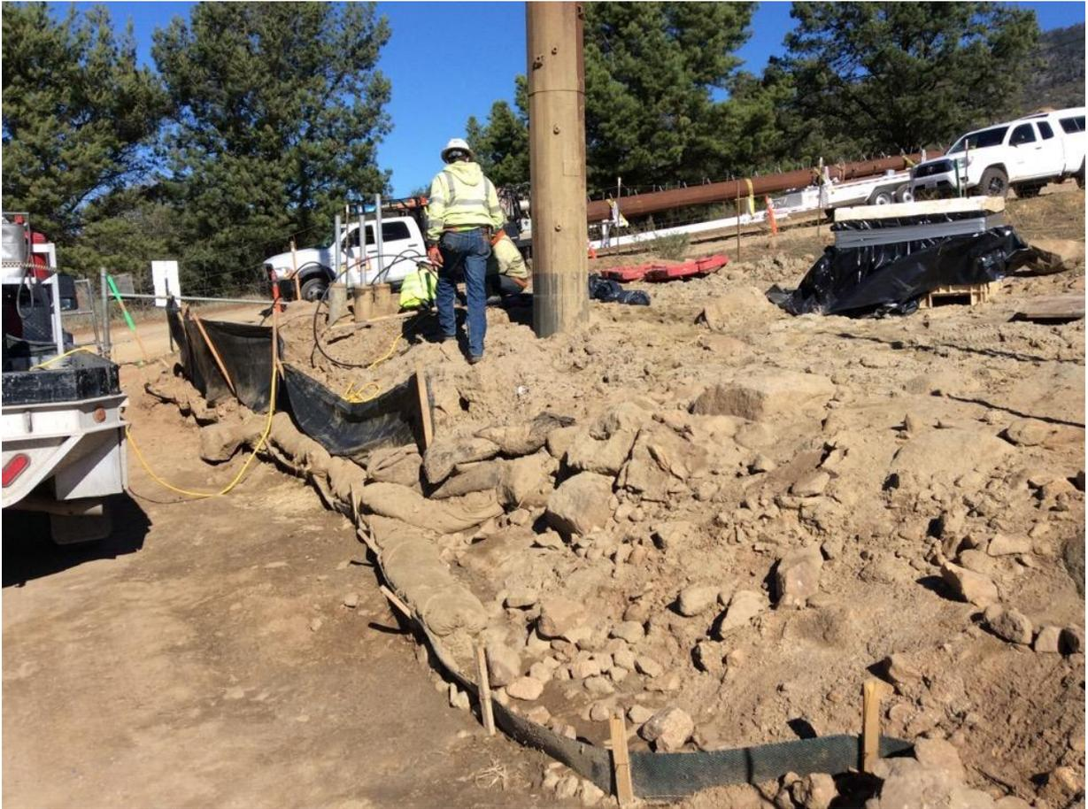
**Photo 4:** During capping at Pole Z118051 (TL 682), erosion control BMPs were observed to be in need of maintenance. The project Lead Environmental Inspector was notified, and BMPs were subsequently repaired.
