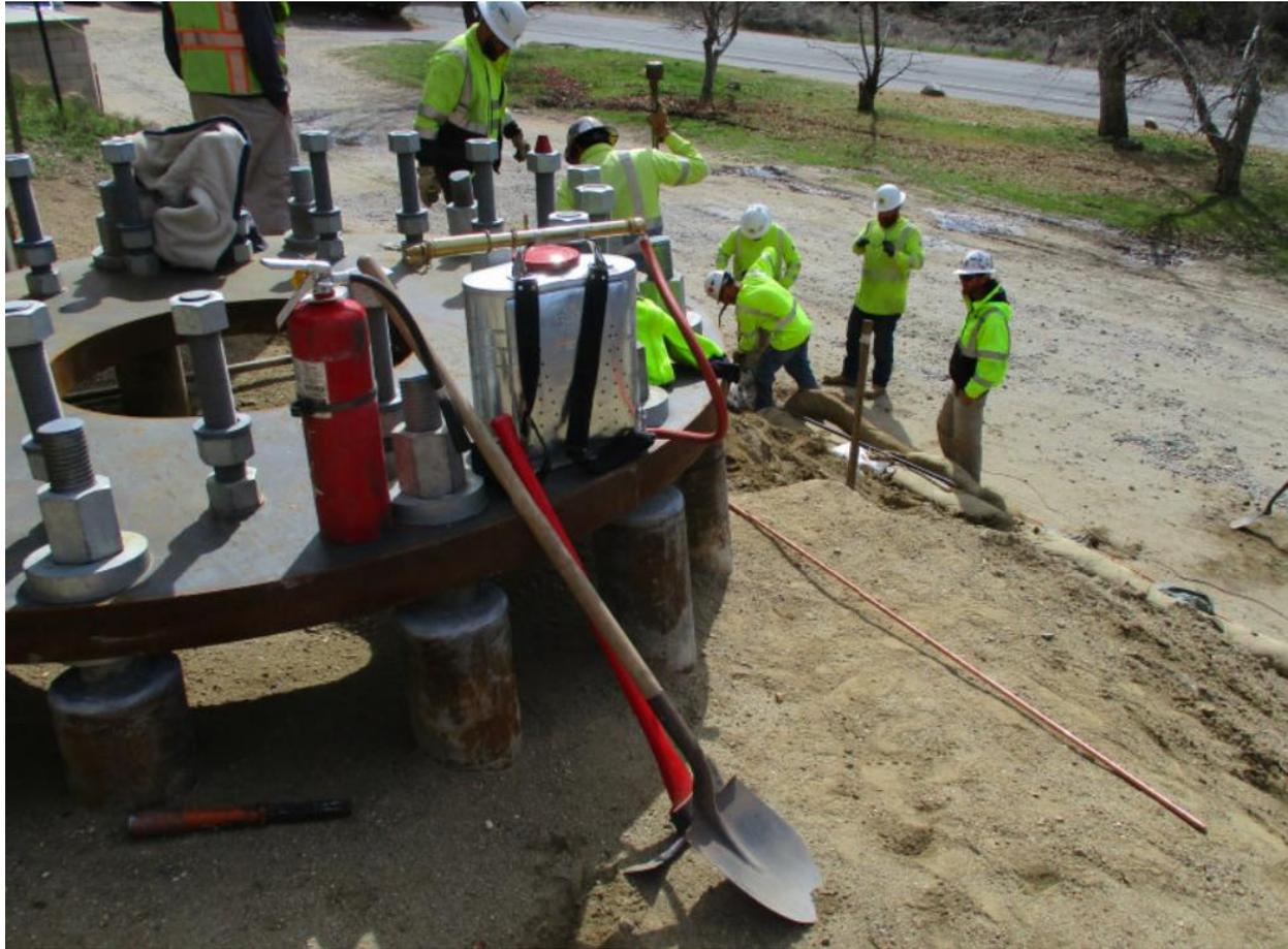
**Photo 3:** A set of fire tools (5-gallon backpack pump, round point shovel, Pulaski, and 2A10BC fire extinguisher) was observed at active construction sites in accordance with APM HAZ-01 and APM HAZ-04 during ground wire and rod trenching at Z118106 (TL 682).
