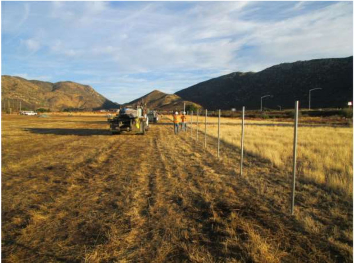
Photo 6: Installing fence posts at the Anderson Staging Yard.
