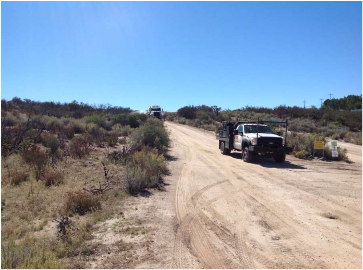
Photo 1: Water was applied to the access road to Pole Z44228 prior to crew ingress per APM AIR-02 (truck is shown here exiting the area). Signage showing approved access roads was observed.
