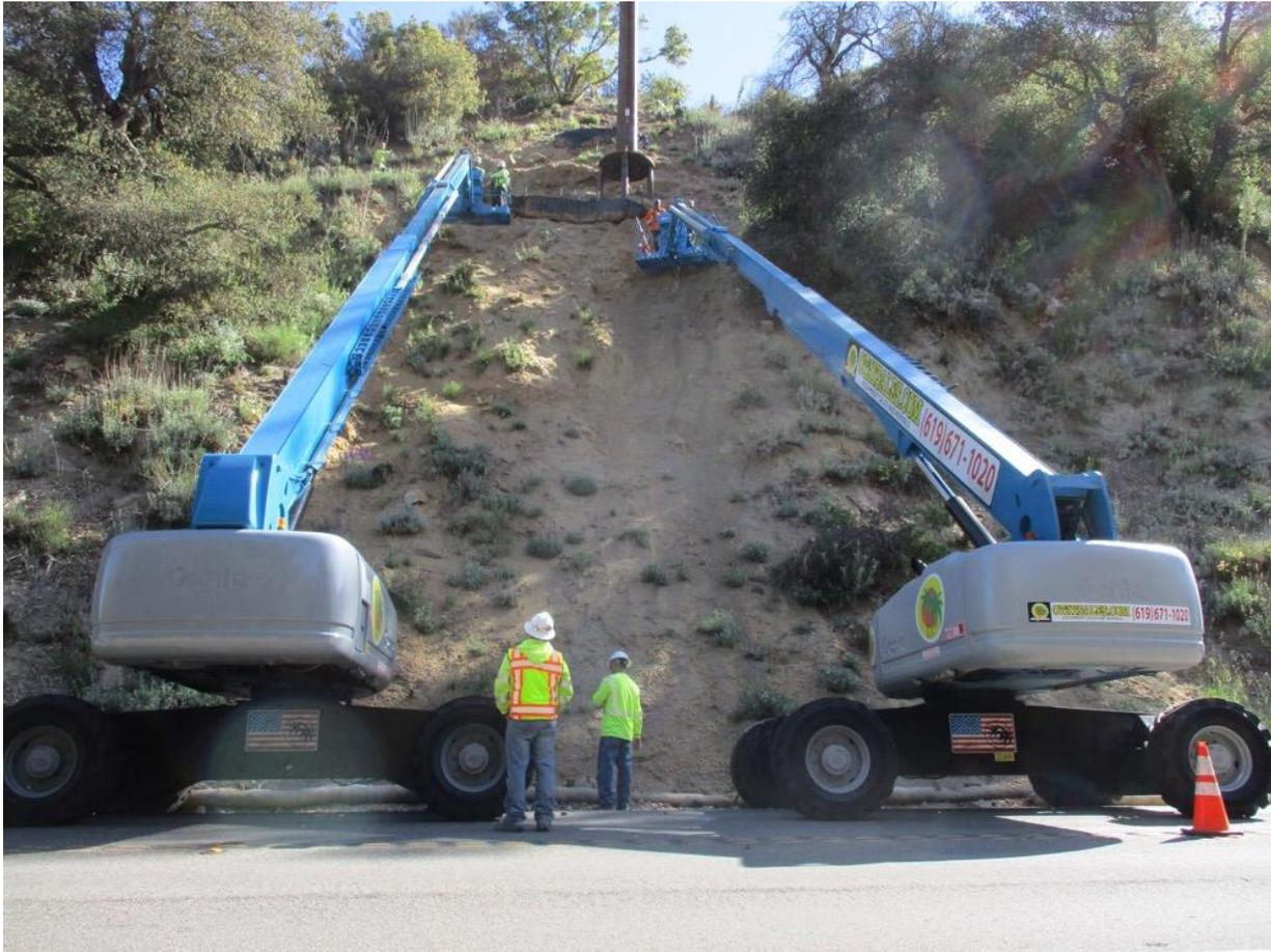
**Photo 6:** A crew installing fiber rolls and preparing to apply hydro-mulch on the steep slope at Z118138 (TL6957) to prevent erosion, in accordance with the Erosion Control Plan and SWPPP.
