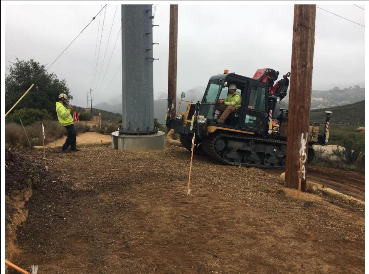
**Photo 1:** Crews position a crane atop pole site Z105008 (TL6957) in order to set up a drilling platform and associated equipment to drill micropile foundations. Biologists were observed on site working with crews as they set up within the work limits, in accordance with MM BIO-1 and MM BIO-22. Straw wattles moved for equipment mobilization were observed reinstalled in accordance with the SWPPP (MM HYD-1).
