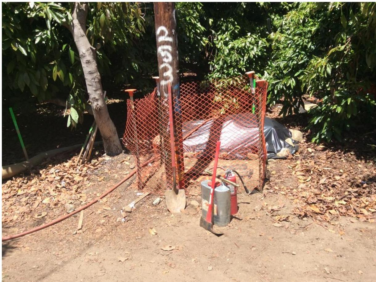
**Photo 6:** The spoils stockpile from the pole hole at Pole P611298 (TL682) was covered with visqueen secured with rocks to prevent erosion in accordance with the ECP and SWPPP (MM HYD-1, MM BIO-7). In addition, the hole was securely covered to prevent wildlife pitfalls, in accordance with MM BIO-23, and a complete set of fire tools was staged on site in accordance with the CFPPP (MM FF-1).
