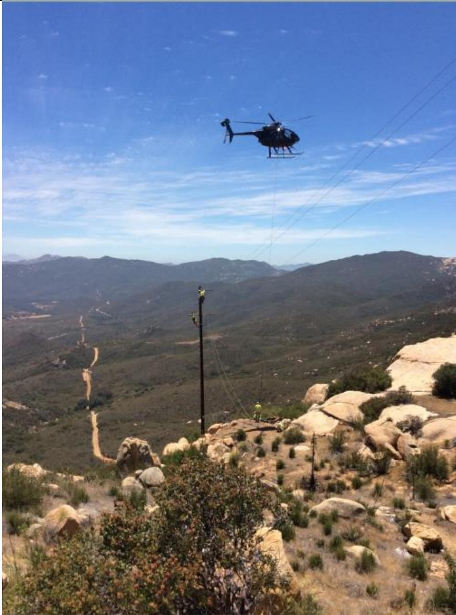
**Photo 1:** Crews were observed conducting helicopter-assisted wire spreading activities at Pole Z571429 (TL 6957).
