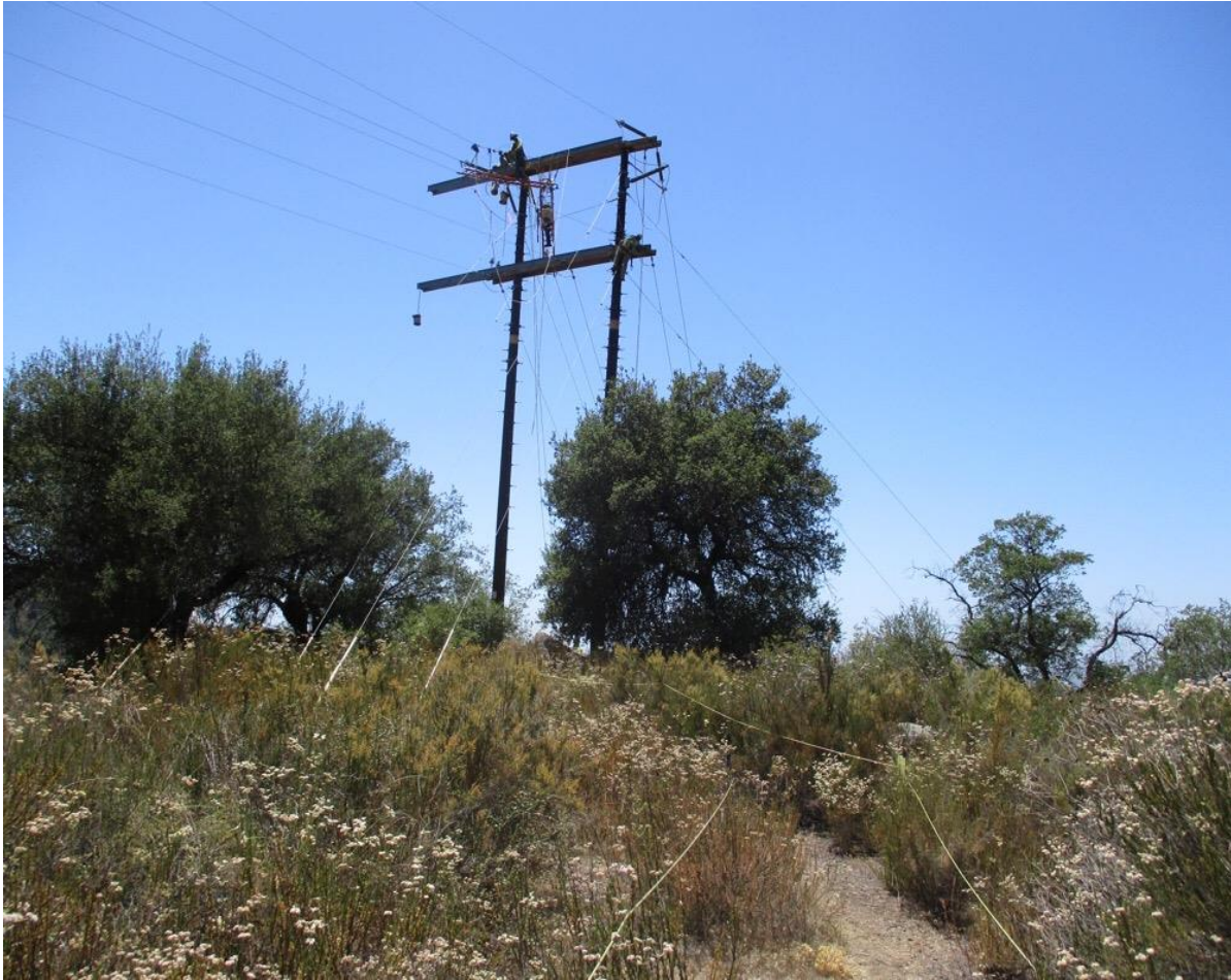
Photo 5: A crew was observed spreading wire at Z118024 (TL 682) to allow for the overhead space necessary for the helicopter transport of drilling equipment to the site. To prevent workers from entering an environmentally sensitive area (ESA), the footpath and workspace were delineated with yellow rope and ESA signage in accordance with the Historic Properties Management Plan (MM CUL-1).
