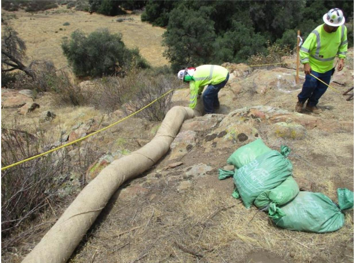
**Photo 6:** Crews were observed installing fiber rolls along the downslope side of the site at P 278746 (C 157) for sediment control in accordance with the Erosion Control Plan and SWPPP (MM HYD-1, MM BIO-7, and APM HYD-09). To prevent potential impacts to cultural resources in accordance with the HPMP (MM CUL-1), gravel bags were used to secure the fiber rolls to the ground surface instead of shoveling a shallow trench and then pounding in wooden stakes.
