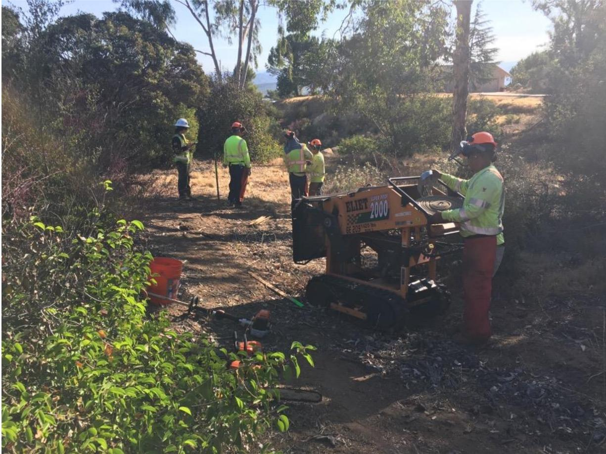
**Photo 3:** A biological monitor was observed discussing work space limits with vegetation clearing crews at pole Z571426 (TL 6957) in accordance with MM BIO-1 and MM BIO-22. A construction crew member prepared a fire hose in order to pre-water vegetation around the area to be cleared in accordance with the CFPPP (MM FF-1).
