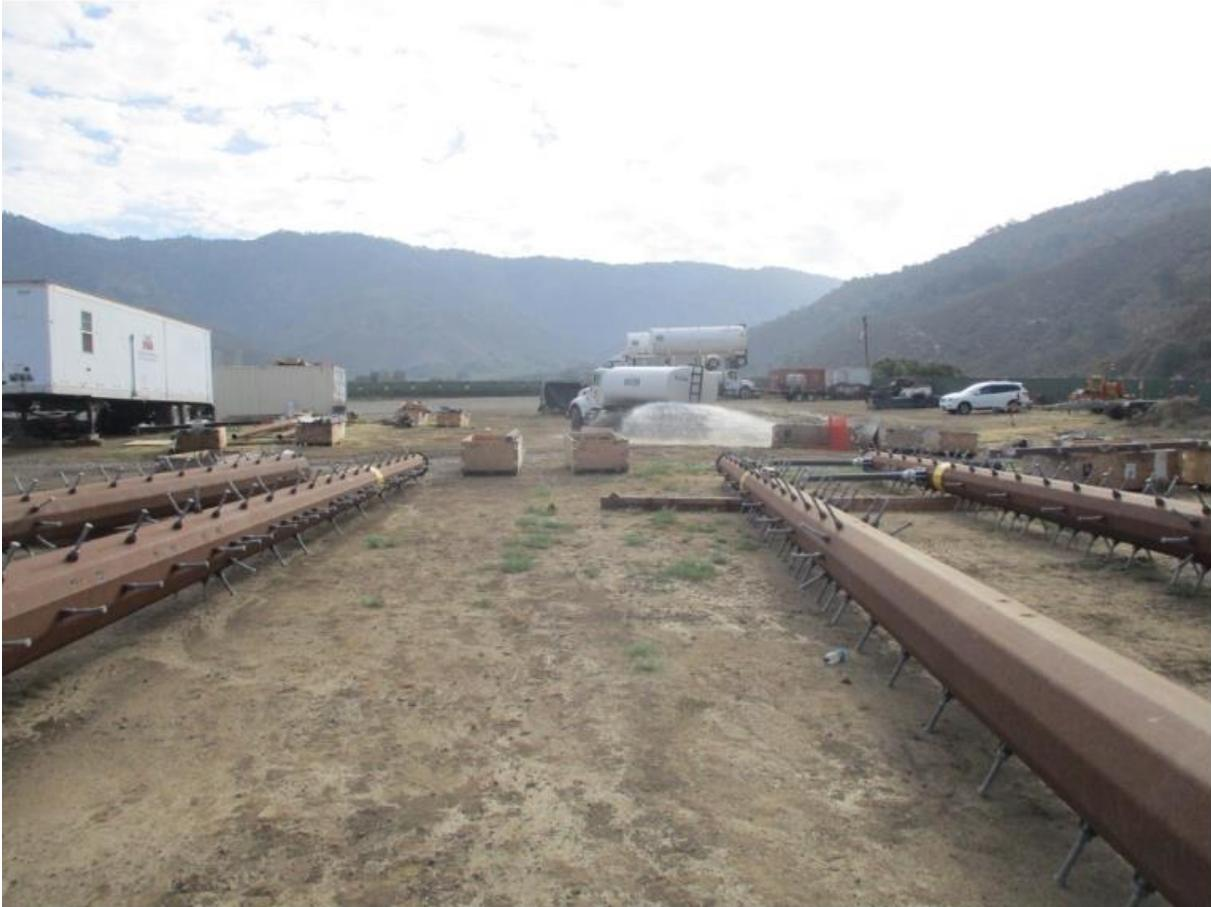
**Photo 1:** During loading of poles for transport at the Nursery Yard (TL682) a water truck was observed wetting the ground for dust control in accordance with APM AIR-02. Opaque green material around the staging yard fence (APM VIS-02) and SWPPP BMPs (MM HYD-1, MM BIO-7) were observed in good conditions.
