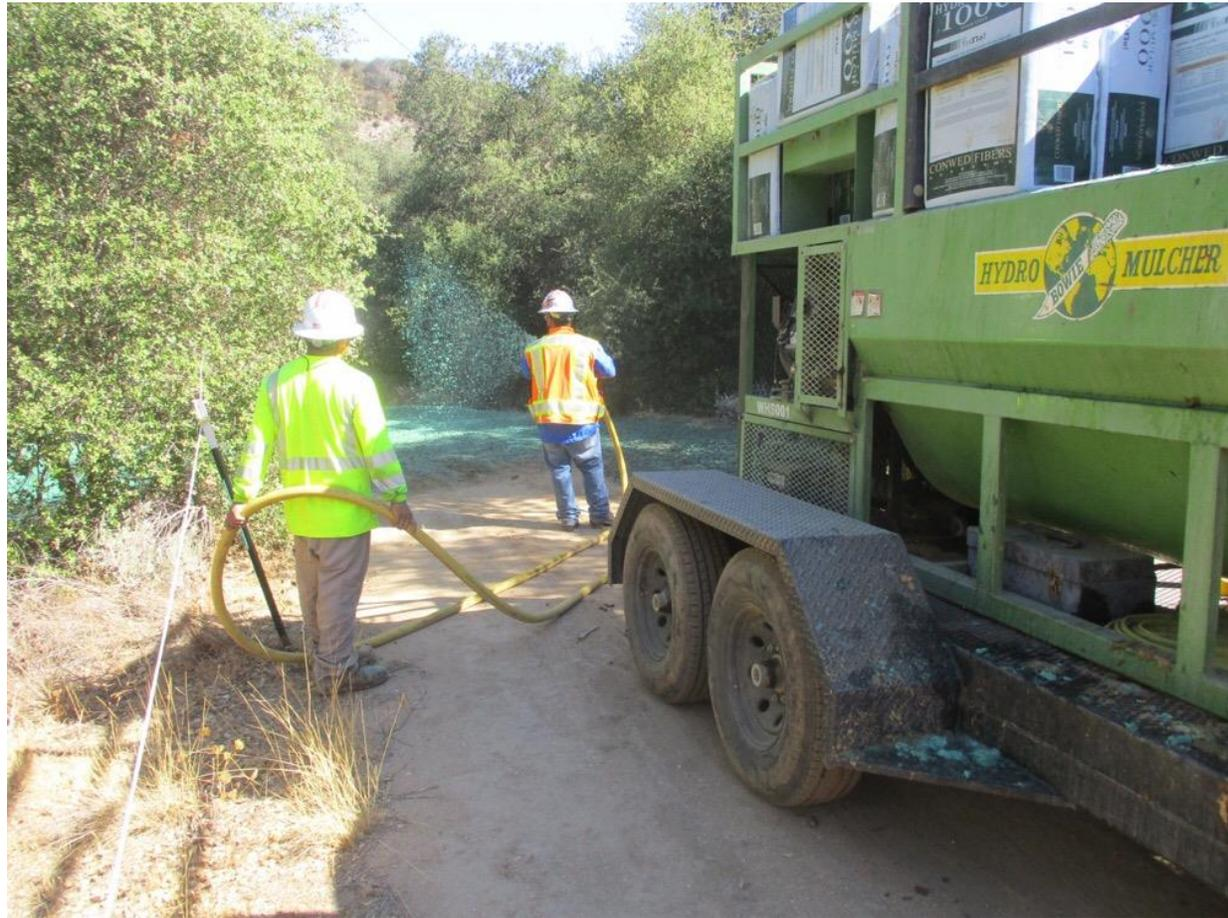
**Photo 2:** A crew is observed applying hydromulch at Z118153 (TL 682), in accordance with the Erosion Control Plan and SWPPP.
