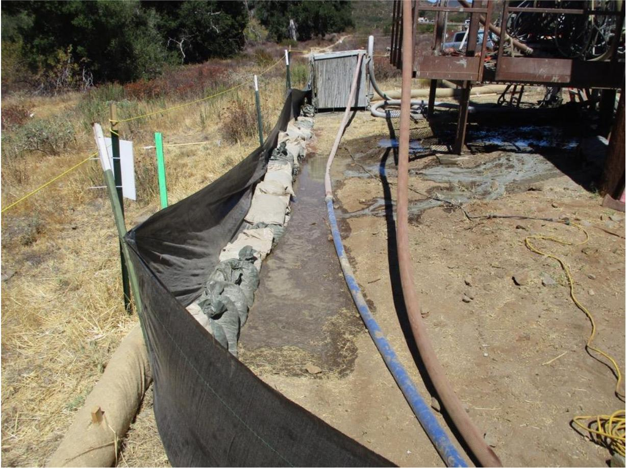
**Photo 5:** During micropile drilling at Z40517 (TL 629C), silt fencing and a gravel bag berm were installed along the downslope side of the work area to contain groundwater from being expelled from the drill hole, in accordance with the Erosion Control Plan and SWPPP.
