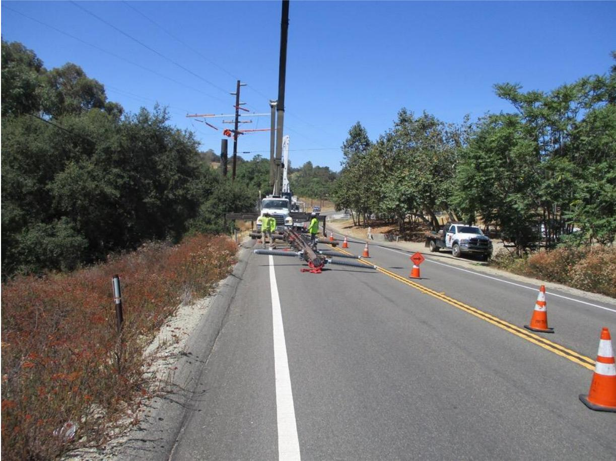
**Photo 6:** During pole framing and installation at Z112236, crews implemented a lane closure along Highway 76 in accordance with APM TRANS-02.
