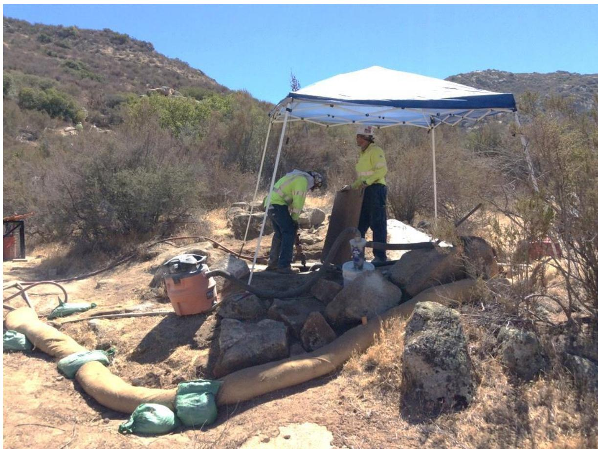
**Photo 3:** The hand digging crew at Pole P258090 (C 157) was observed using a containment system to capture dust emissions from rock jackhammering, in accordance with APM AIR-05.
