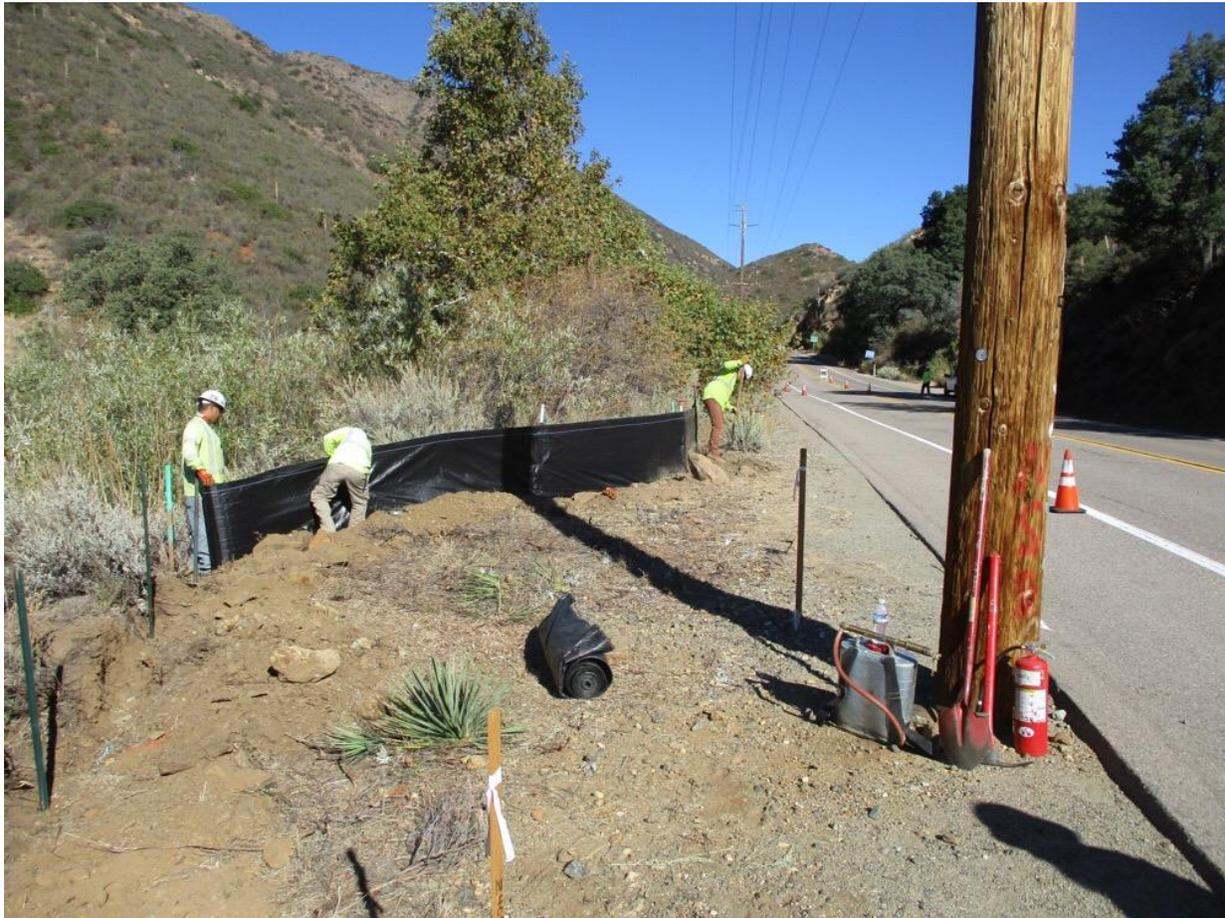
**Photo 3:** A construction crew observed installing silt fence at Z40506 (TL 629C) in accordance with the Erosion Control Plan and SWPPP (MM HYD-1, MM BIO-7) .
