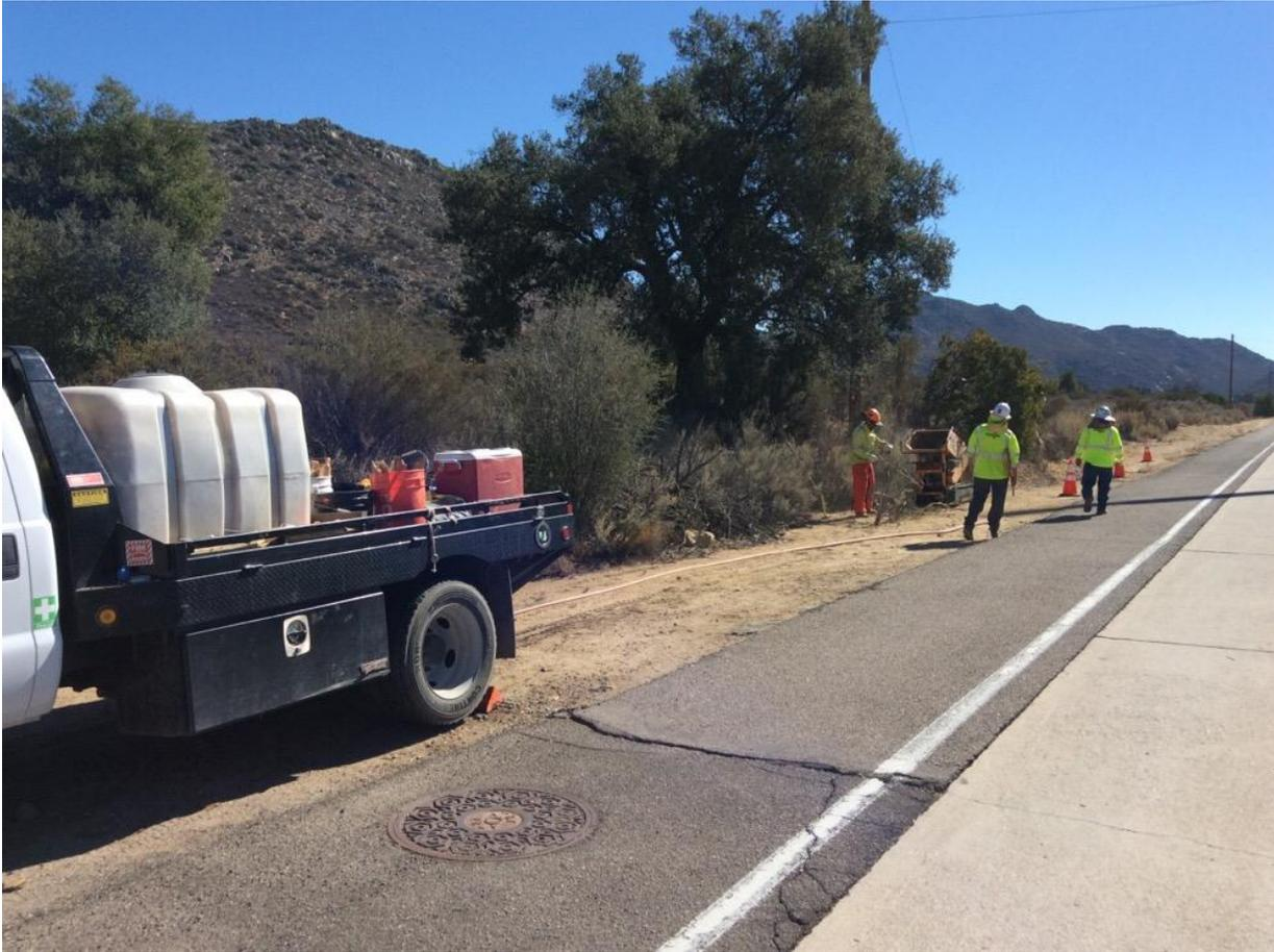
**Photo 5:** During vegetation chipping at Pole Z206014S (TL 629C), the crew was equipped with at least 100 gallons of water with a pump and hose, as required by the CFPPP Fire Matrix for the activity, location, and FPI.
