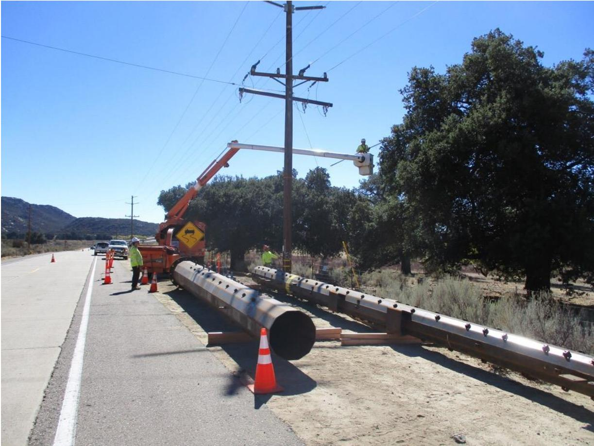
**Photo 4:** A construction crew observed trimming a nearby oak at Z40539 (TL 629C) for pole installation and line clearance.
