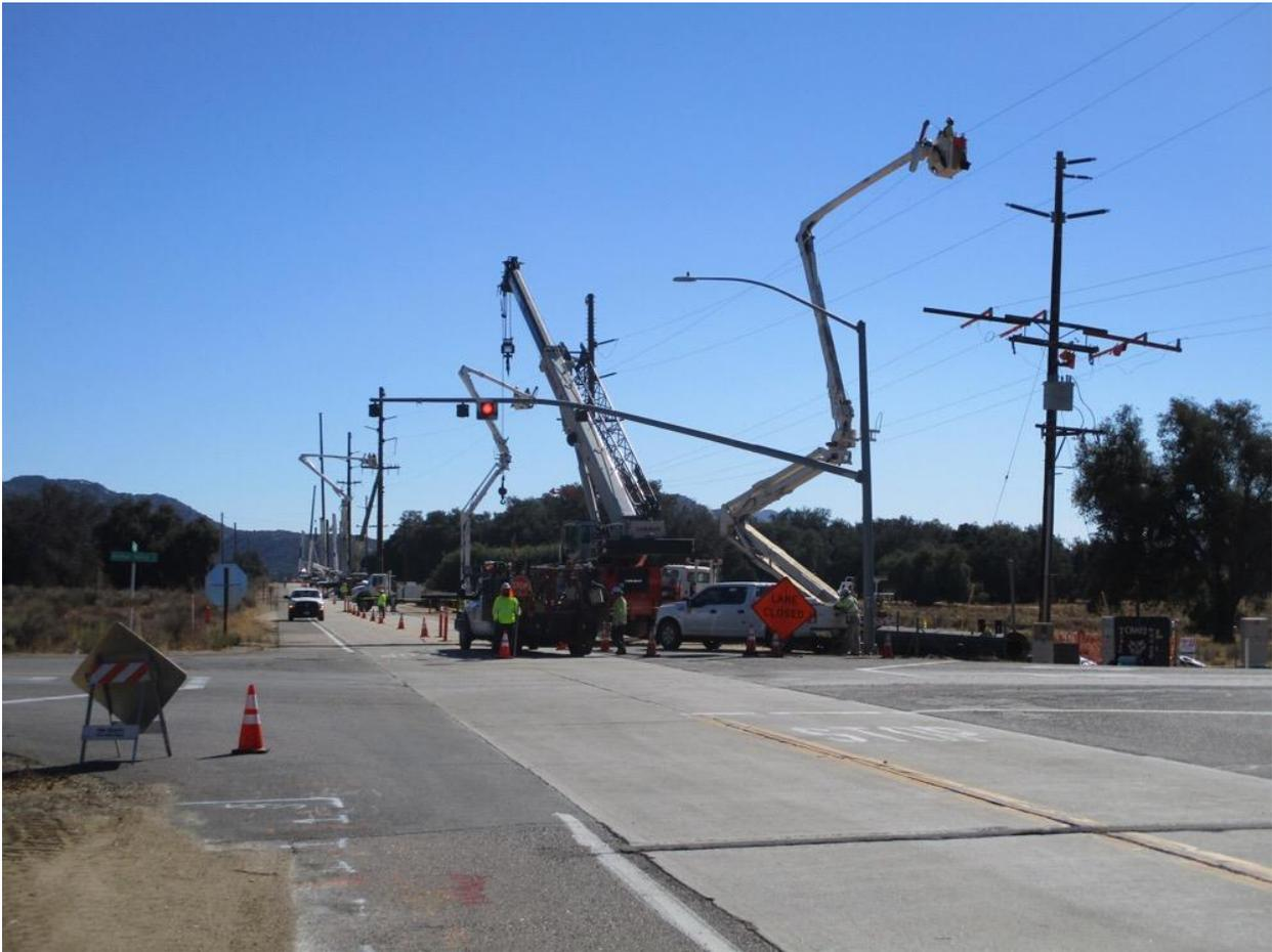
**Photo 6:** A construction crew observed conducting a lane closure along Old Highway 80 between Z40529 and Z100056 (TL 629C) and using a pilot car to lead motorists around construction areas in accordance with APM TRANS-02.
