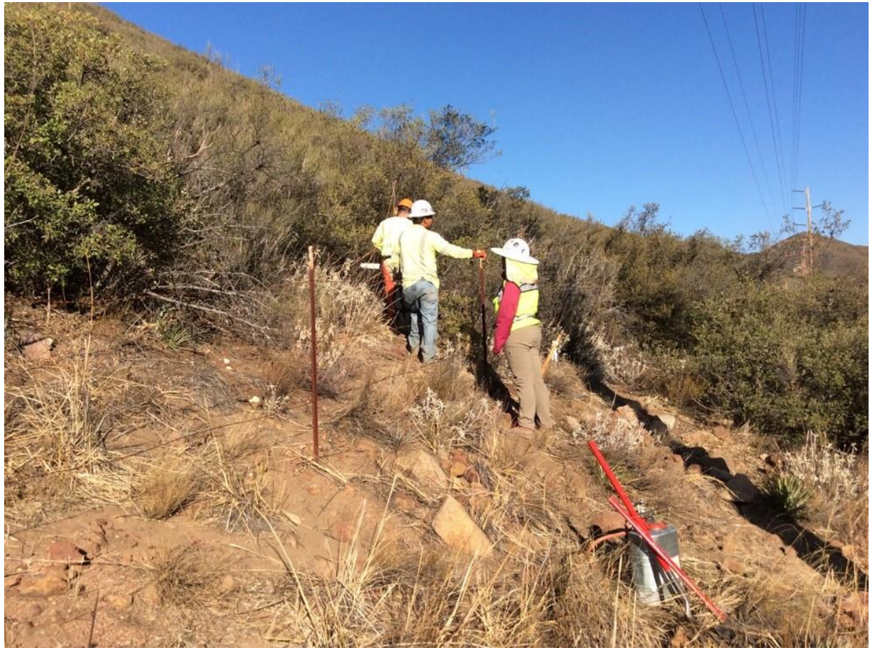
Photo 3: During vegetation removal activities to prepare the site at Pole Z40424 (TL 629C) for construction, a biological monitor was present in accordance with MM BIO-3. A complete set of fire tools was also observed within 50 feet of the activity in accordance with the CFPPP fire prevention matrix for vegetation clearing work on CNF land with a PAL of C.
