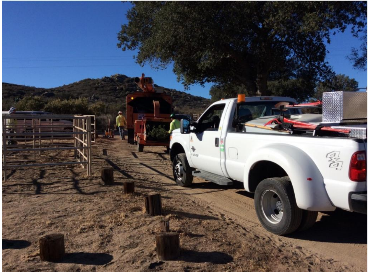
Photo 2: A Fire Patrol remained with the UTS tree trimming crew along the Access Road between Poles Z100048-Z100049 (TL 629C) to ensure the crew was equipped with at least 100 gallons of water with pump and hose during chipping, as required by the CFPPP Fire Matrix (MM FF-1) for the day's fire conditions (PAL D on CNF land).
