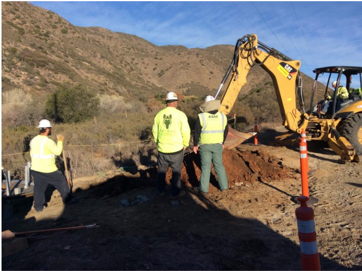
Photo 1: Archaeological and Cultural Monitors were present during ground rod trenching at Pole Z40515 (TL629C) in accordance with the HPMP, APM CUL-04, and MM CUL-1. In addition, crew members were observed adhering to ESA fencing in accordance with the HPMP and APM CUL-03.
