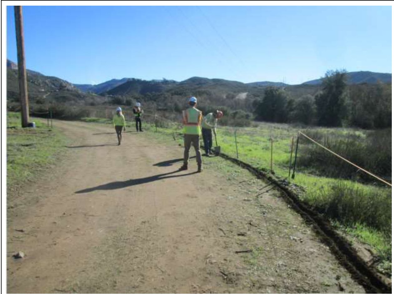
Photo 1: Archaeological monitors were observed overseeing installation of SWPPP BMPs along TL 625B adjacent to ESAs in accordance with the HPMP (MM CUL-1).
