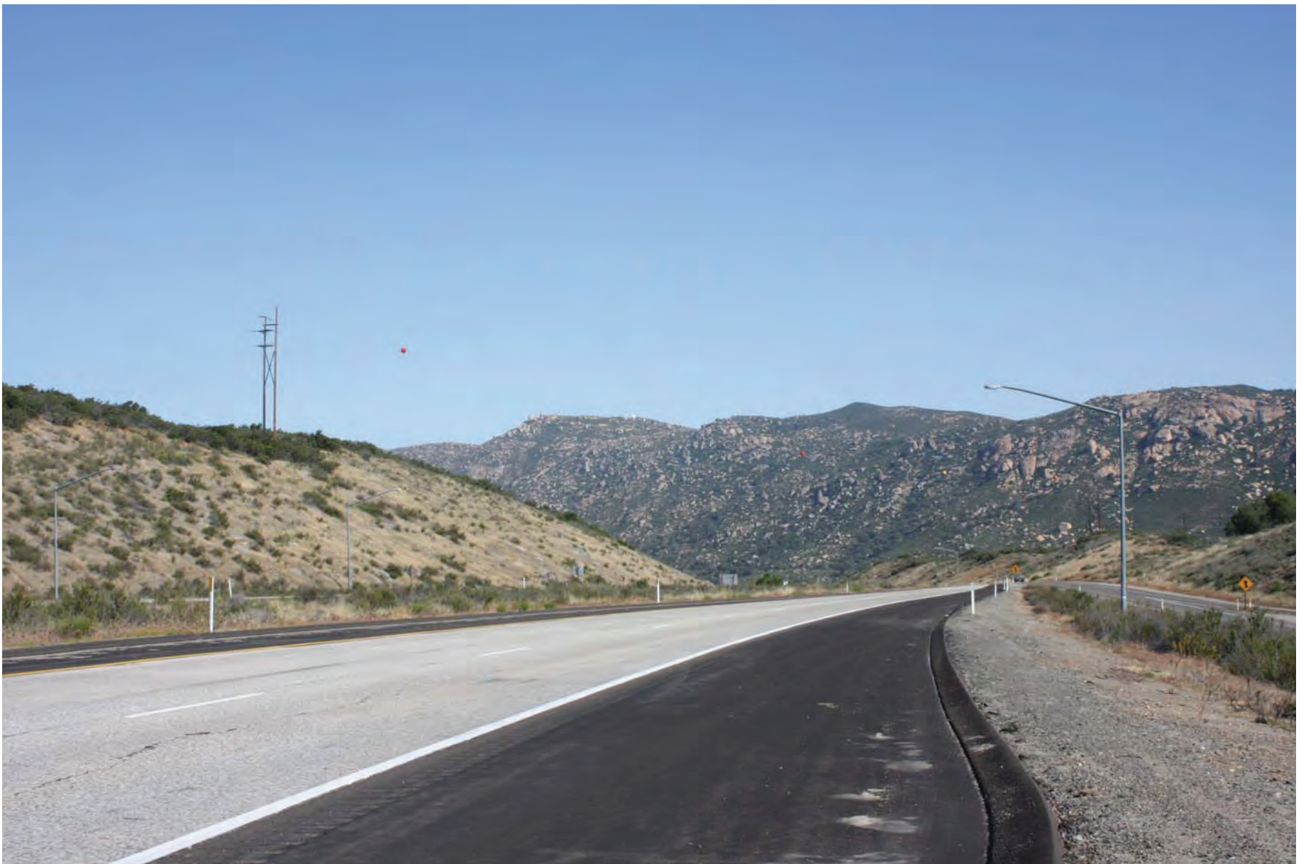
Existing view from I-8 westbound looking northwest (KVP 10)
