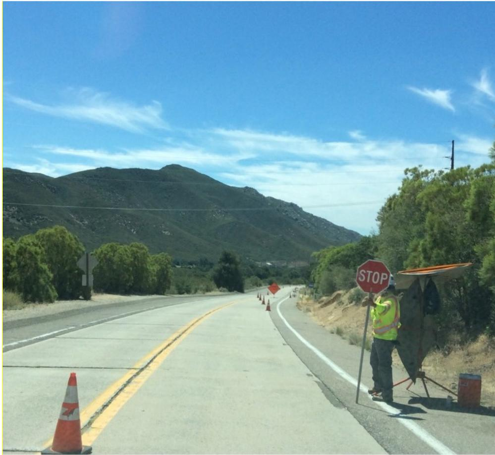
**Photo 6:** Signage, cones, flagpersons, and a clearly marked pilot vehicle were used to direct one-way traffic around the work area on Old Highway 80 (TL 629A) in accordance with the Traffic Control Plan (TCP; APM TRANS-05) and APM TRANS-02.
