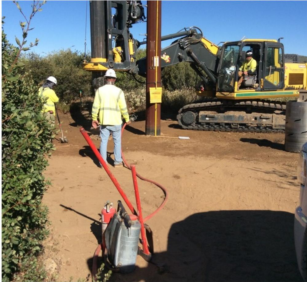
**Photo 4:** A crew was observed drilling a direct bury pole hole at P258505 (C 79B). A Dedicated Fire Patrol, at least 150 gallons of water with pump and hose, and a full set of fire tools were observed on site in accordance with the CFPPP Fire Prevention Matrix (MM FF-1) for foundation drilling on USFS land with a PAL Ev.
