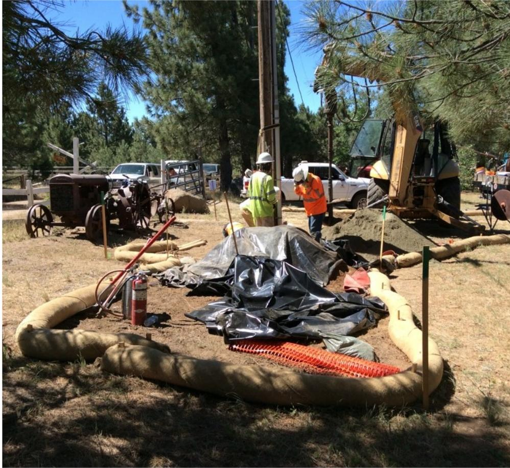
**Photo 5:** A crew was observed digging a direct bury pole hole at P45115 (C 440 Phase II). Erosion control BMPs at the site were observed in good condition in accordance with the ECP (MM HYD-1) and SWPPP (MM HYD-1, MM BIO-7).
