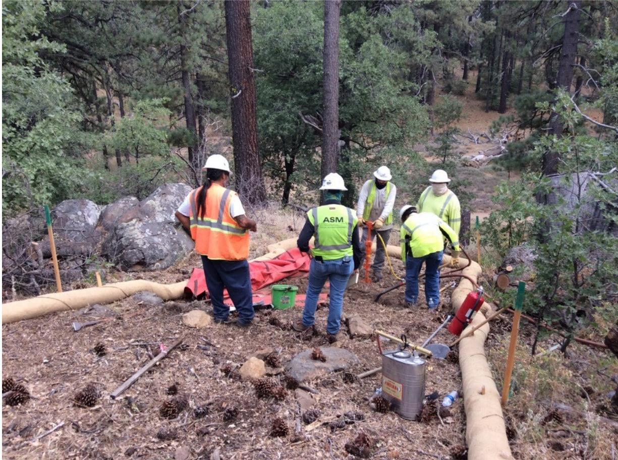
**Photo 2:** A crew was observed digging an anchor excavation on C 440 within clearly delineated work limits in accordance with MM BIO-1. Additionally, Archaeological and Cultural Monitors were present in accordance with the HPMP (MM CUL-1) and APM CUL-04.
