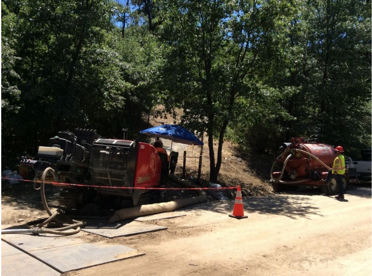
**Photo 5:** Site-specific erosion control BMPs were used under the directional drill on Los Huecos Road (C 440) to contain drill mud that may result from the activity in accordance with the SWPPP and APM HYD-09.
