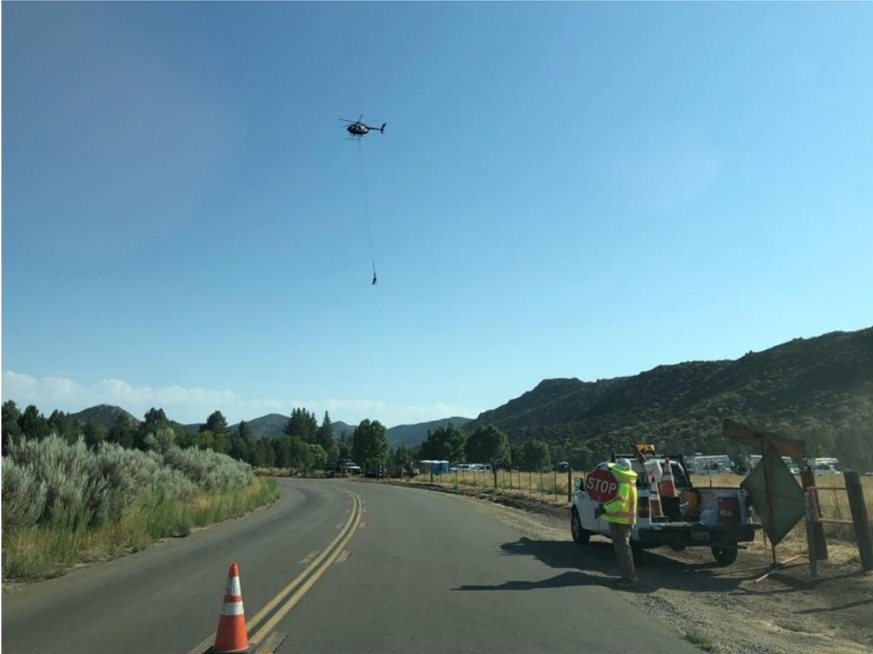
**Photo 6:** Cones, signage, and flagpersons were used to regulate traffic along Pine Creek Road (TL 629A) while helicopter external load operations in accordance with the Traffic Control Plan (APM TRANS-05), APM TRANS-02, and the Aviation Safety Plan.
