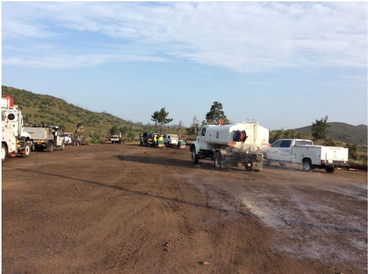
**Photo 1:** A water tender was observed applying water to the surface at Shrine Camp Staging Yard (C 440) before and during helicopter activities to minimize dust emissions from rotor wash in accordance with APM AIR-02 and the Aviation Safety Plan (MM PHS-5).
