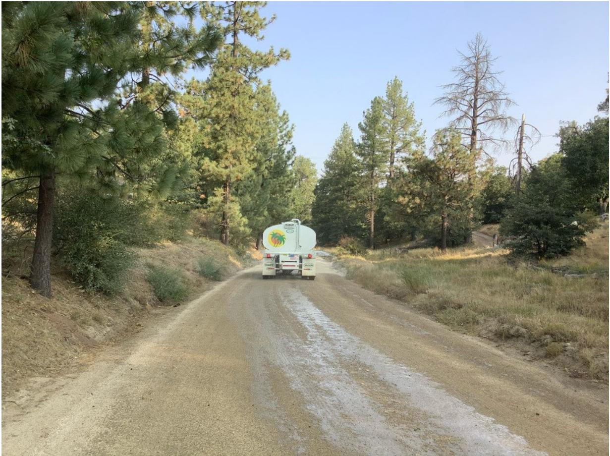
**Photo 1:** A water tender was observed applying water to the surface on Los Huecos Road (C 440) to minimize dust emissions from Project vehicular traffic in accordance with APM AIR-02.
