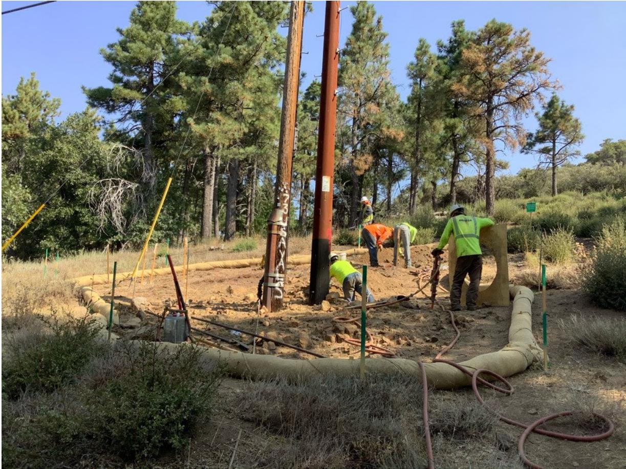
**Photo 2:** A crew was observed digging pole and anchor excavations at Pole P40370 (C 440). Crew members and materials were observed remaining within clearly delineated work limits in accordance with MM BIO-1.
