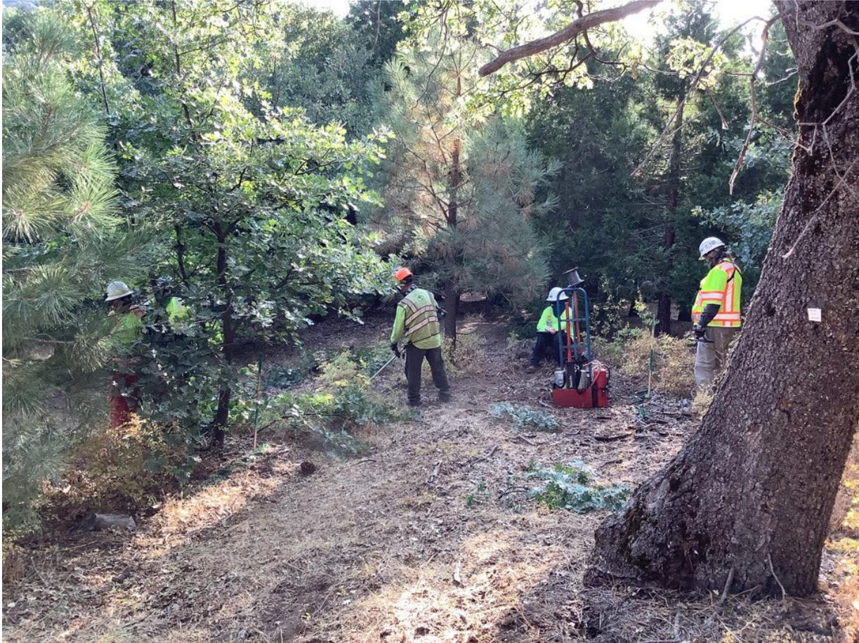
**Photo 3:** A Biological Monitor was observed monitoring vegetation removal at Pole P260424 (C 440) in accordance with MM BIO-3. In addition, the crew was observed using only battery-operated tools, a full set of fire tools was observed within 50 feet of the activity, and a Dedicated Fire Patrol was present in accordance with the CFPPP Fire Prevention Matrix for vegetation removal on USFS land with a PAL Ev (MM FF-1).
