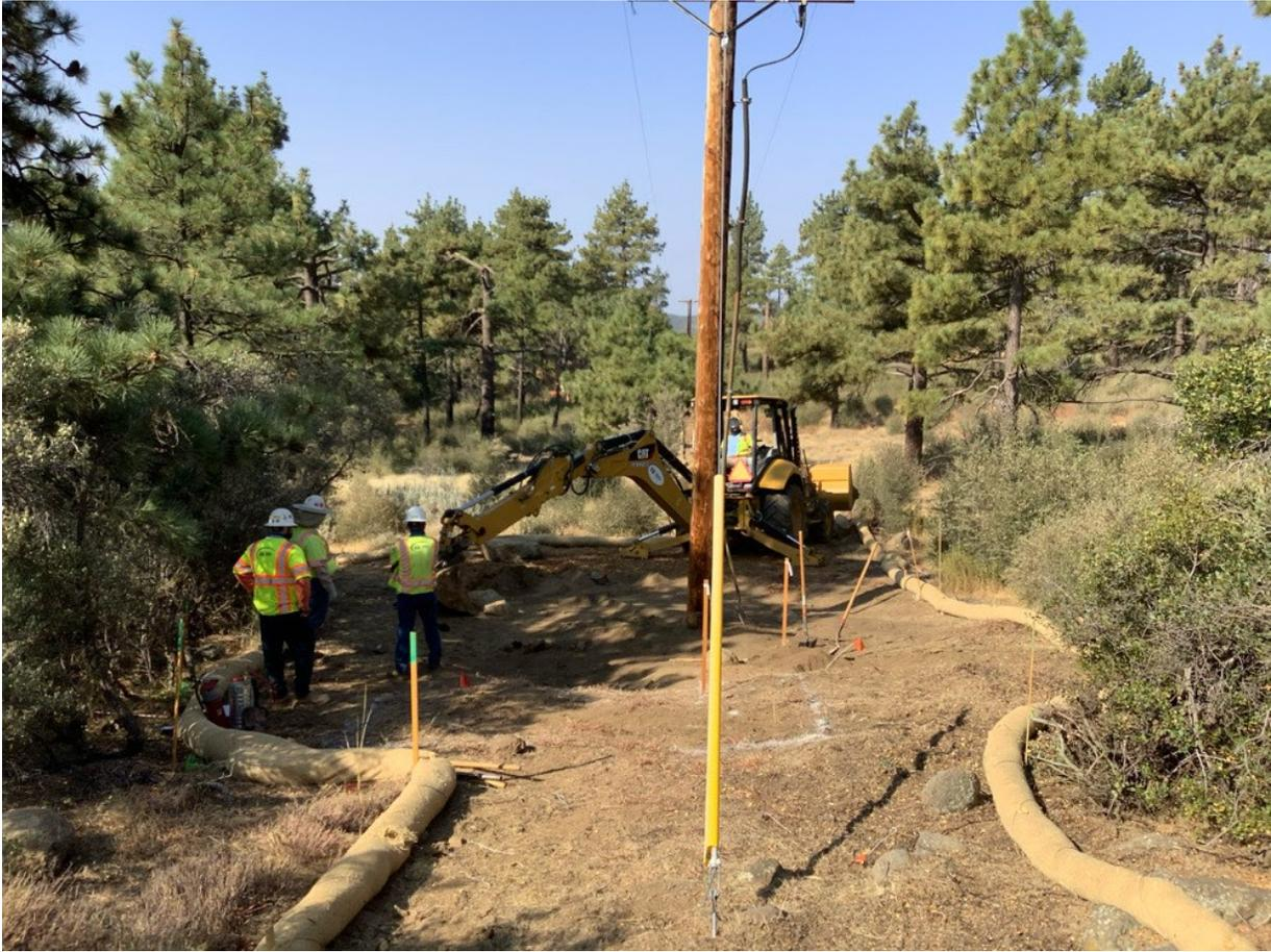
**Photo 6:** A crew was observed excavating a trench for a retaining wall near Pole P40143 (C 440). Site-specific erosion control BMPs were observed in good condition in accordance with the ECP, SWPPP (MM HYD-1 and MM BIO-7), and APM HYD-09.
