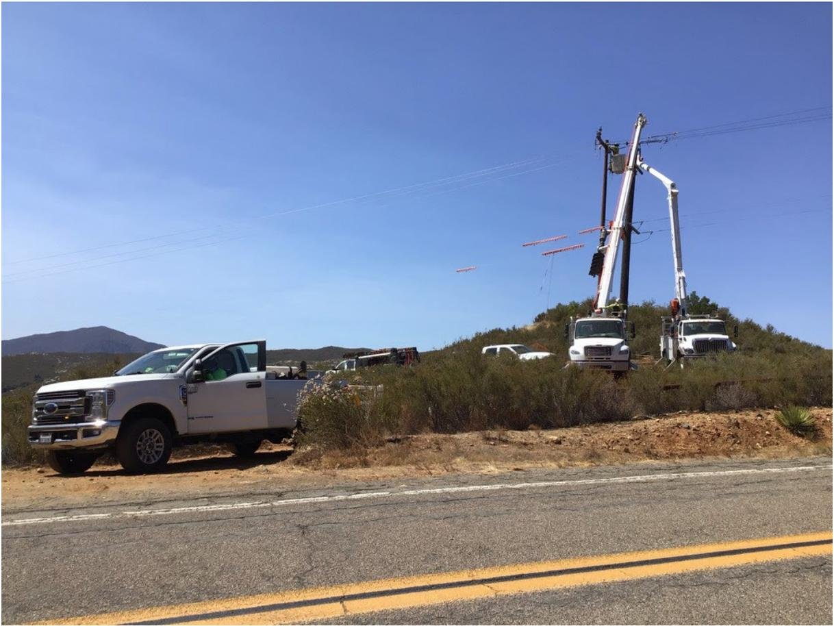
**Photo 4:** During overhead line work at Pole P258522 (C 79B), a Dedicated Fire Patrol was present and equipped with at least 150 gallons of water with pump and hose in accordance with the CFPPP Fire Prevention Matrix for conductor work with de-energized lines on USFS land with a PAL Ev.
