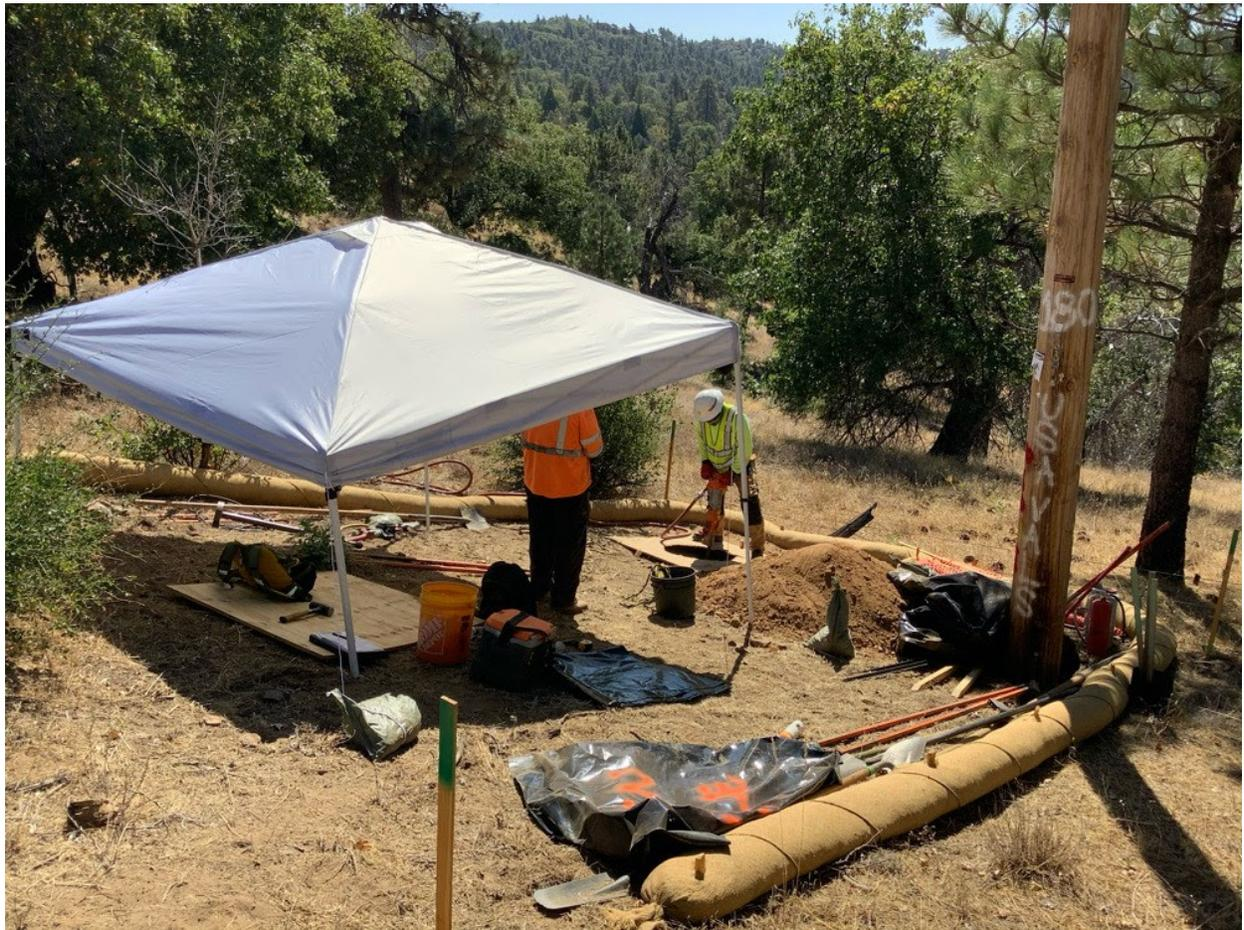
**Photo 1:** A crew was observed digging a direct bury pole hole at Pole P40320 (C 440) within clearly delineated work limits in accordance with MM BIO-1.
