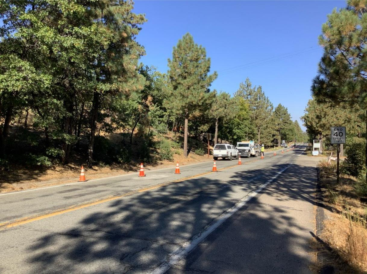
**Photo 6:** Cones, signage, and flagpersons were used to direct one-way traffic on Sunrise Highway around the work area (C 440) in accordance with the Traffic Control Plan and APM TRANS-02.
