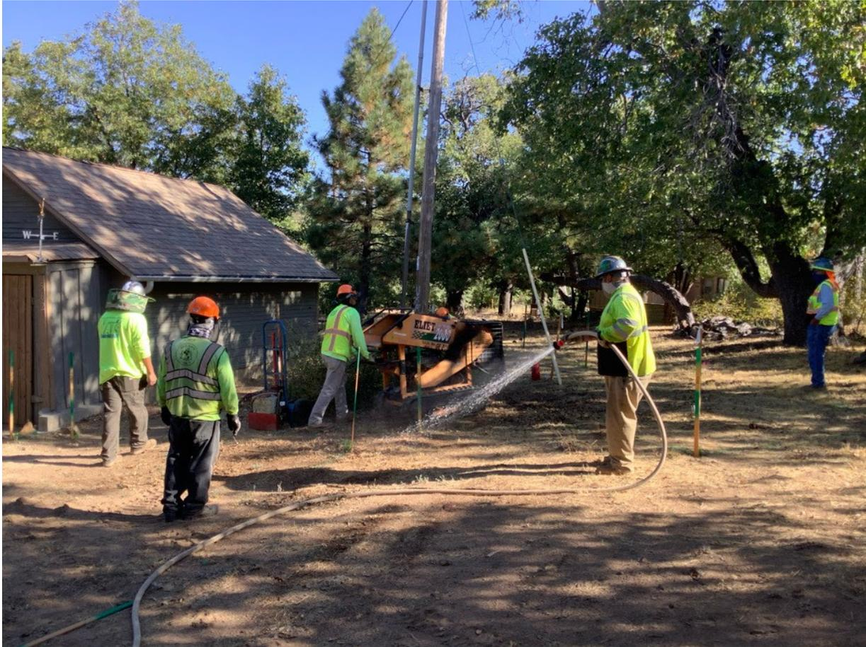
**Photo 3:** A crew was observed chipping vegetation at Pole P40208 (C 440). A full set of fire tools was observed within 50 feet of the activity, at least 150 gallons of water was observed on site, and a Dedicated Fire Patrol was observed wetting down the area in accordance with the CFPPP Fire Prevention Matrix for chipping on USFS land with a PAL Ev.
