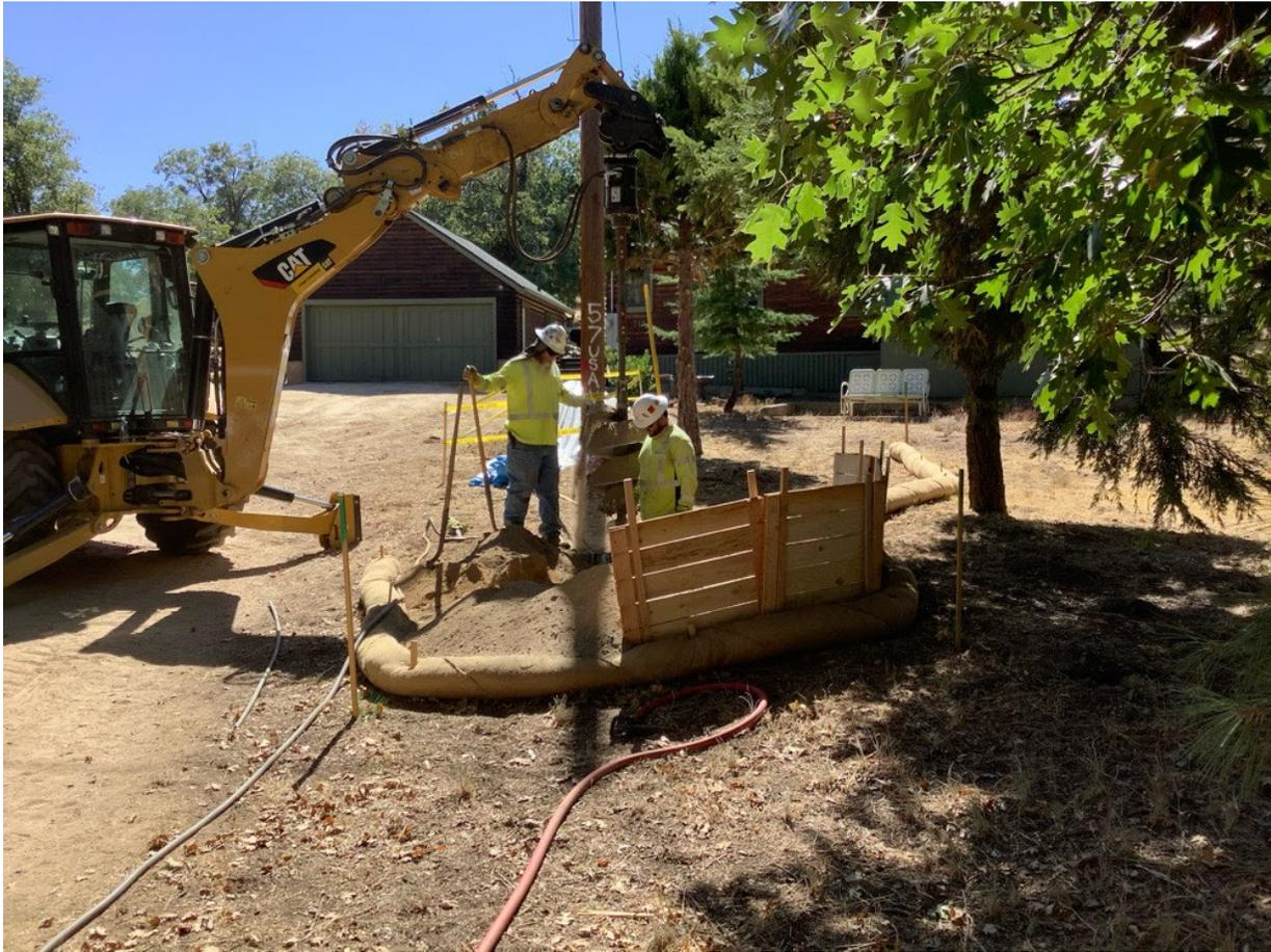
**Photo 5:** Site-specific sediment control BMPs were observed during anchor excavation at Pole P40383 (C 440) in accordance with the ECP and SWPPP (MM HYD-1), and APM HYD-09.
