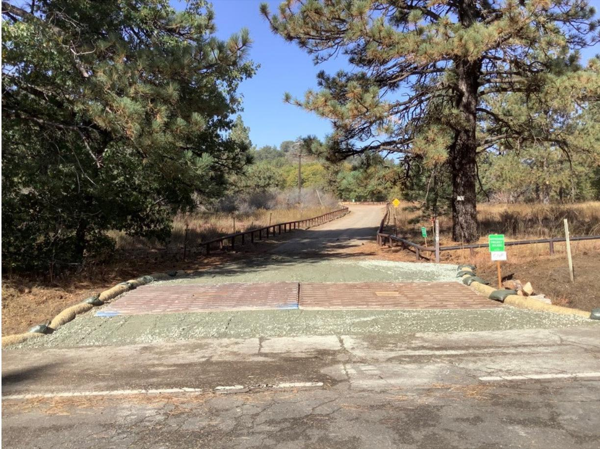
**Photo 5:** The entrance to Escondido Ravine Road (C 440) was stabilized with gravel and rattle plates to prevent trackout in accordance with the SWPPP.
