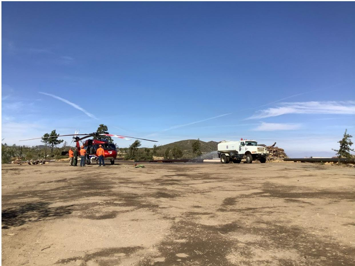
**Photo 1:** A water tender was observed applying water at Shrine Camp Staging Yard (C 440) prior to helicopter operations to minimize dust emissions from rotor wash in accordance with APM AIR-02 and the Aviation Safety Plan (MM PHS-5).
