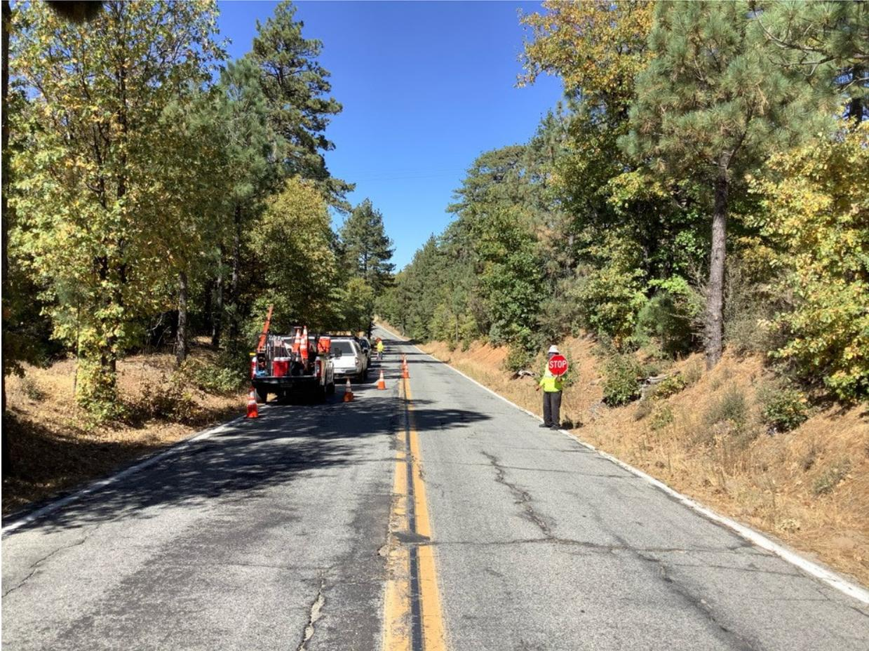
**Photo 6:** Cones, signage, and flagpersons were used to direct one-way traffic on Sunrise Highway during construction activities at Pole P40476 (C 440) in accordance with APM TRANS-02.
