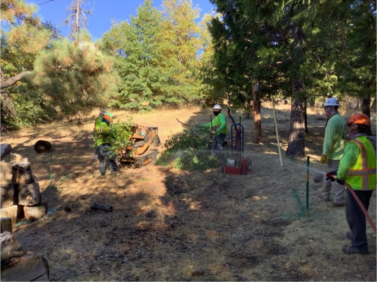
**Photo 4:** During chipping at Pole P40213 (C 440), a full set of fire tools was observed within 50 feet of the activity, at least 100 gallons of water with pump and hose were observed on site, and the area was wet down to prevent ignitions in accordance with the CFPPP for chipping on NFS land with a PAL D.
