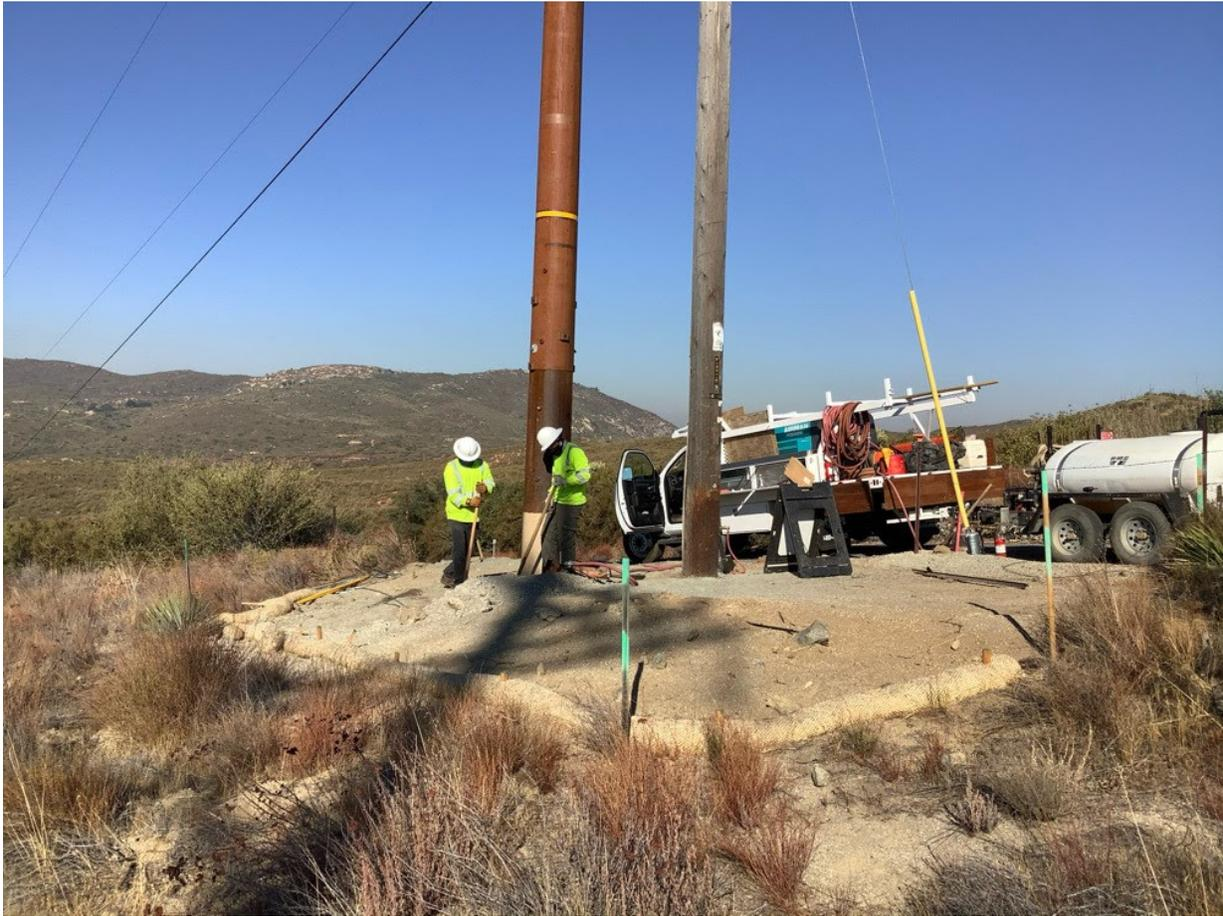
**Photo 2:** A crew was observed trenching for ground rod installation at Pole P198439 (C 79B) within clearly delineated work limits in accordance with MM BIO-1.
