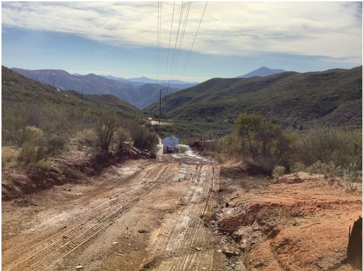
**Photo 1:** During access road maintenance along TL 6923, a water tender was observed applying water to the road to minimize dust emissions in accordance with APM AIR-02.
