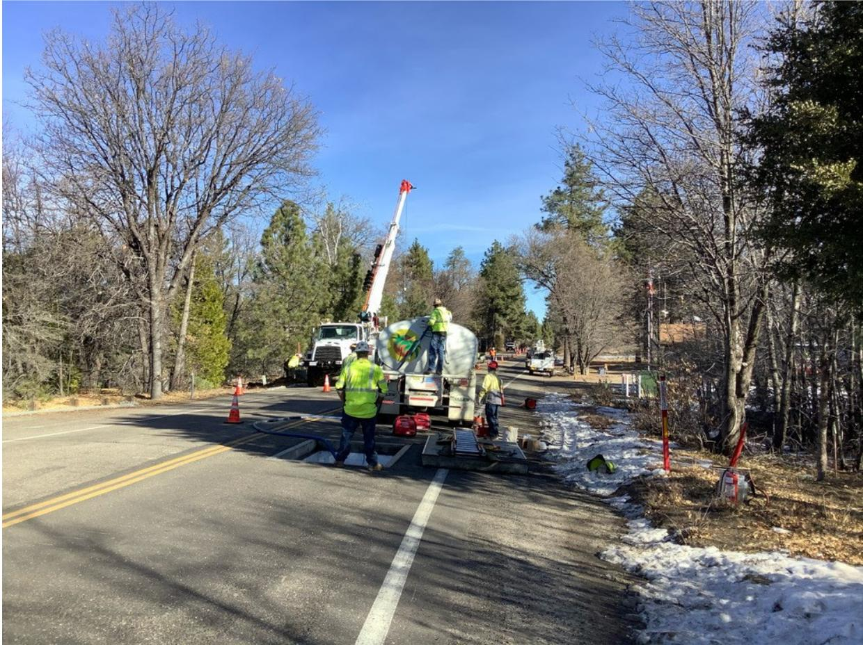
**Photo 6:** During dewatering activities on C 440, groundwater was pumped into a truck-mounted storage tank and transported to an authorized discharge location in accordance with APM HYD-08.
