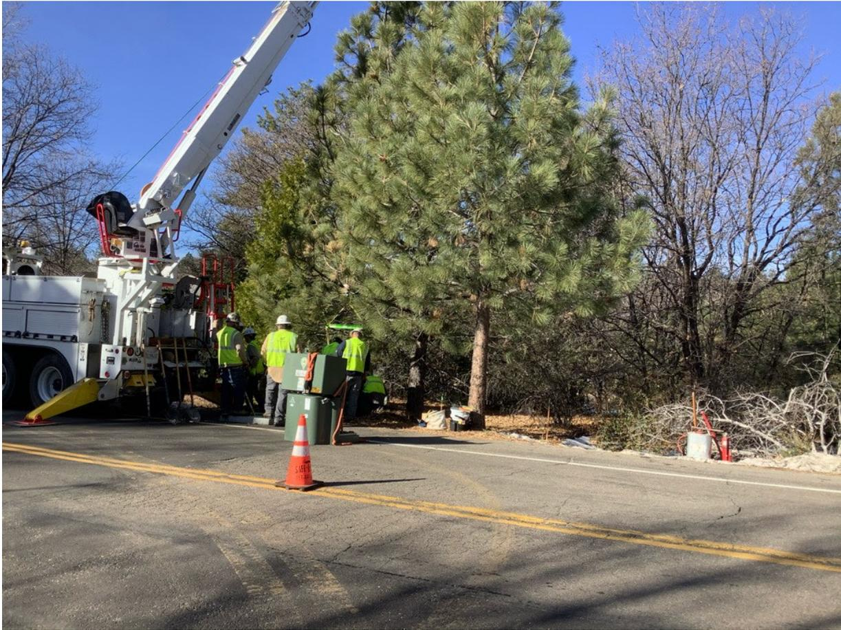
**Photo 5:** A full set of fire tools was observed within 50 feet of transformer replacement on C 440 in accordance with the CFPPP.
