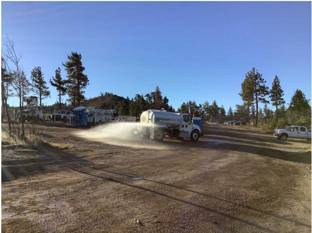
**Photo 1:** A water tender was observed applying water to the surface at Shrine Camp Staging Yard (C 440) throughout the day to minimize dust emissions in accordance with APM AIR-02.
