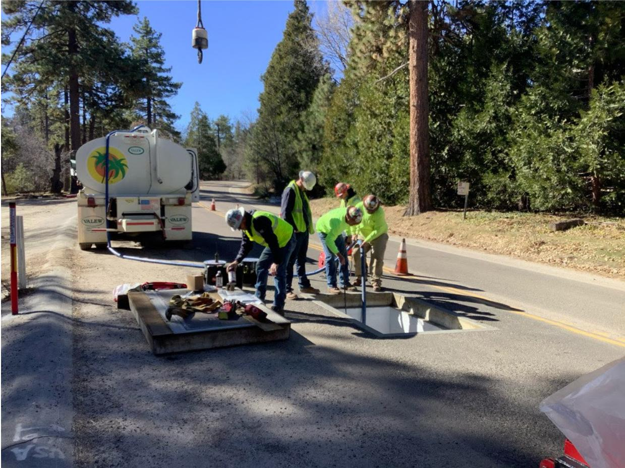
**Photo 6:** During dewatering at a hand hole along Sunrise Highway (C 440), water was pumped into a truck-mounted storage tank for dispersal in accordance with APM HYD-08.
