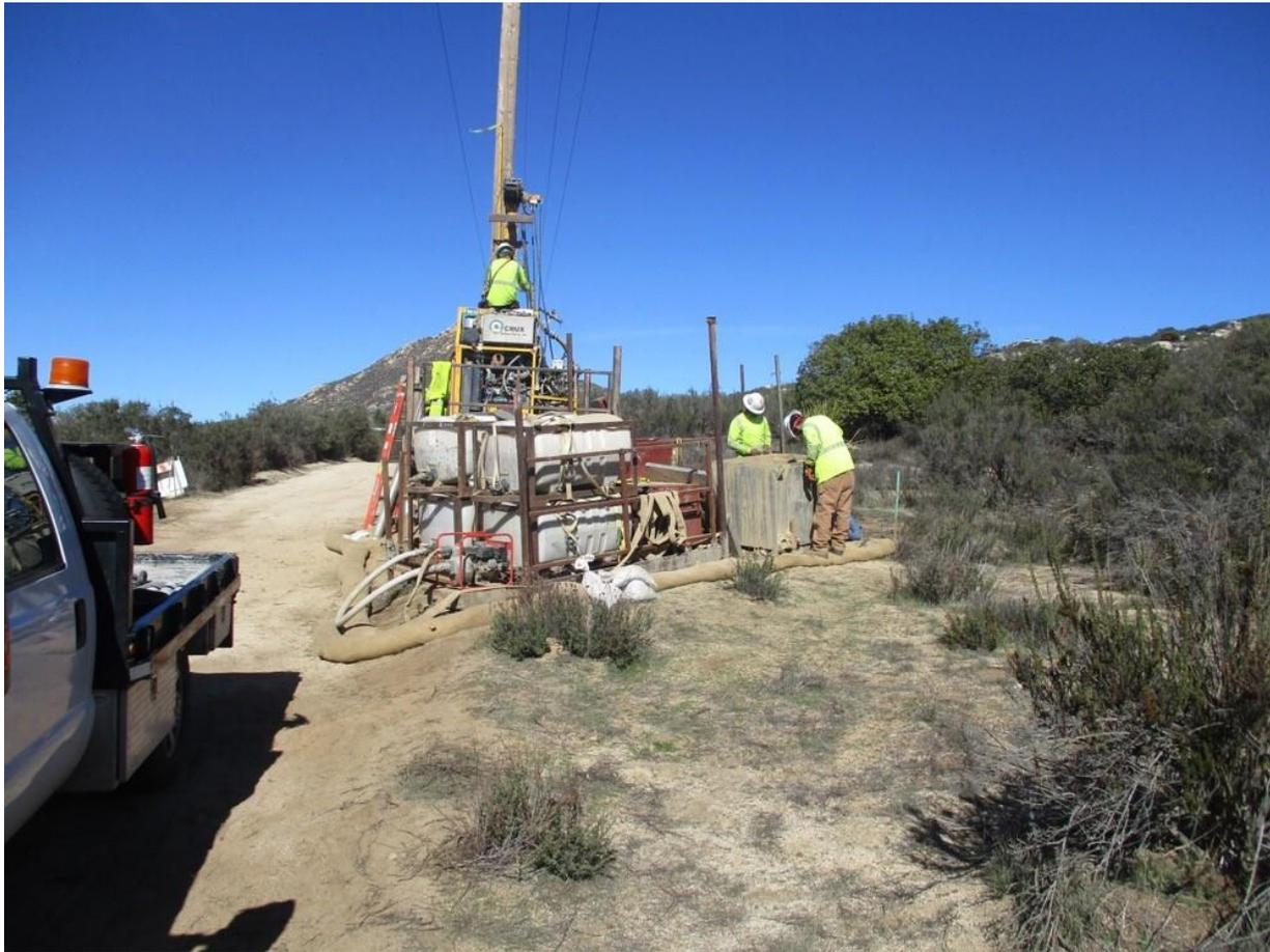
**Photo 5:** During micropile foundation hole drilling at Pole Z41007, the construction crew was observed cleaning out the cuttings containment box, which is used to trap drill cuttings and control dust emissions in accordance with APM AIR-05.
