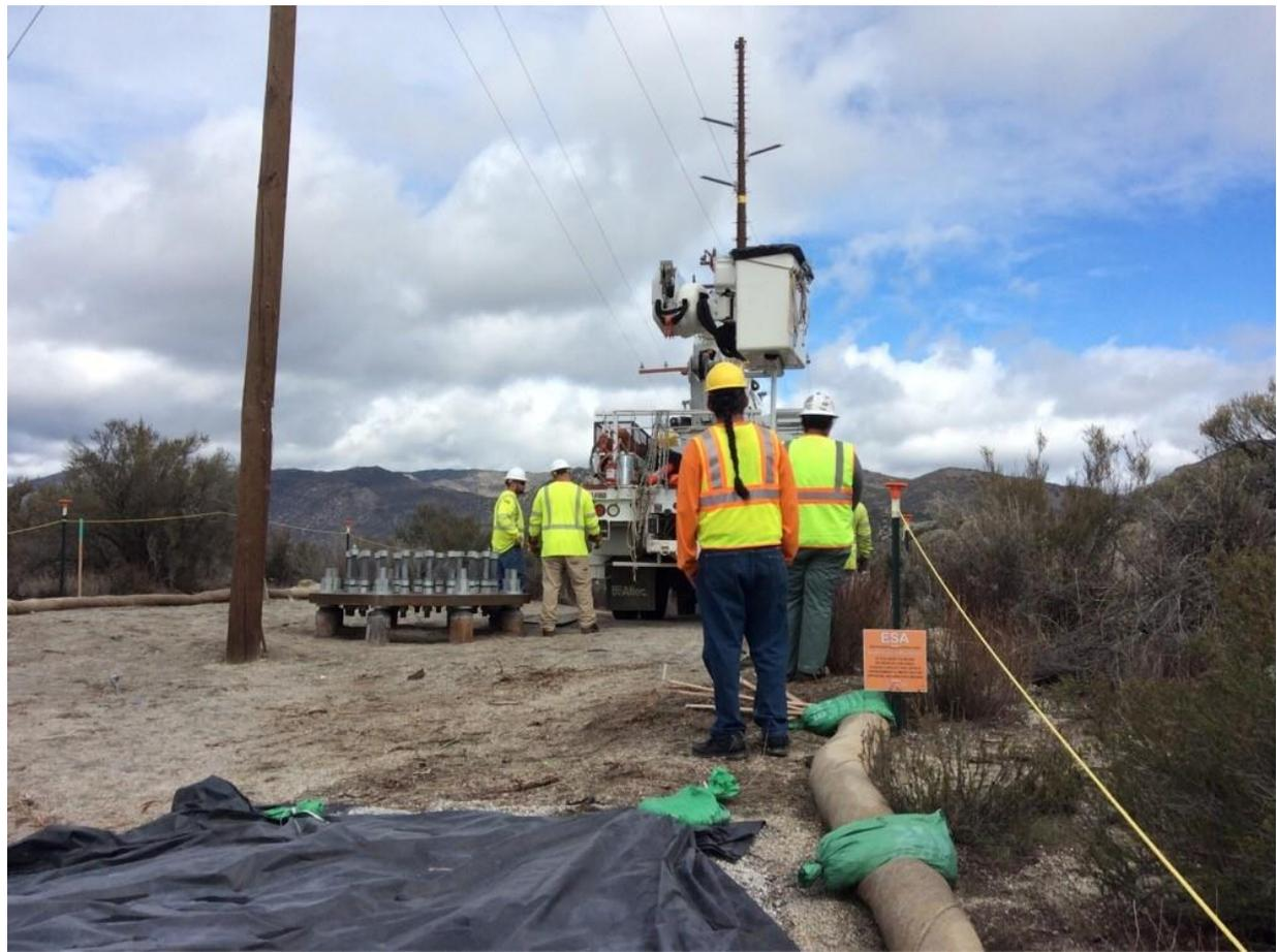
**Photo 1:** A construction crew observed setting up a bucket truck in order to spread wire at Pole Z100051 (TL 629C). Archeological and Native American monitors were on-site monitoring the activity, and ensuring that no disturbance occurred to an adjacent cultural ESA in accordance with the HPMP, MM CUL-1, and APM CUL-04.
