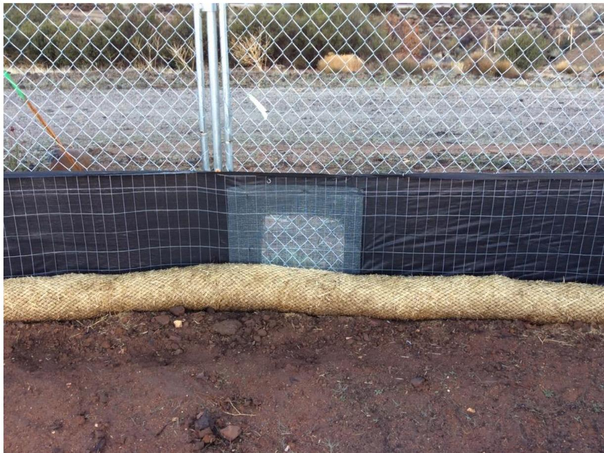
**Photo 5:** The Arroyo Toad Authorized Biologist approved screened cut-outs along the down-slope sections of the arroyo toad fencing at the Buckman Springs Fly Yard to allow water flow-through and maintain protections for arroyo toad.
