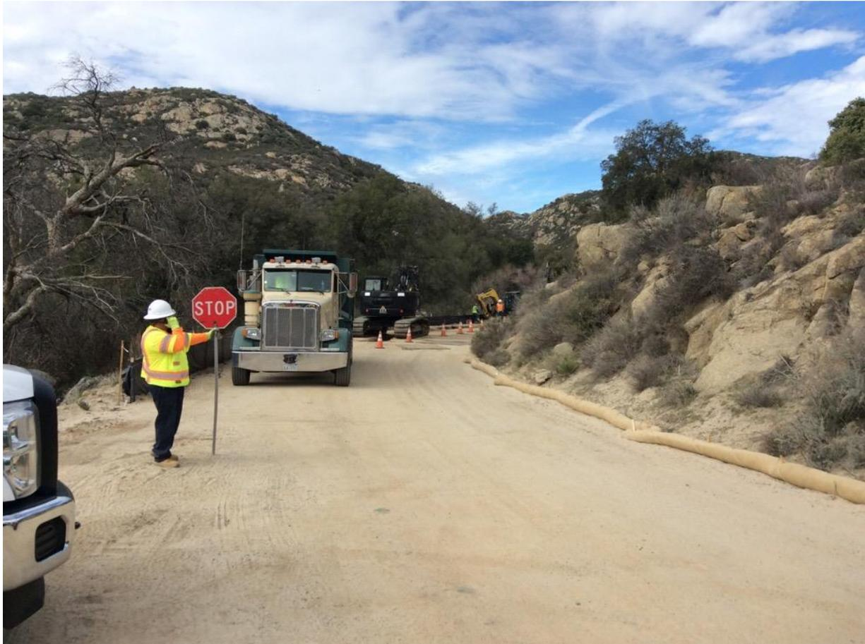
**Photo 3:** A construction crew was observed trenching for the underground distribution line along Morena Stokes Road (C 449). Traffic was regulated along the road to maintain a safe travel lane for motorists in accordance with APM TRANS-02.
