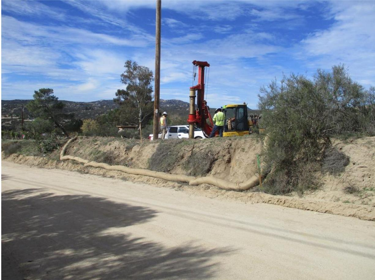
**Photo 2:** A construction crew observed drilling direct bury pole hole at Z40999 (TL 6958). Fiber rolls used for erosion and sediment control were observed to be in good condition, in accordance with the Erosion Control Plan and SWPPP.
