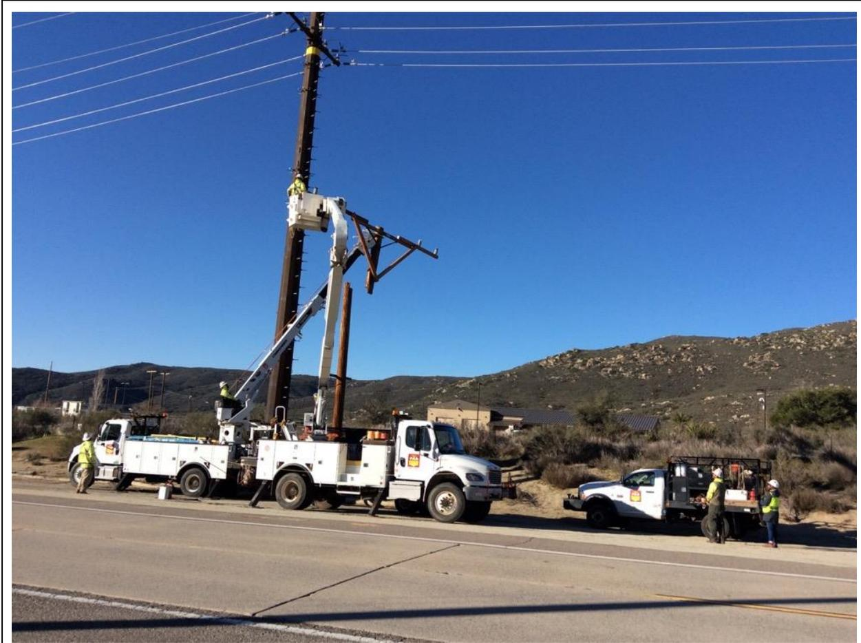
**Photo 1:** A construction crew observed removing the old wooden pole at Z40525 (TL 629C).
