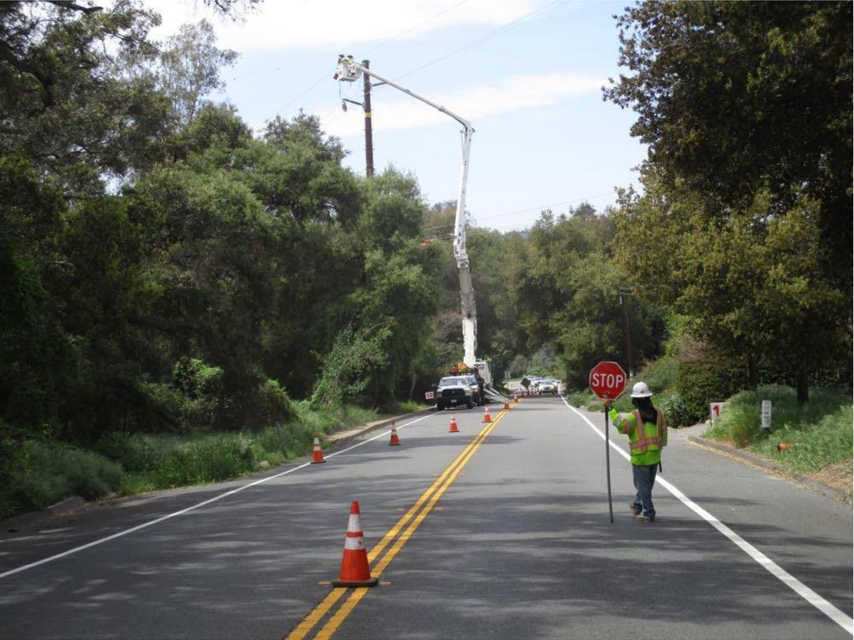
**Photo 6:** During 69 kV wire clipping at Z115713 (TL 682), traffic personnel directed one way traffic around staged equipment along Highway 76 in accordance with APM TRANS-02.
