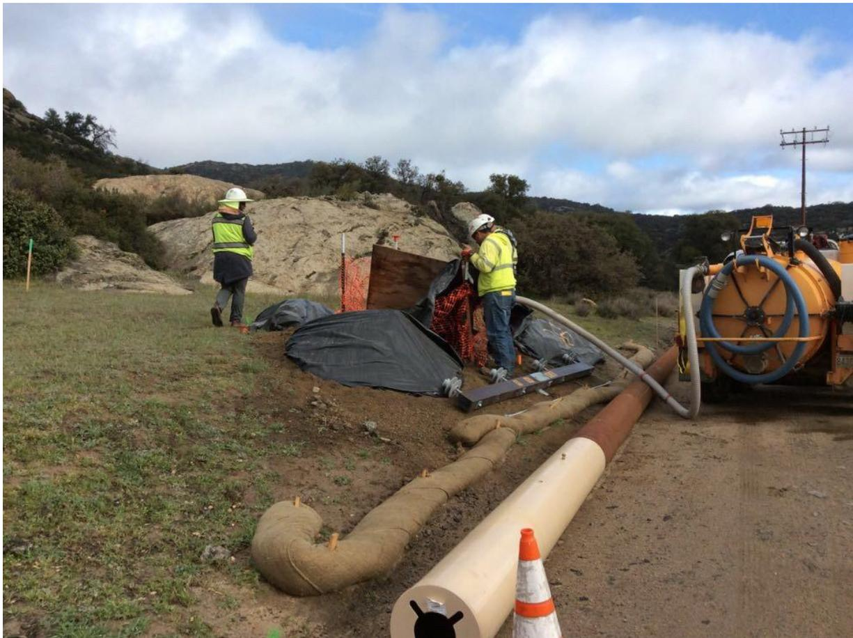
**Photo 3:** A construction crew was observed pumping groundwater out of the pole excavation at P258869 (C 449) prior to pole setting. A Biological Monitor was present in accordance with MM BIO-22 and the spoils stockpile was observed to be securely covered in accordance with the Erosion Control Plan and SWPPP. The water was transported in the vacuum machine to Buckman Springs Fly Yard, where it was dispersed for dust control in accordance with APM AIR-02.
