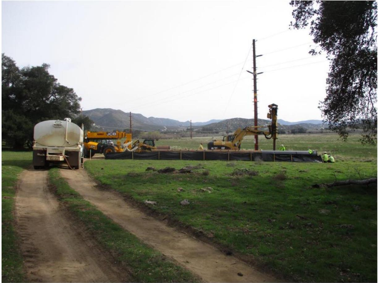
**Photo 5:** Construction crews were observed drilling for a direct bury pole hole at Z409970. Silt fence was observed in good condition in accordance with the SWPPP.
