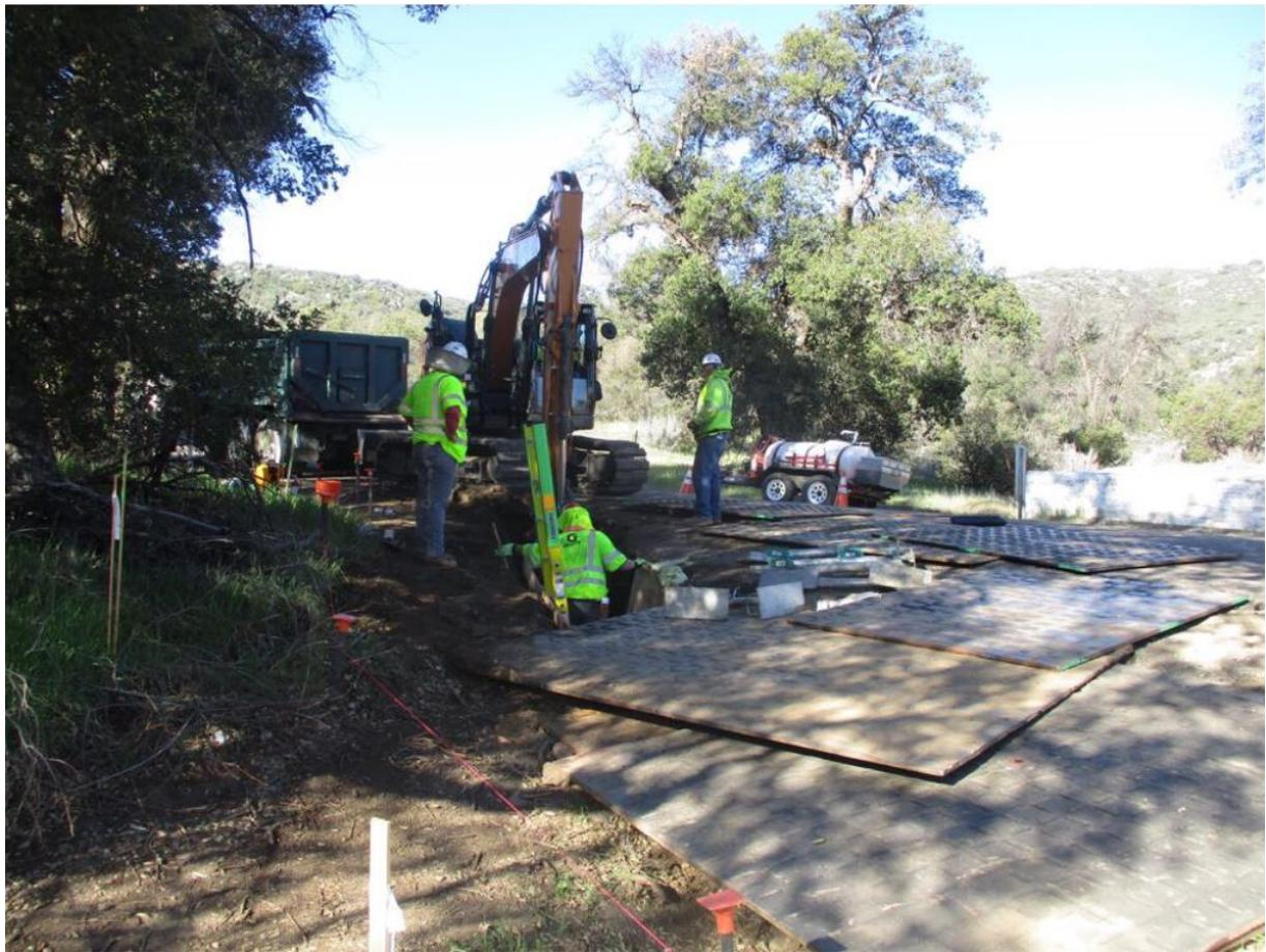
**Photo 1:** Construction crews were observed trenching for the installation of 12 kV underground line at C449. Due to the presence of a cultural resources ESA within 50 feet, an archeological and Native American monitor were observed inspecting excavated soils in accordance with the HPMP, MM CUL-1, and APM CUL-04.
