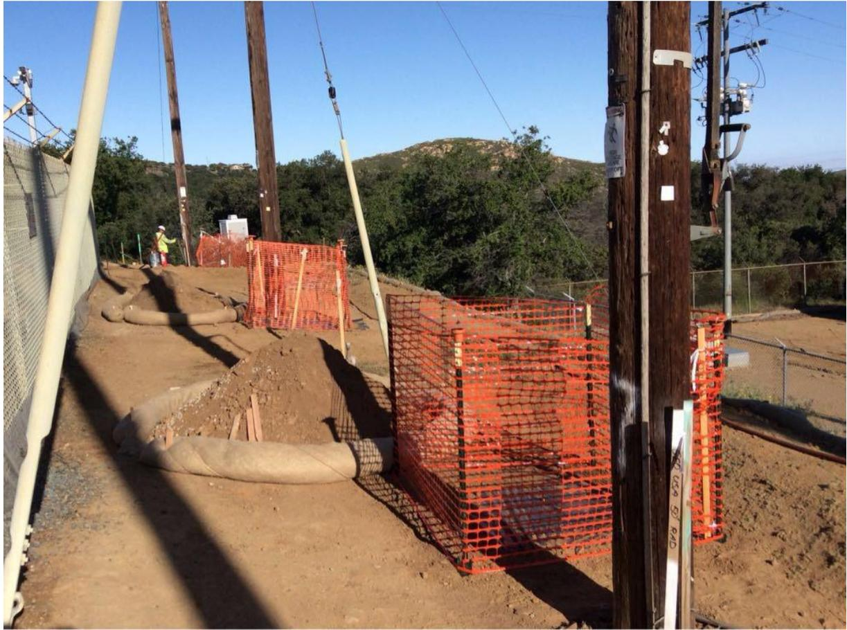
**Photo 4:** Spoils from pole excavations occurring along TL 629A were stabilized with fiber rolls in accordance with the Erosion Control Plan and SWPPP (MM HYD-1, MM BIO-7) and excavations were securely covered in accordance with MM BIO-23.
