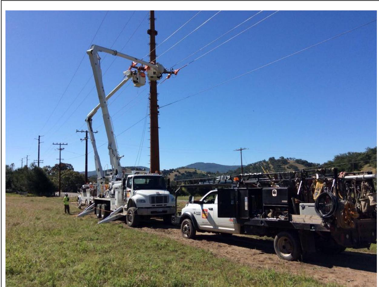
**Photo 5:** A construction crew was observed removing temporary disconnects at Pole Z128035 on TL 682. Construction work occurred within the work limits and approved access road in accordance with MM BIO-1.
