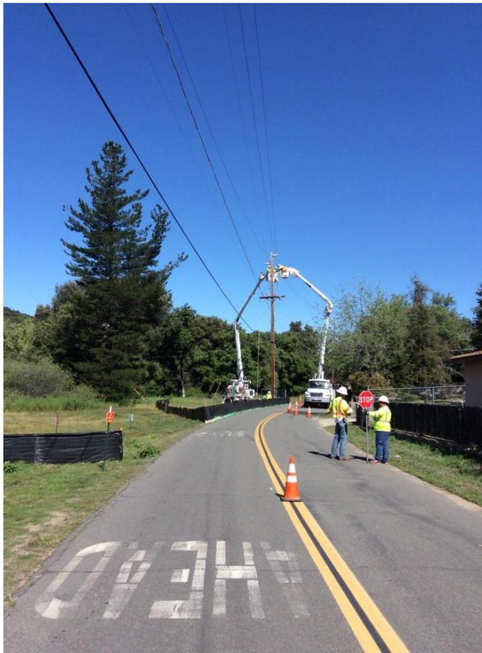
**Photo 1:** A construction crew was observed spreading wire at Pole Z172804 (TL 629A). Flagmen and signs were used to regulate traffic and maintain a safe transportation corridor in accordance APM TRANS-02. Exclusionary fencing for arroyo toad was observed to be secure and in good condition in accordance with APM BIO-3.
