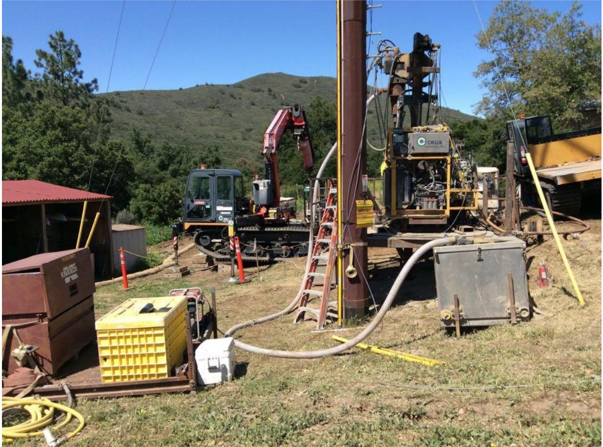
**Photo 2:** A containment box was used to trap drill cuttings during micropile drilling in order to reduce dust emissions at Z173104 (TL 629A) in accordance with APM AIR-05. Fuel for the micropile equipment was observed stored within a double-walled cell to prevent the release of hazardous materials onto the ground in accordance with MM PHS-2.
