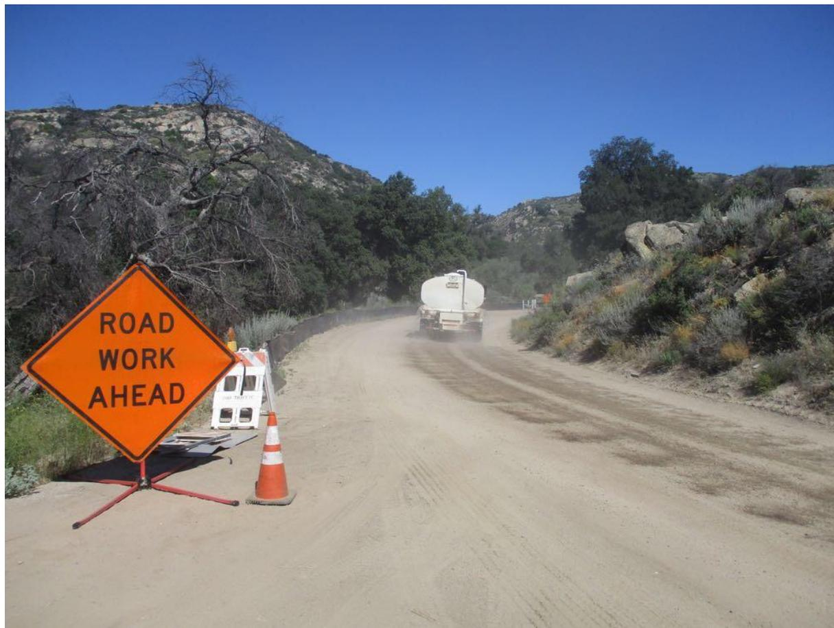
**Photo 5:** A water truck was observed being used to control fugitive dust emissions along Corral Canyon Truck Trail in accordance with APM AIR-02 and APM AIR-05. Traffic control signage was also observed along the road in accordance with the Traffic Control Plan.
