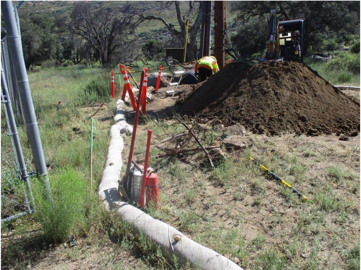
**Photo 3:** During excavation work to install intercepts at P161903 (C 449), perimeter fiber rolls were observed functional in accordance with the ECP and SWPPP. A complete set of fire tools was staged on site (5-gallon backpack pump, round point shovel, Pulaski, and 2A10BC fire extinguisher) in accordance with the CFPPP (MM FF-1).
