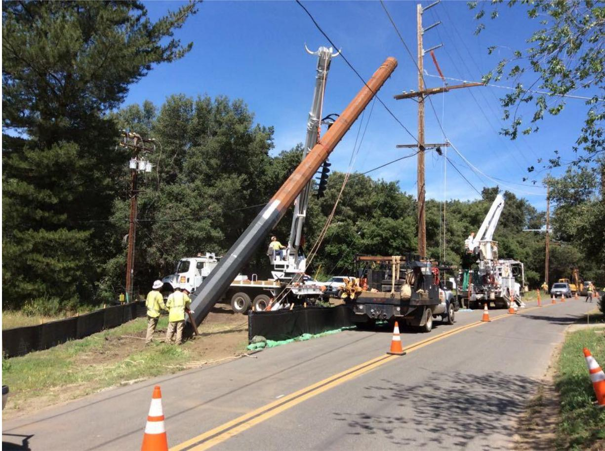
**Photo 2:** A construction crew was observed setting the pole base at Pole Z172804 (TL 629A). Cones, signage, and traffic flaggers were used to maintain a safe travel corridor for motorists in accordance with the Traffic Control Plan and APM TRANS-02. Arroyo toad exclusion fencing was observed in good condition with gravel bags in accordance with arroyo toad avoidance and minimization measures (APM BIO-03).
