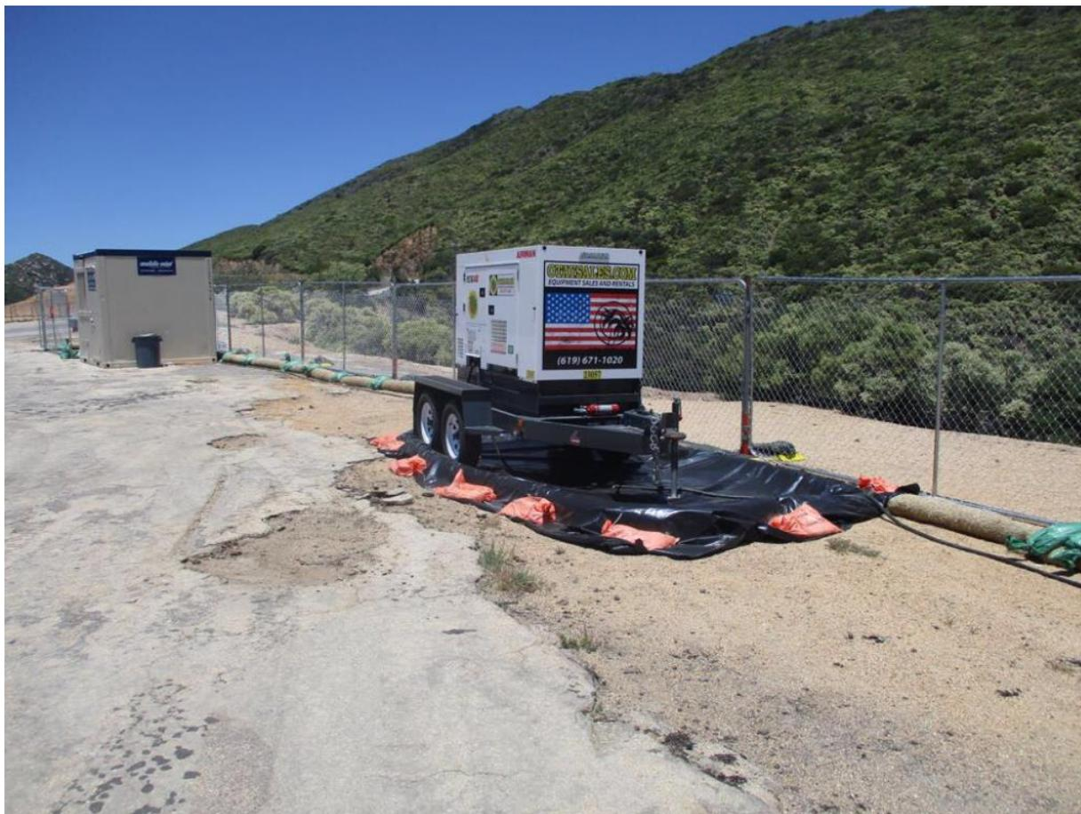
**Photo 6:** Visqueen was observed staged beneath a stationary generator at a C 440 staging yard for drip and spill protection in accordance with the SRNP and MM PHS-2.
