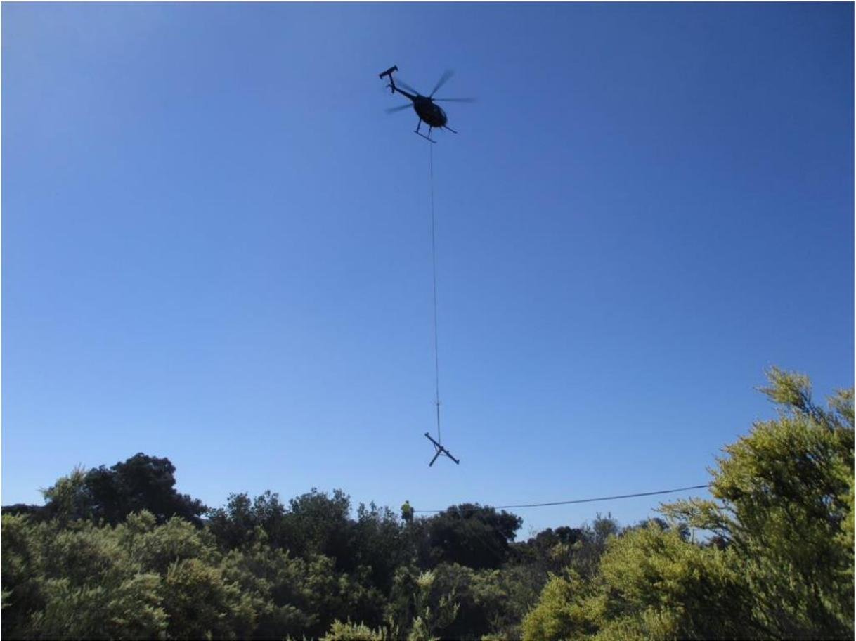
**Photo 4:** Crews were observed cutting off old wooden poles above communications lines and removing pole tops via helicopter external loads along C 449 (P45925, above).
