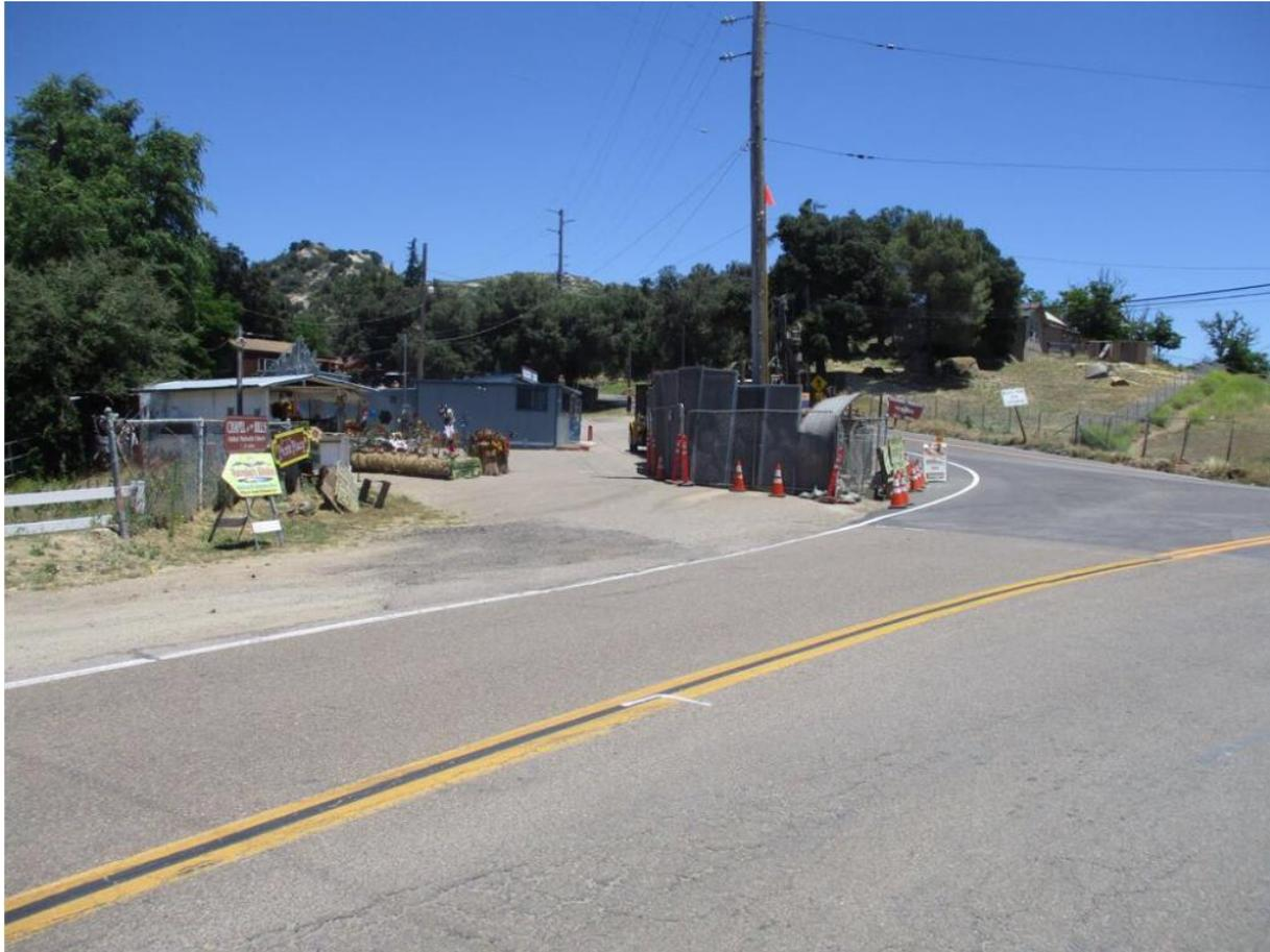
**Photo 3:** Noise barriers were observed being implemented at Z173060 (TL 629A) during micropile drilling activities to reduce noise in accordance with MM NOI-1.
