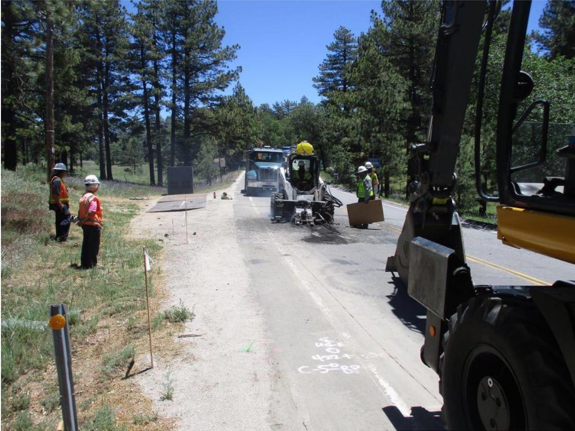
**Photo 5:** During asphalt grinding at Station 422+74 (C 440) in preparation for vault excavation and steel plate installation, water was applied at the recommendation of the SDG&E fire coordinator for fire risk mitigation in accordance with the fire prevention matrix in the CFPPP. Cultural resource monitors were present on-site for upcoming vault excavation work in accordance with the HPMP, MM CUL-1, and APM CUL-04.
