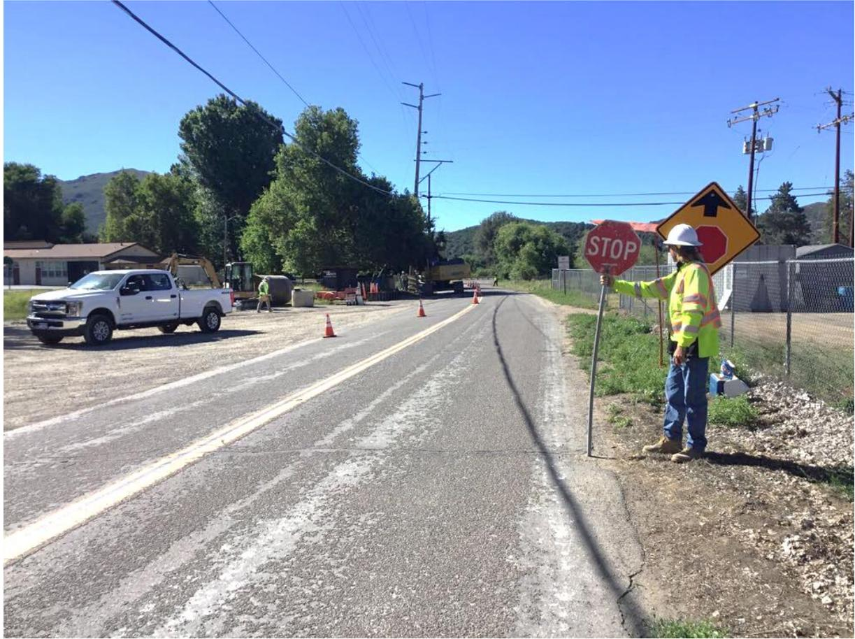
**Photo 2:** During micropile drilling operations along River Drive at Pole Z373253 (TL 629A). A traffic flagger was observed conducting a lane closure and directed one-way traffic in accordance with the TCP (APM TRANS-05) and APM TRANS-02.
