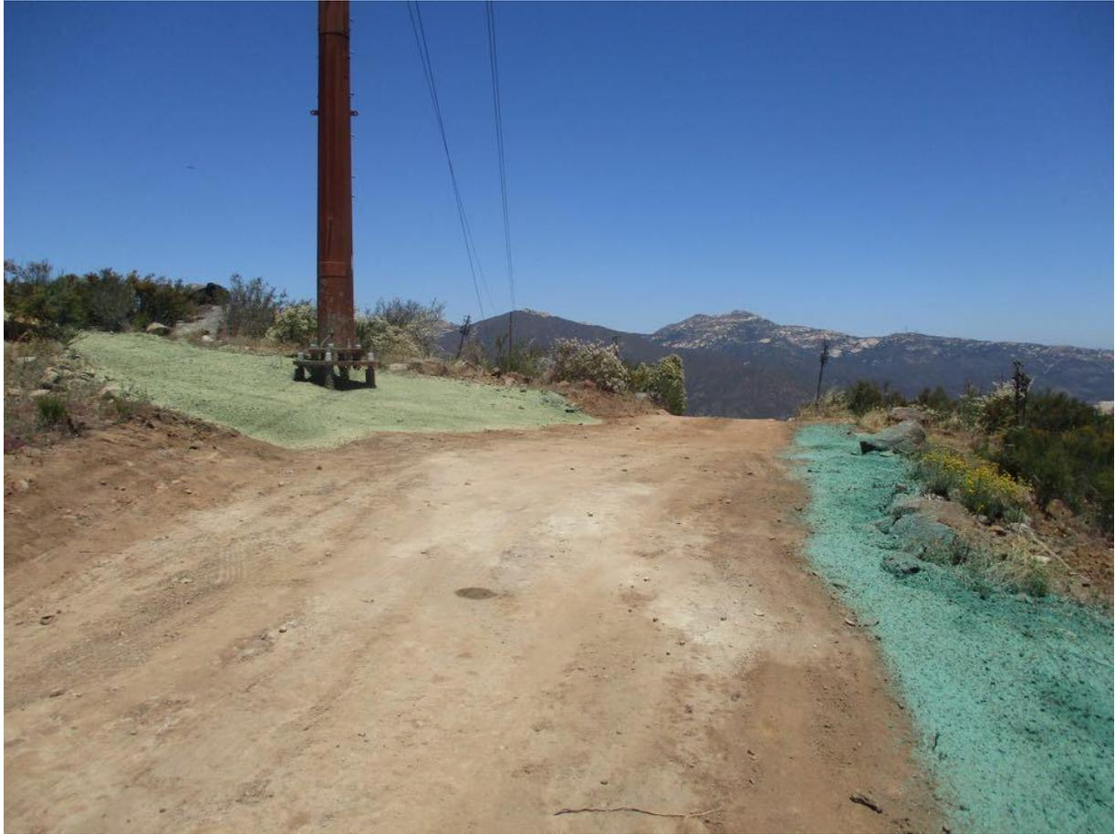
**Photo 6:** Hydraulic mulch was observed applied at completed Pole Z571463 (TL 6957) and along the access road for post-construction erosion control in accordance with the ECP, SWPPP, and HRP (MM HYD-1, MM BIO-9, MM BIO-4).
