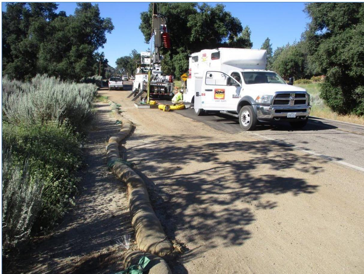
**Photo 4:** A construction crew was observed splicing 12 kV lines at a vault along C 449. Fiber rolls were observed along the work space in good condition in accordance with the ECP and SWPPP (MM HYD-1, MM BIO-7).
