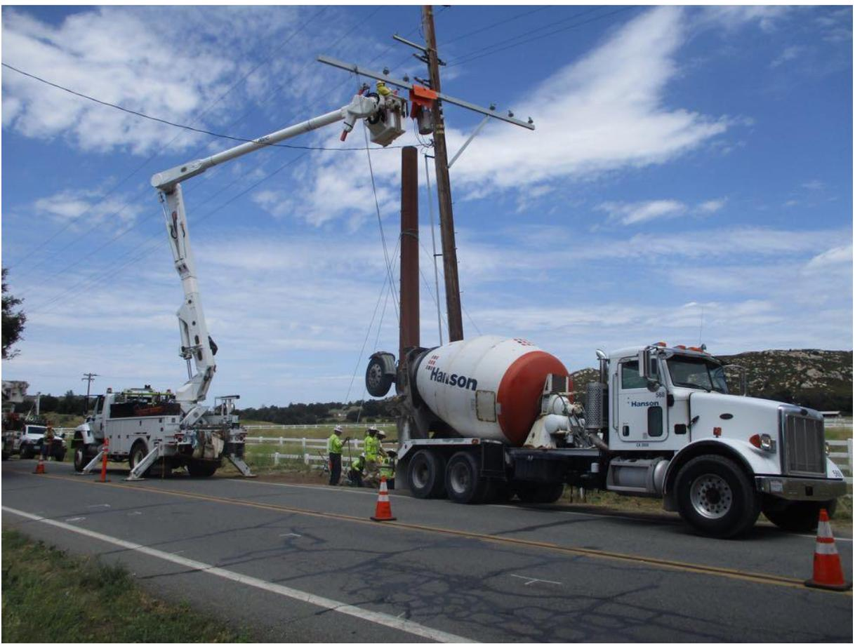
**Photo 1:** A construction crew was observed removing 12 kV wire protectors used during pole setting, and backfilling around the pole base with concrete on TL 629A. A crew member was conducting traffic control along Viejas Boulevard during the activities in accordance with the TCP (APM TRANS-05).
