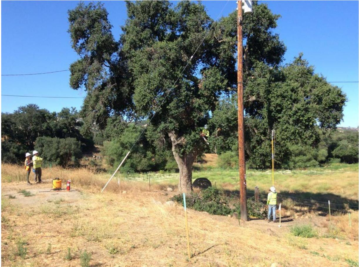
**Photo 3:** A crew member at Pole P275795 (TL 625C) was observed holding a tree pruner at a work limits stake to increase the visibility of the stake to the crew member in the tree, ensuring that tree trimming remained within approved work limits in accordance with MM BIO-1. Biological monitors were present to oversee the vegetation removal activity in accordance with MM BIO-3.
