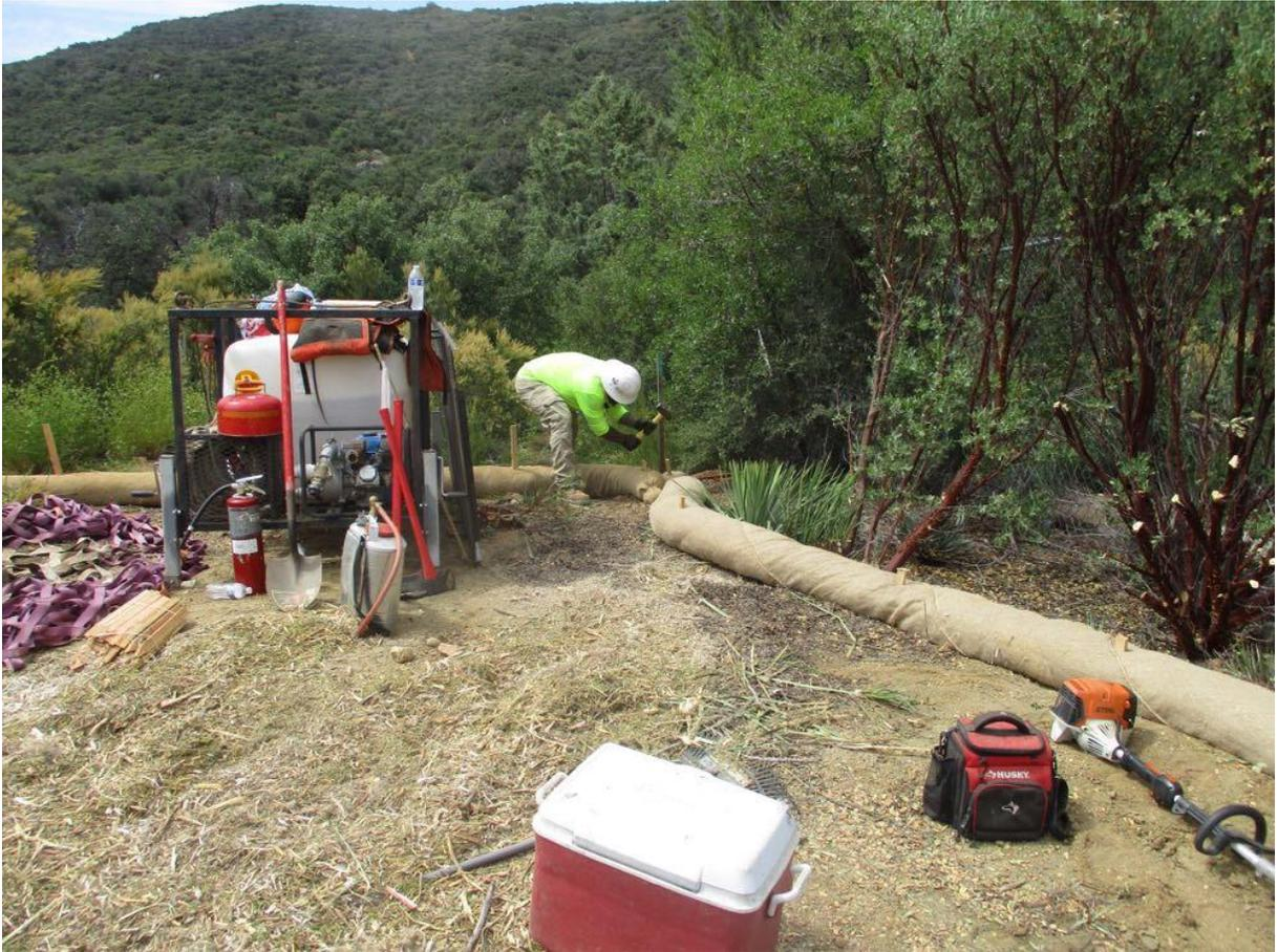
**Photo 2:** A construction worker observed installing perimeter fiber rolls at Pole Z173110 (TL 629A) for erosion control in accordance with the ECP and SWPPP (MM HYD-01, MM BIO-7).
