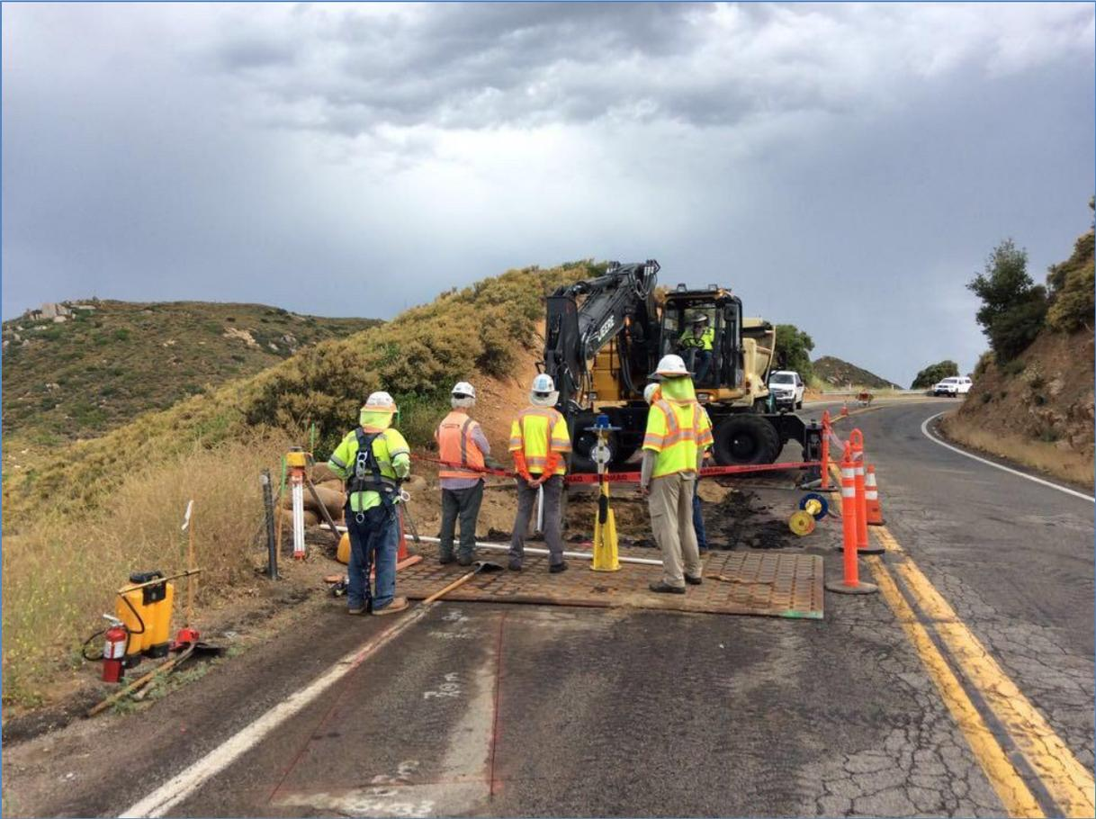
**Photo 4:** A biological, archaeological, and cultural monitor were present during vault excavation (C 440) in accordance with MM BIO-22, MM CUL-1, and APM CUL-04. A complete set of fire tools were staged on site (5-gallon backpack pump, round point shovel, Pulaski, and 2A10BC fire extinguisher) in accordance with the CFPPP (MM FF-1).
