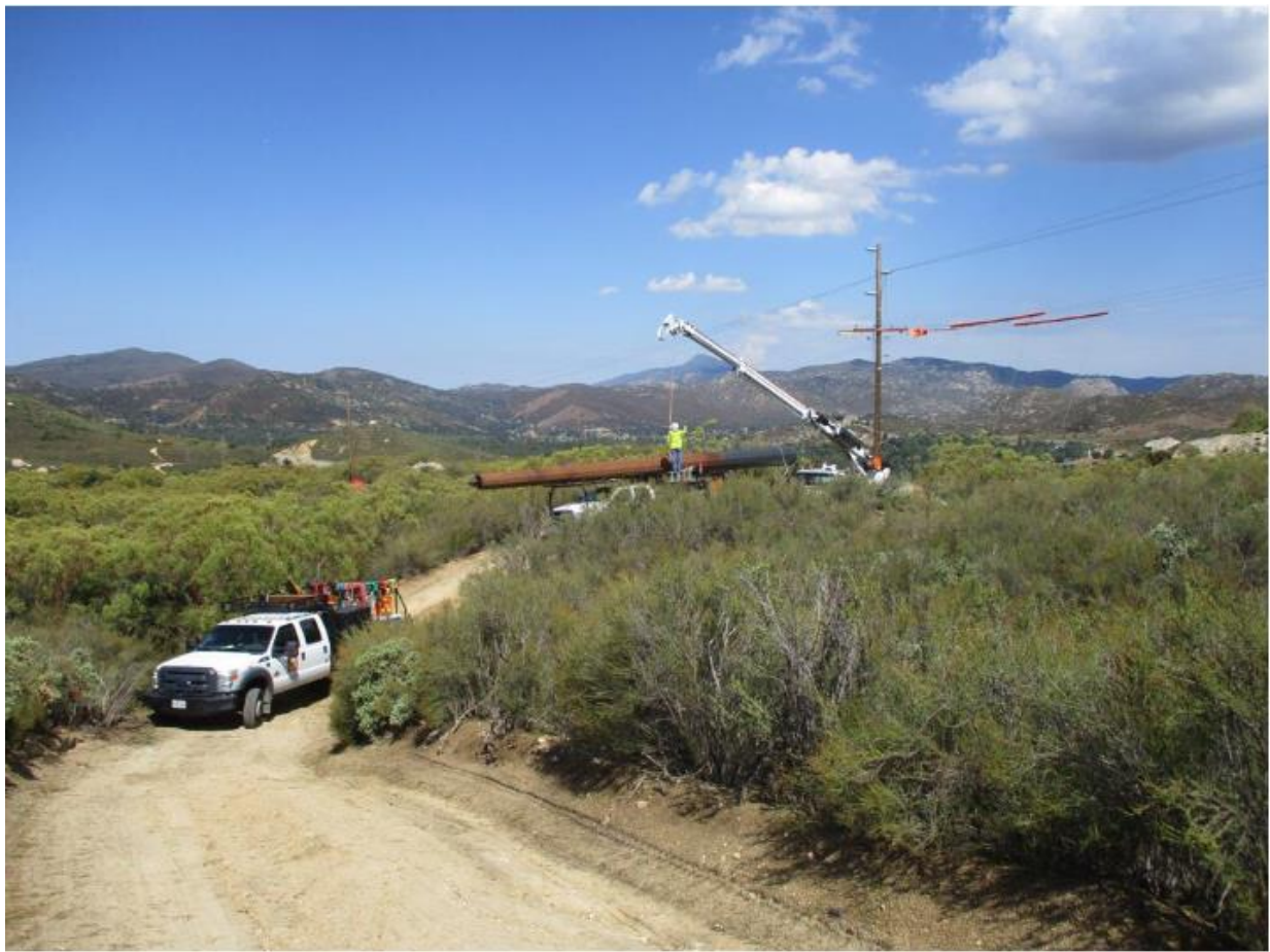
Photo 1: While installing a new pole at Z276646 (TL 629A), equipment was staged within the limits of the approved access road in accordance with MM BIO-1.
