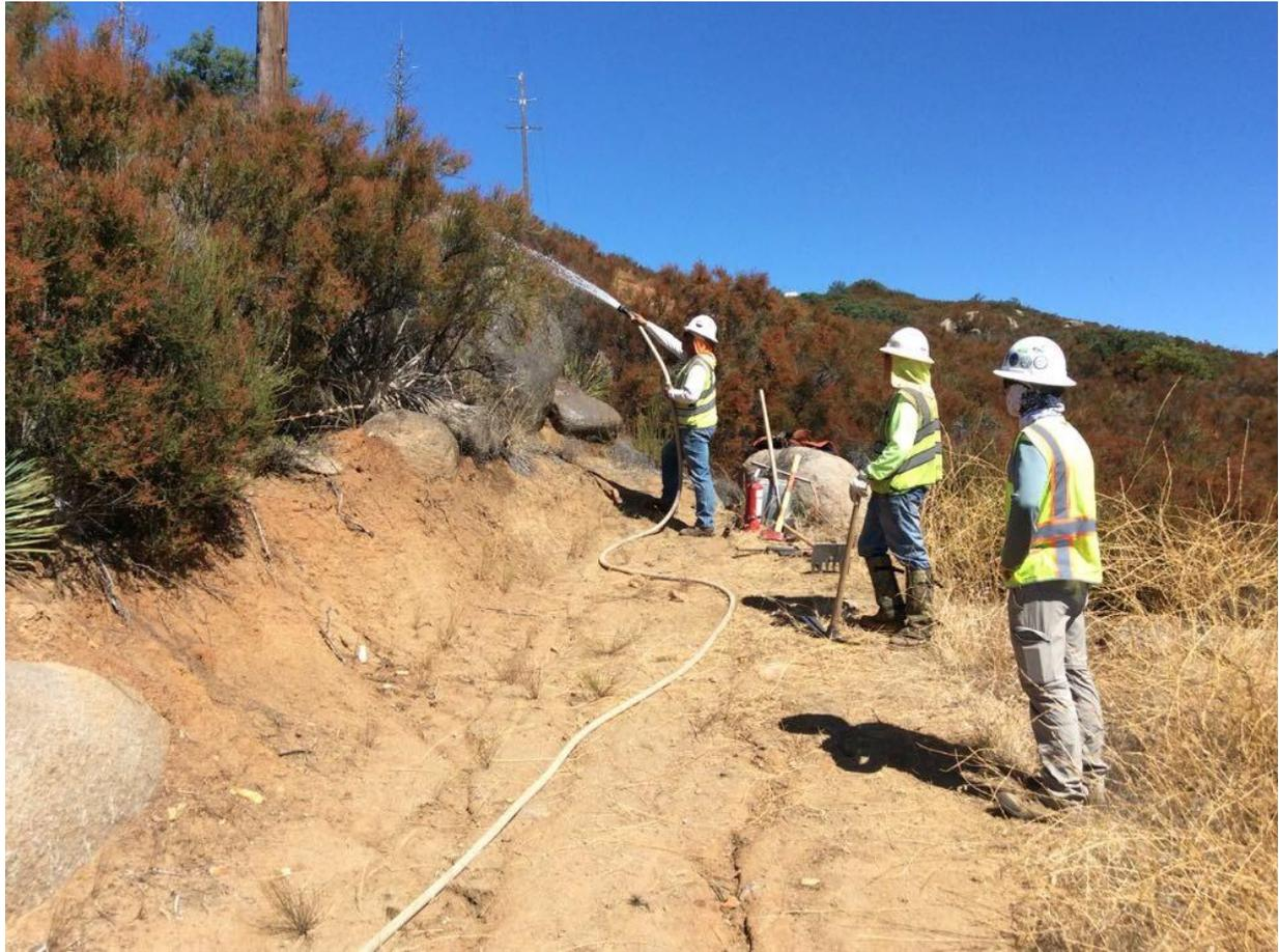
**Photo 4:** In preparation for vegetation clearing and chipping at Pole Z272992 (TL 625C), the area was wet down in accordance with the CFPPP Fire Matrix (MM FF-1) for chipping work on private land with a FPI of Elevated.
