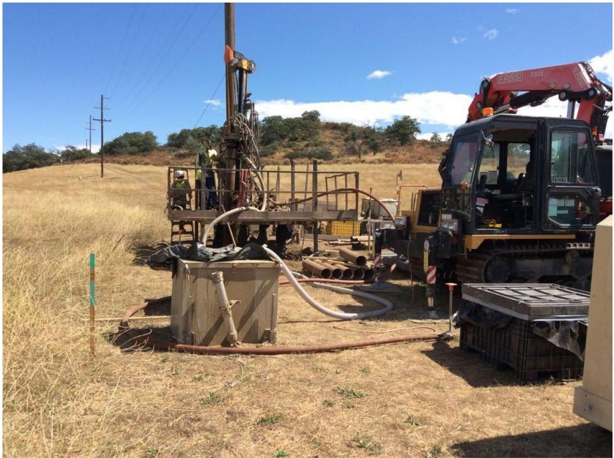
**Photo 1:** During drilling for a micropile foundation at Pole Z272950 (TL 625C), a crew was observed using a containment box to trap drill cuttings and reduce dust emissions from drilling in accordance with APM AIR-05.
