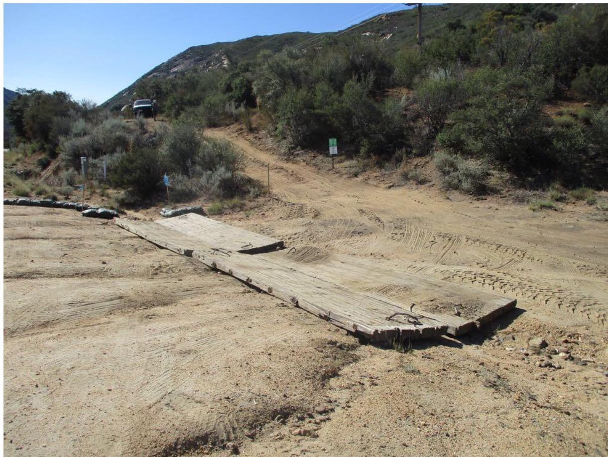
**Photo 5:** During micropile drilling at Pole Z40255 (TL 629A), a jurisdictional drainage crossing along the site access road was flagged, gravel bags were installed, and timber mats were used to prevent impacts to the stream channel in accordance with APM HYD-06.
