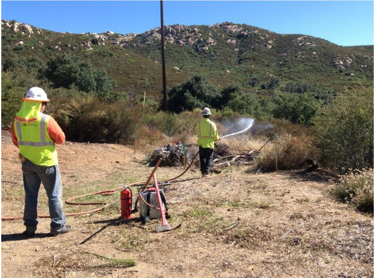
**Photo 4:** In preparation for vegetation clearing and chipping on the access road to Pole P119857 (TL 625C), the area was wet down in accordance with the CFPPP Fire Matrix (MM FF-1) for chipping work on private land with a FPI of Elevated.
