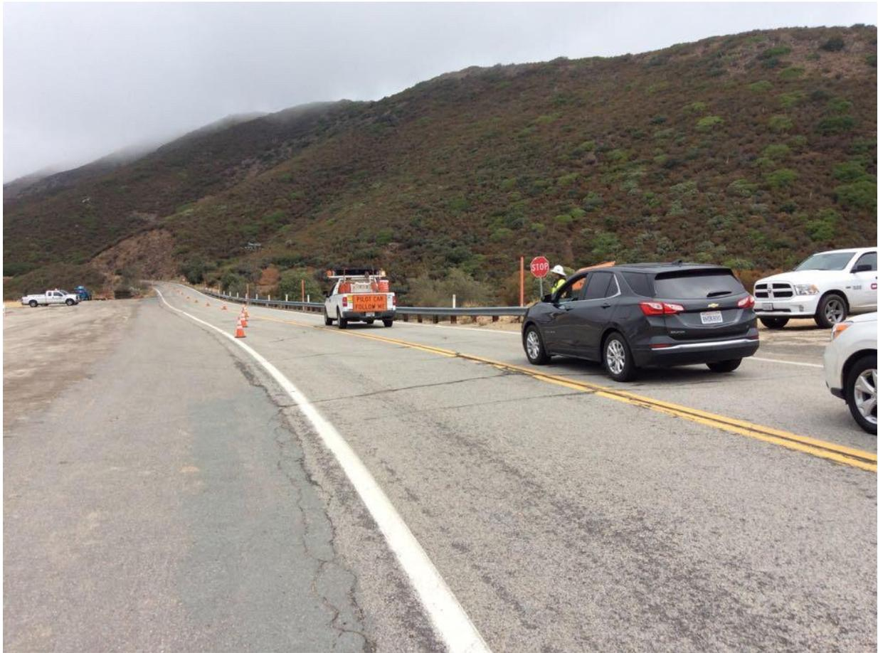
**Photo 6:** A clearly marked pilot vehicle was used to shuttle traffic through the construction zone along Sunrise Highway where one lane was closed for trenching activities (C 440) in accordance with the TCP (APM TRANS-05).
