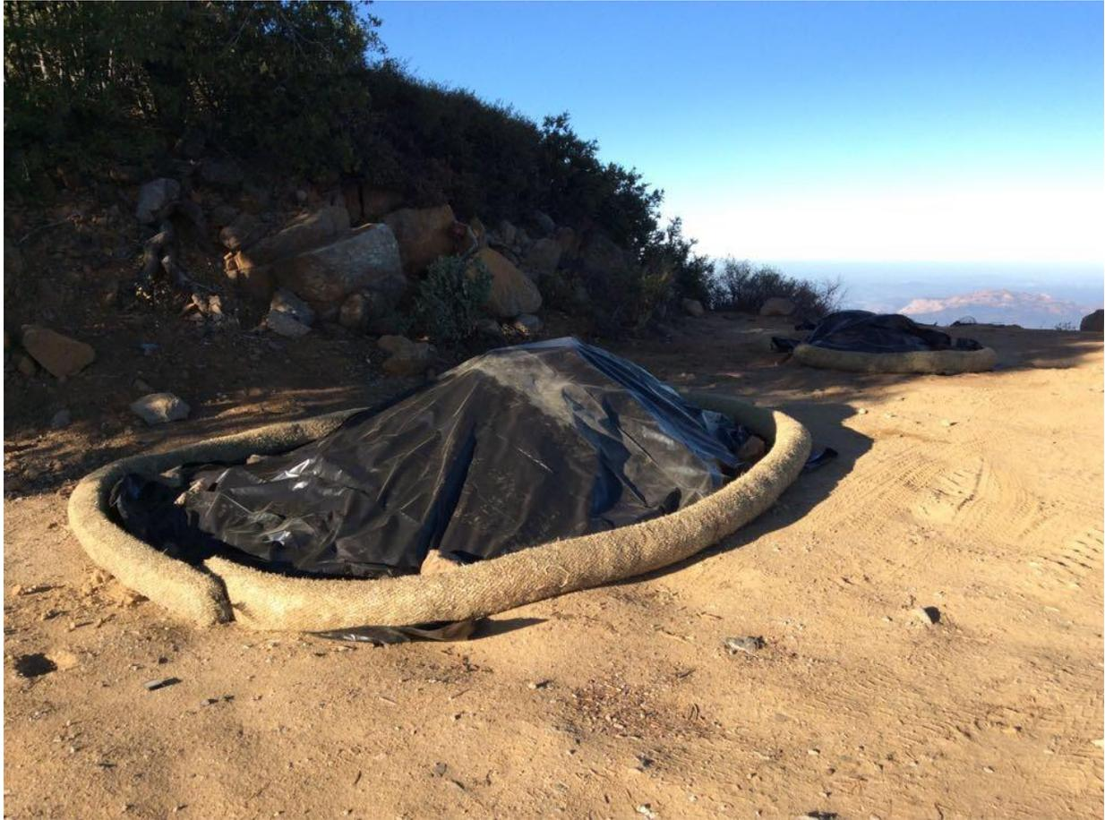
**Photo 5:** Dirt stockpiles staged within a stringing site on Lookout Road (C 79A) were covered with plastic sheeting and surrounded by fiber rolls in accordance with the Erosion Control Plan and Storm Water Pollution Prevention Plan (MM HYD-01, MM BIO-7), and APM HYD-09.
