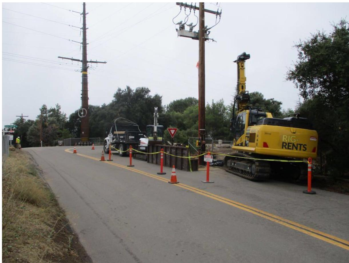
**Photo 1:** During direct bury pole hole drilling at Pole Z172738 (TL 629A), the crew was observed exporting spoils using a haul truck with a load cover in accordance with APM AIR-02.
