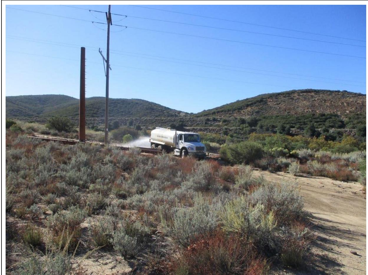
**Photo 1:** Prior to crew ingress into Pole Z276634 (TL 629A), a water truck was observed wetting down the area to prevent dust emissions in accordance with APM AIR-02 and APM AIR-05.
