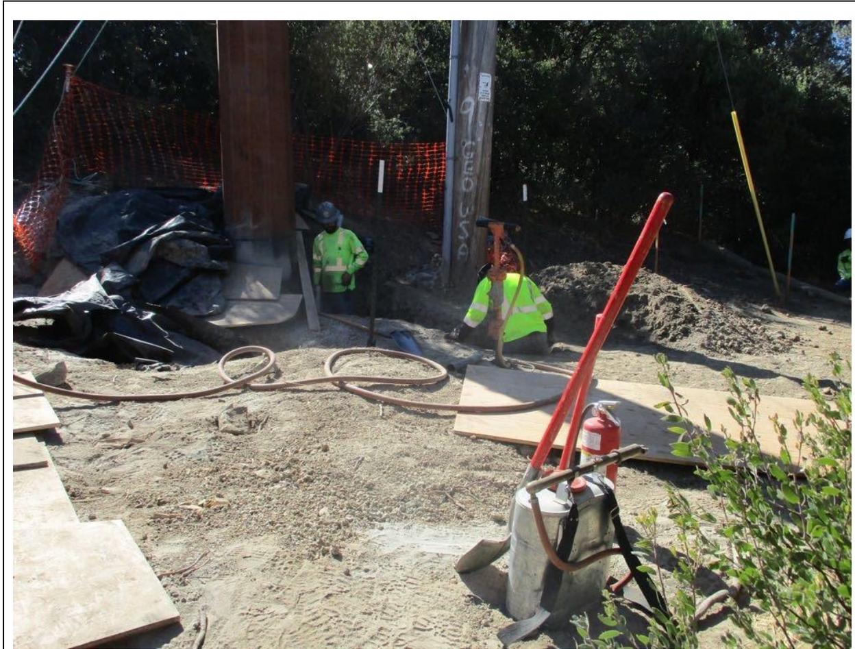
**Photo 4:** During intercept installation at Pole Z172741 (TL 629A), a set of fire tools was observed within 50 feet of the activity in accordance with APM HAZ-04 and the CFPPP (MM FF-1).
