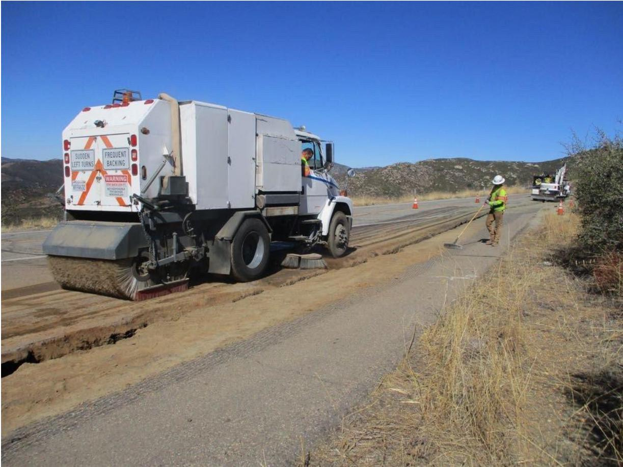
**Photo 6:** After trenching for the underground distribution line at C 440 (Phase 1), a street sweeper was observed being operated along Sunrise Highway to clean the road and prevent off-site erosion in accordance with the ECP (MM HYD-1) and SWPPP (MM BIO-7).
