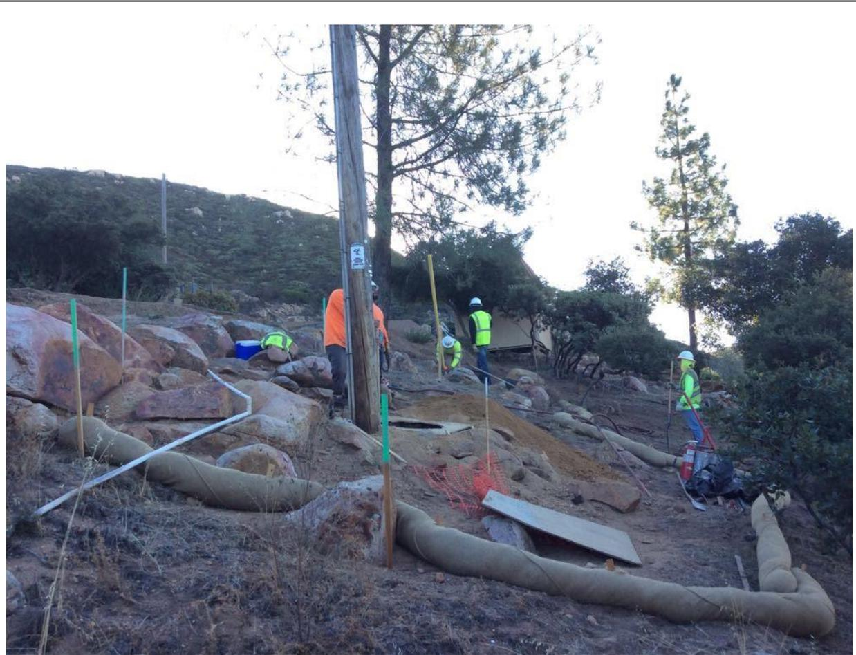
**Photo 2:** During direct bury pole and anchor excavations at Pole P33490 (TL 625C), crews were observed remaining within clearly delineated work limits in accordance with MM BIO-1. SWPPP BMPs were observed in place in accordance with MM HYD-01, MM BIO-7, and APM HYD-09.
