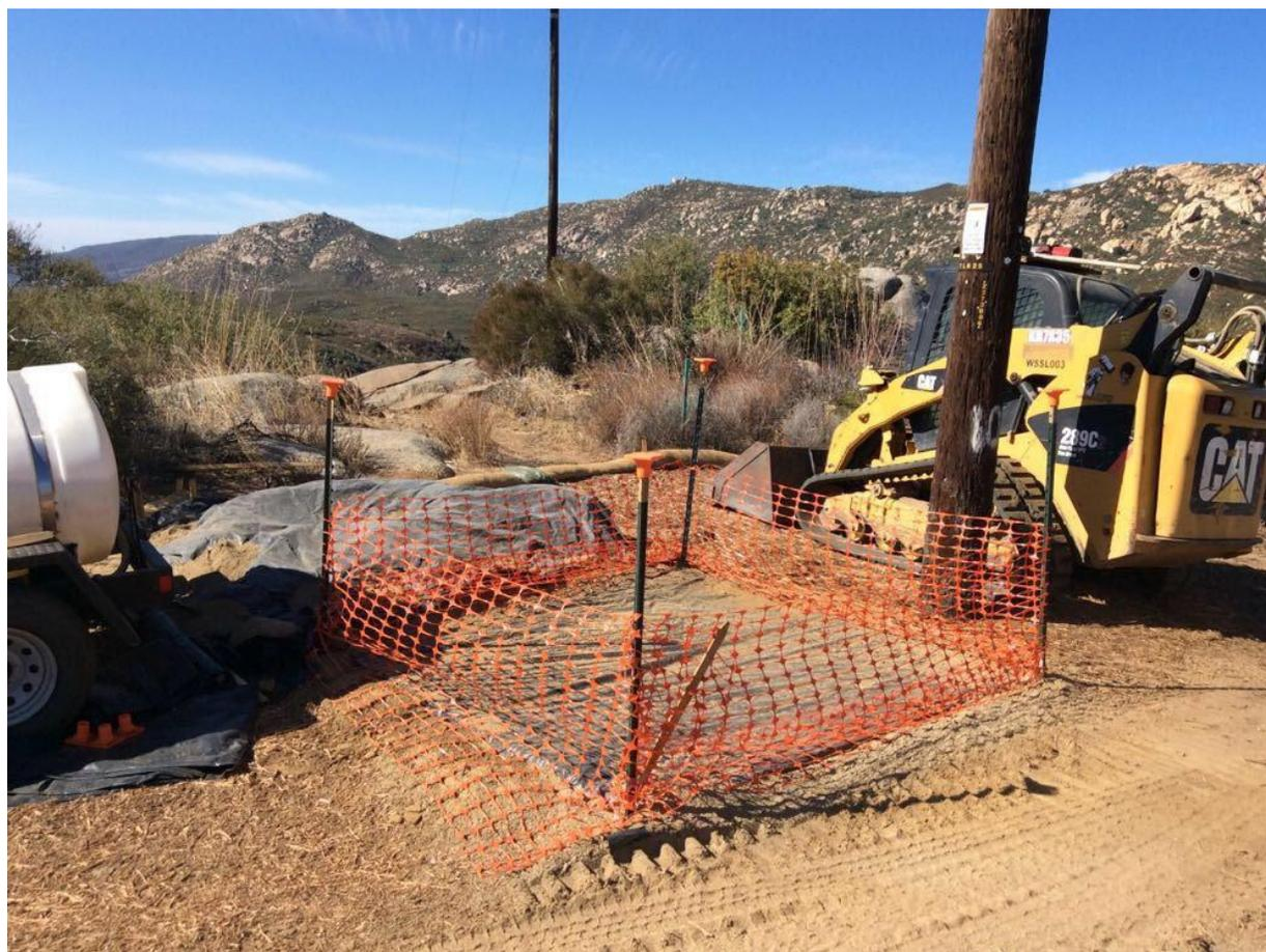
**Photo 2:** The pole hole at Pole Z273006 (TL 625C) was observed to be securely covered to prevent wildlife entrapment in accordance with MM BIO-23.
