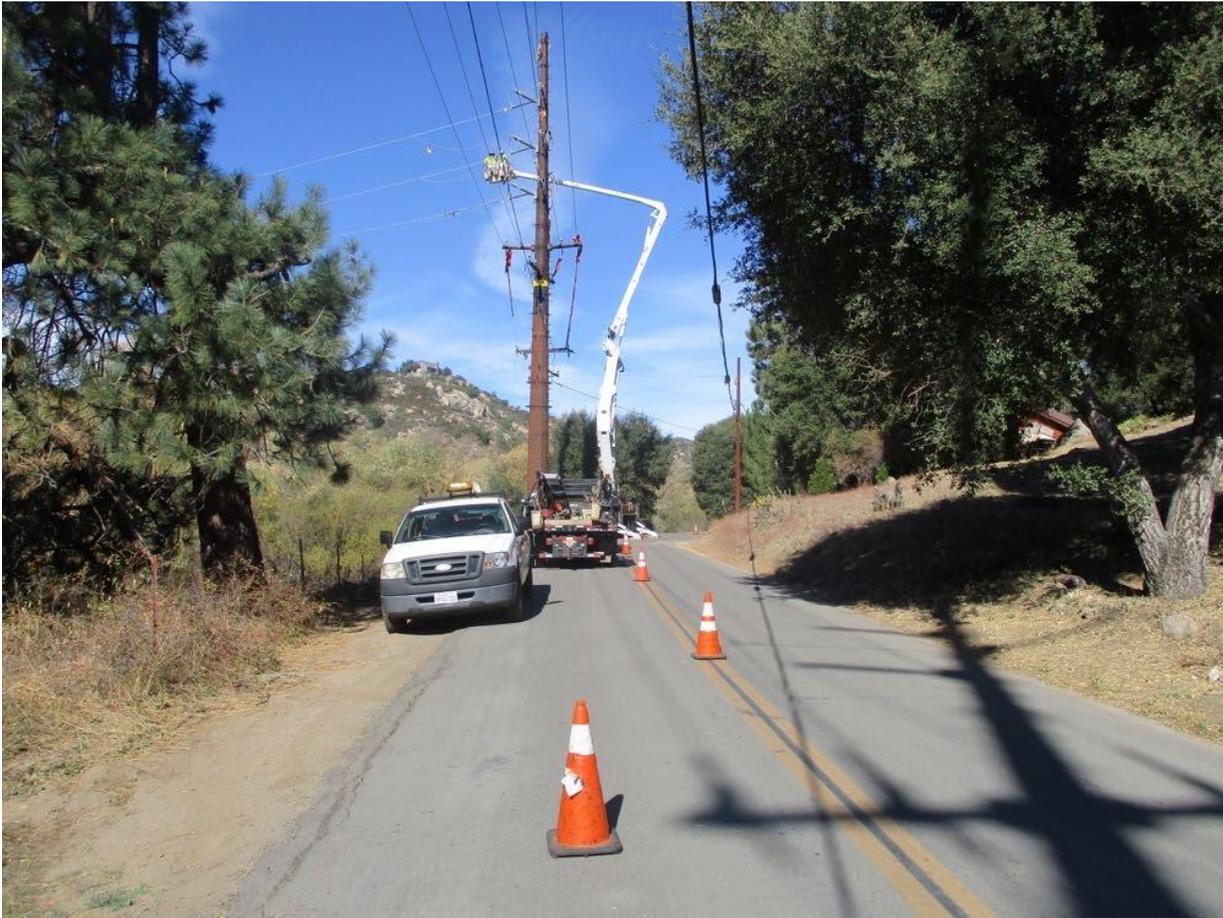
**Photo 6:** During overhead dead-end activities at Pole Z172800 (TL 629A), one-way traffic was directed around the work site with the use of signage, cones, and flaggers in accordance with APM TRANS-02 and APM TRANS-05.
