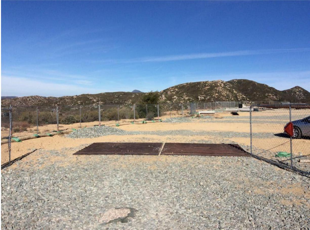
**Photo 5:** The entrance to Staging Yard 2A (C 440) was observed to be stabilized with rattle plates and rock aprons in accordance with project Erosion Control Plan (ECP), SWPPP (MM HYD-01, MM BIO-7), and APM HYD-09.
