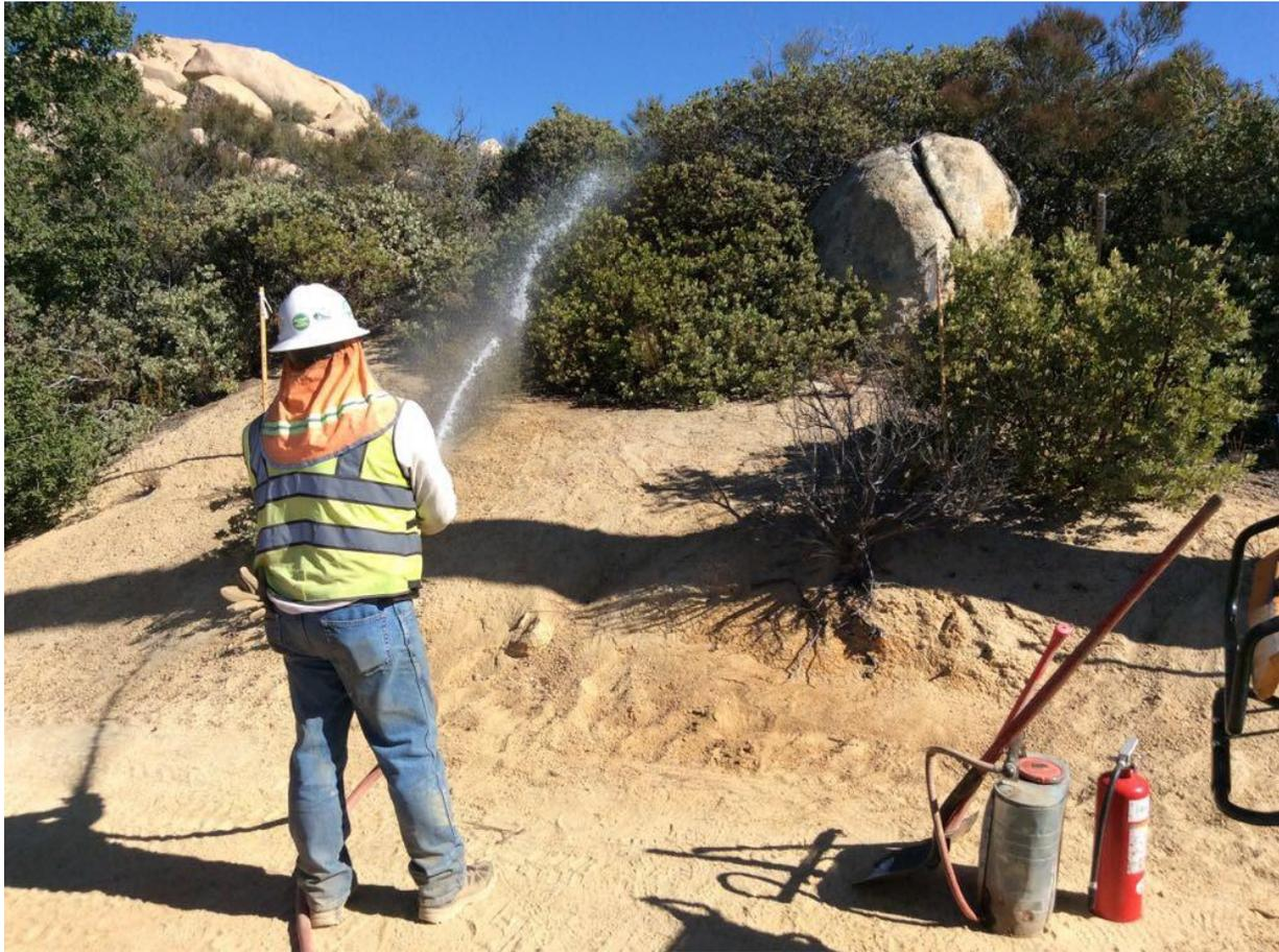
**Photo 4:** A crew member was observed wetting down vegetation prior to removal and chipping at Pole Z273018 (TL 625C) in accordance with the CFPPP Fire Prevention Matrix for the activity on NFS land with a Project Activity Level (PAL) D. In addition, a complete set of fire tools was observed on site.
