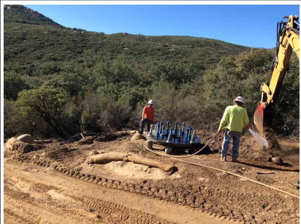
**Photo 1:** A crew at Pole Z293927 (TL 625C) was observed using water to minimize dust emissions during ground rod trenching in accordance with APM AIR-05.
