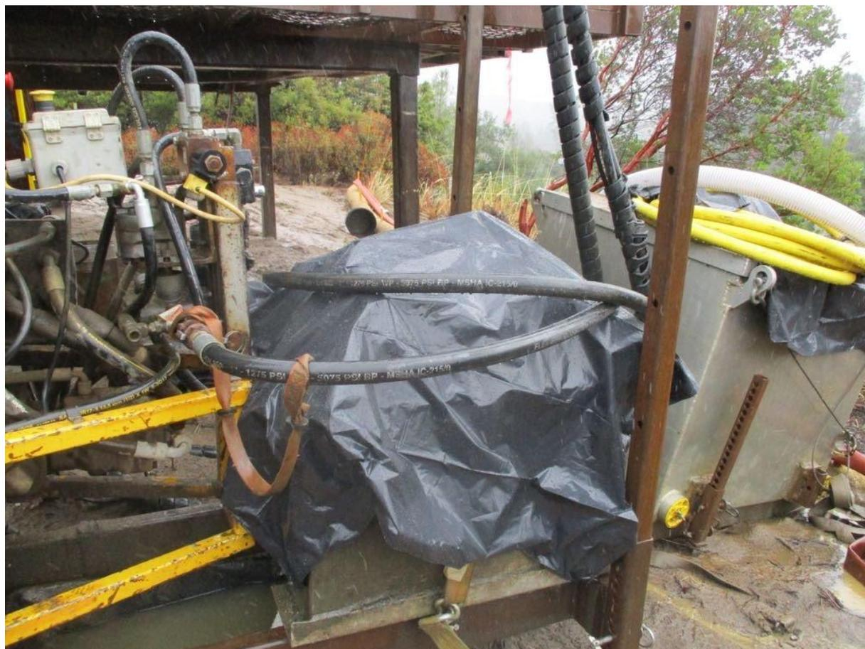
**Photo 4:** In accordance with the SNRP and MM PHS-2, a fuel cell at Pole Z173163 (TL 629A) was observed to be covered during a rain event in order to prevent the containment from filling up and any possible hazardous materials from making contact with the ground.
