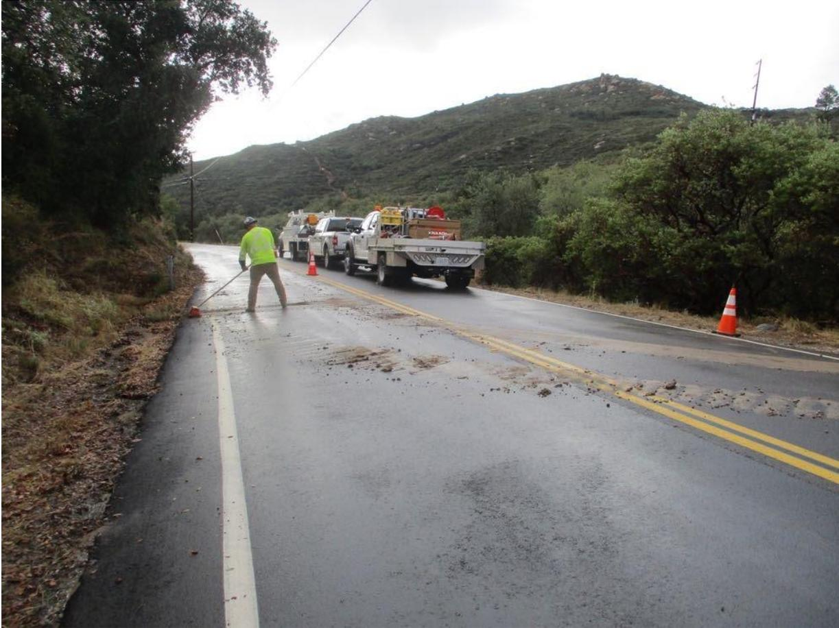
**Photo 6:** In accordance with the ECP and SWPPP, a worker was observed cleaning up trackout left on Viejas Grade Road that was left by drill demobilization. The worker noted that a street sweeper was being mobilized to the area as well.
