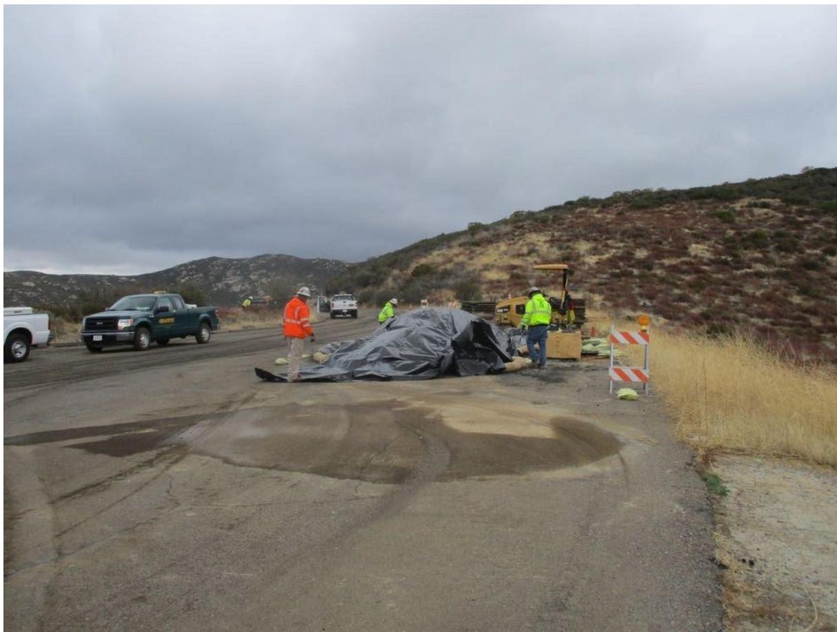
**Photo 5:** Crews were observed covering an asphalt stockpile and securing surrounding fiber rolls at a Staging Area along C 440 in preparation for a forecasted rain event, in accordance with the ECP and SWPPP.
