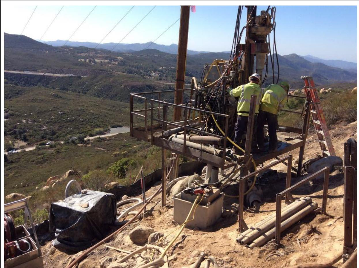
**Photo 1:** A micropile drilling crew at Pole Z273014 (TL 625C) was observed using a covered containment box to trap drill cuttings and reduce dust emissions during micropile drilling in accordance with APM AIR-05.
