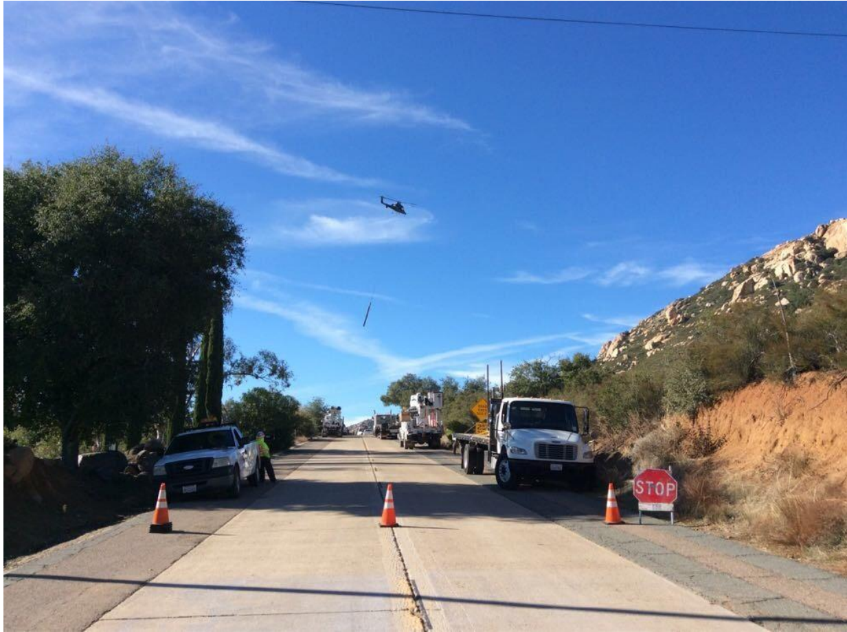
Photo 6: In accordance with the APM TRANS-02 and the Aviation Safety Plan (MM PHS-5), traffic control measures such as cones, signage, and flaggers were observed being used to regulate traffic and prevent the public from accessing Wildwood Glen Fly Yard (TL 625C), where helicopter external load operations supporting pole installation were being conducted.
