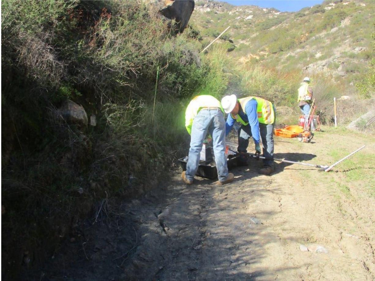
**Photo 4:** A vegetation removal crew was observed using a drip pan while refueling tools at Pole Z571489 (TL 6923) to prevent leaks or spills from being discharged onto the ground in accordance with MM PHS-2 and the SRNP.
