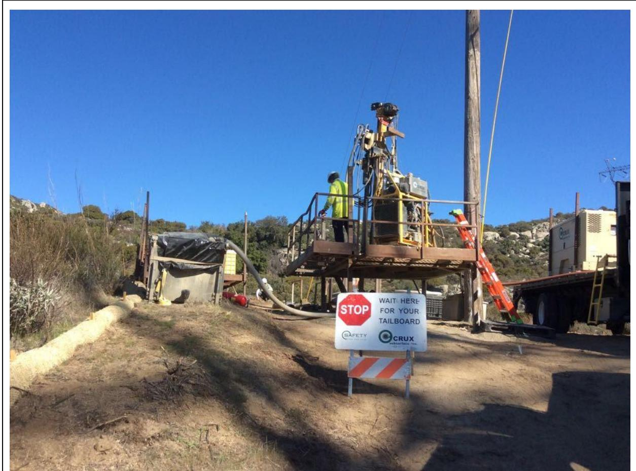
**Photo 1:** During micropile drilling at Pole Z972890 (TL 6923), a containment box was used to trap drill cuttings and reduce dust emissions in accordance with APM AIR-05.
