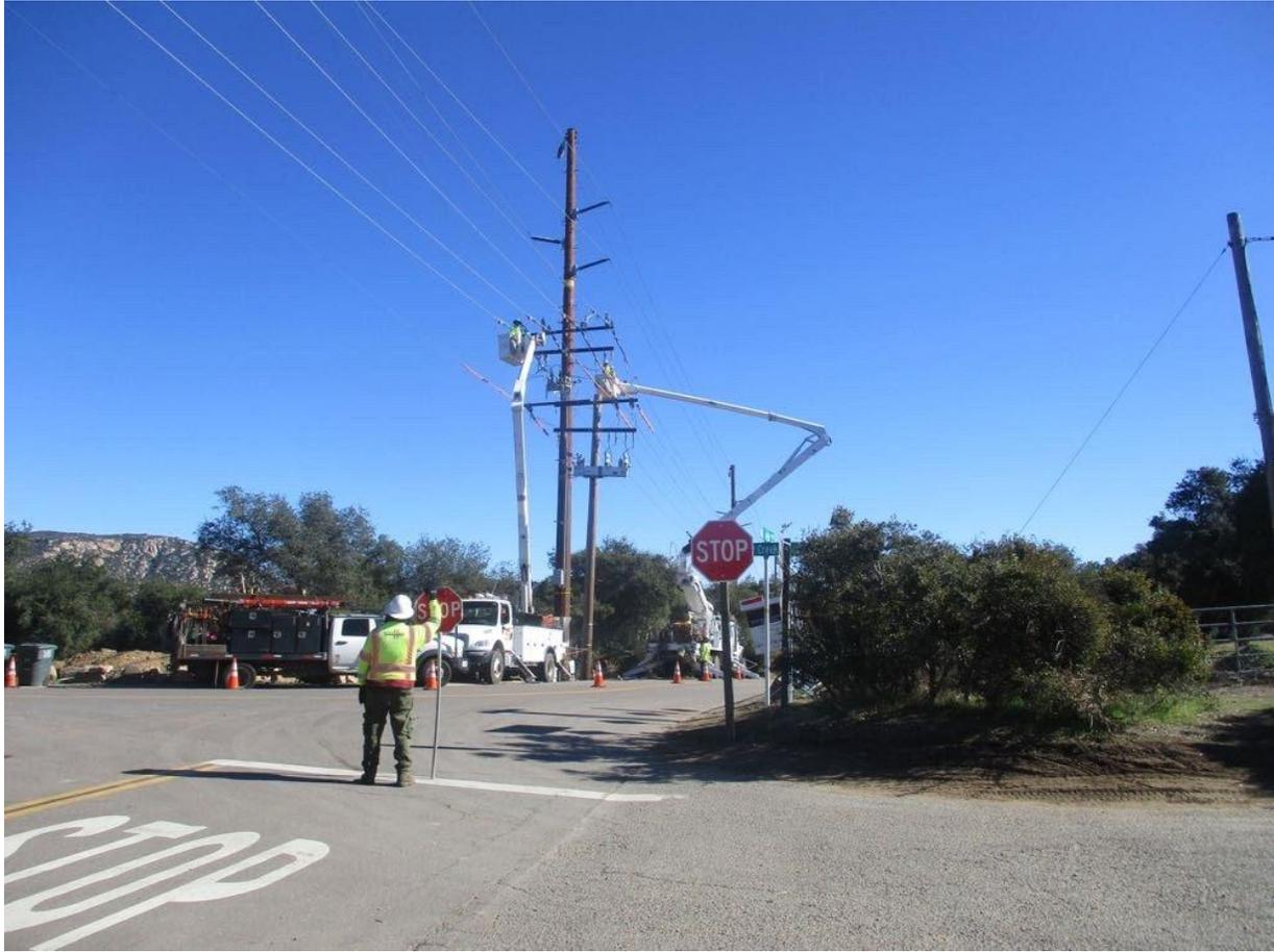
**Photo 6:** During overhead work associated with 12 kV wire stringing at Pole Z172738 (TL 629 A), a traffic control crew directed one-way traffic around the activity on Oak Grove Drive in accordance with the TCP and APM TRANS-02.
