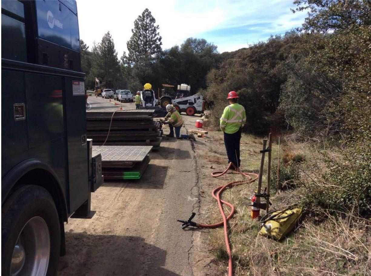
**Photo 3:** A Dedicated fire patrol, equipped with a full set of fire tools (5-gallon backpack pump, round point shovel, Pulaski, and 2A10BC fire extinguisher), was observed monitoring hot work near station 211+20 (C 440) in accordance with the CFPPP. The fire patrol noted that he had also wet down the surrounding area prior to the activity.
