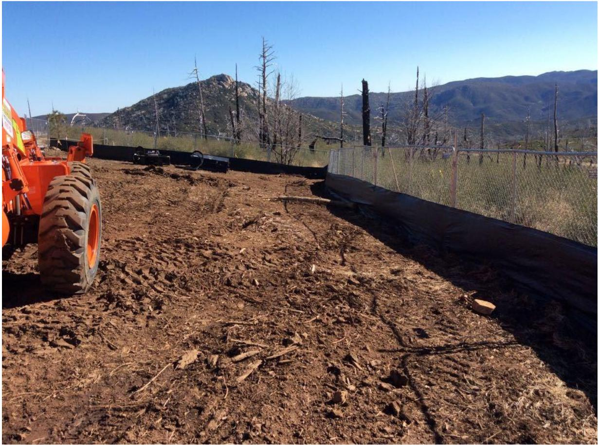
**Photo 5:** Silt fence at Azalea Staging Yard (C 79A) was observed to be in good condition in accordance with the ECP and SWPPP.
