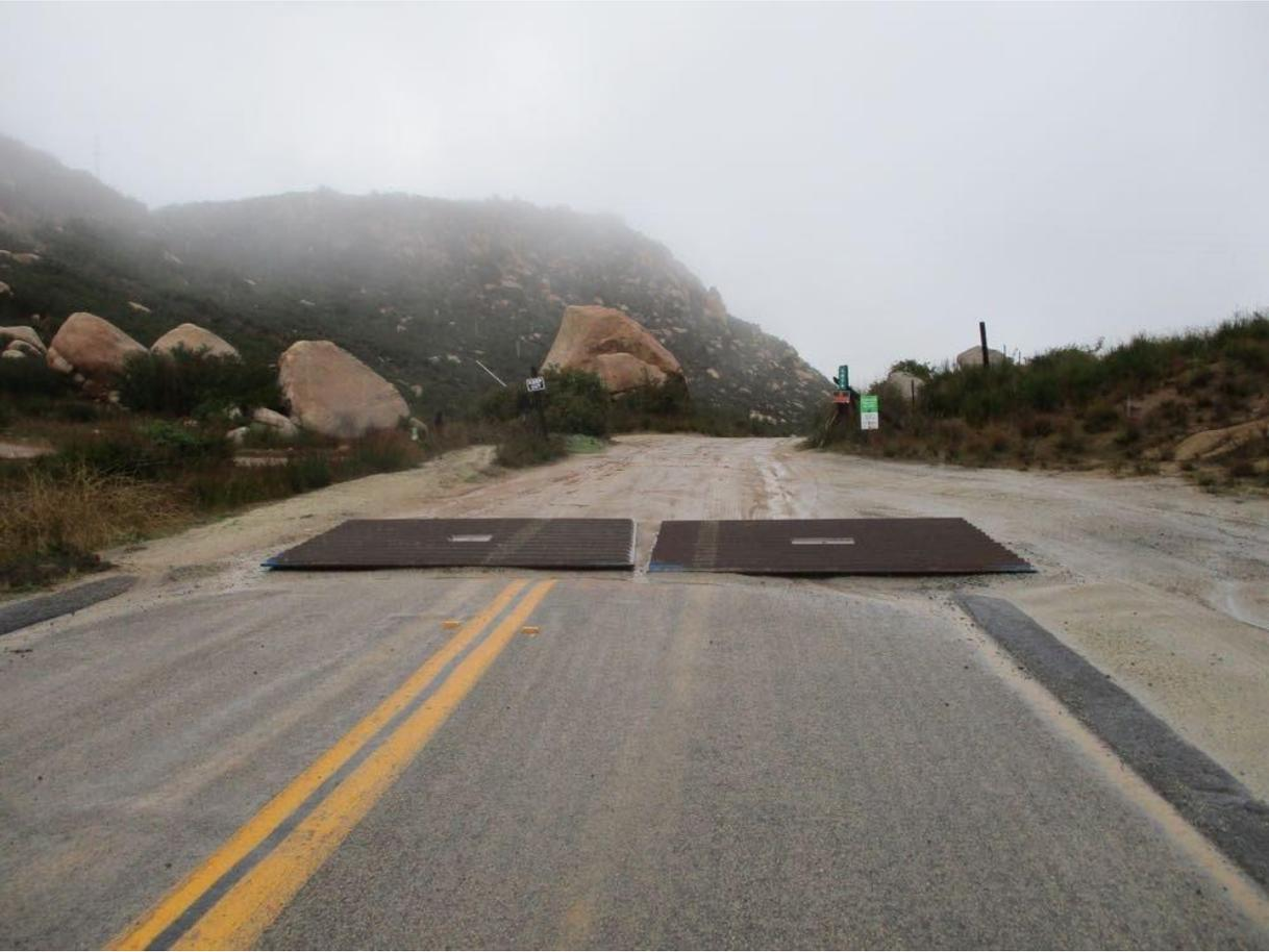
**Photo 6:** Rattle plates were observed at the point of ingress/egress to the Right of Way off Round Potrero Road (TL 6923) in accordance with the ECP and SWPPP.
