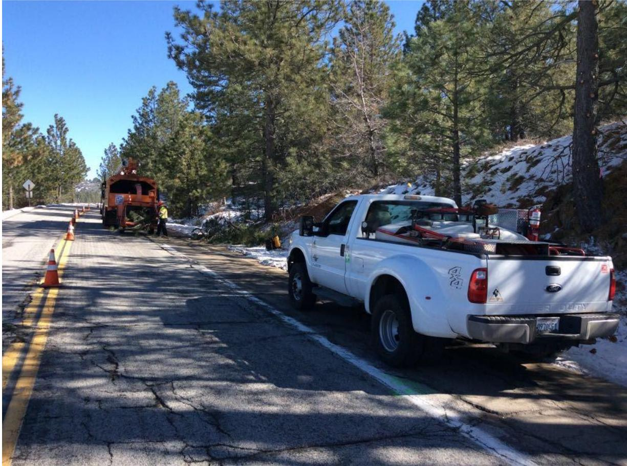
**Photo 5:** During vegetation chipping on Sunrise Highway (C 440), a full set of fire tools was staged within 50 feet of the activity and a Fire Patrol was equipped with at least 100 gallons of water with pump and hose in accordance with the CFPPP specifications for chipping on CNF land with a PAL C.
