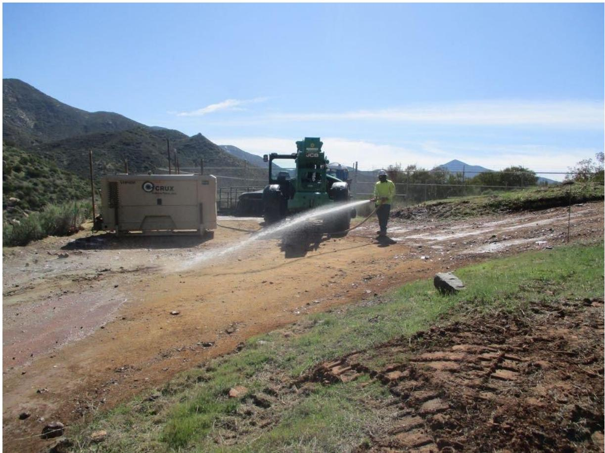
**Photo 1:** A crew member was observed wetting down the work area at Pole Z972788 (TL 6923) prior to helicopter external load operations to minimize dust emissions in accordance with APM AIR-02 and APM AIR-05.
