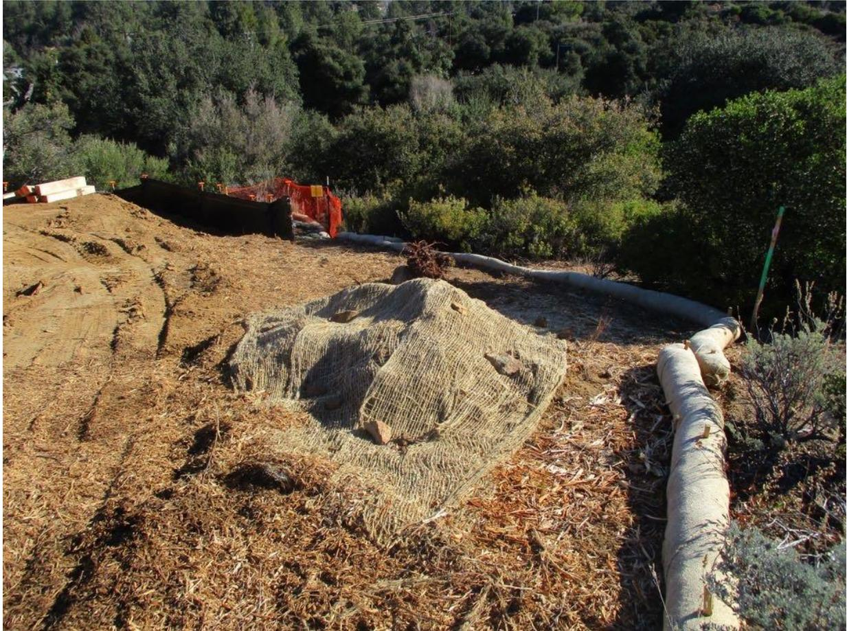
**Photo 3:** Salvaged topsoil was set aside after crane pad grading at pole Z774861. The topsoil will be used for restoration in accordance with the Habitat Restoration Plan and MM-BIO-4.
