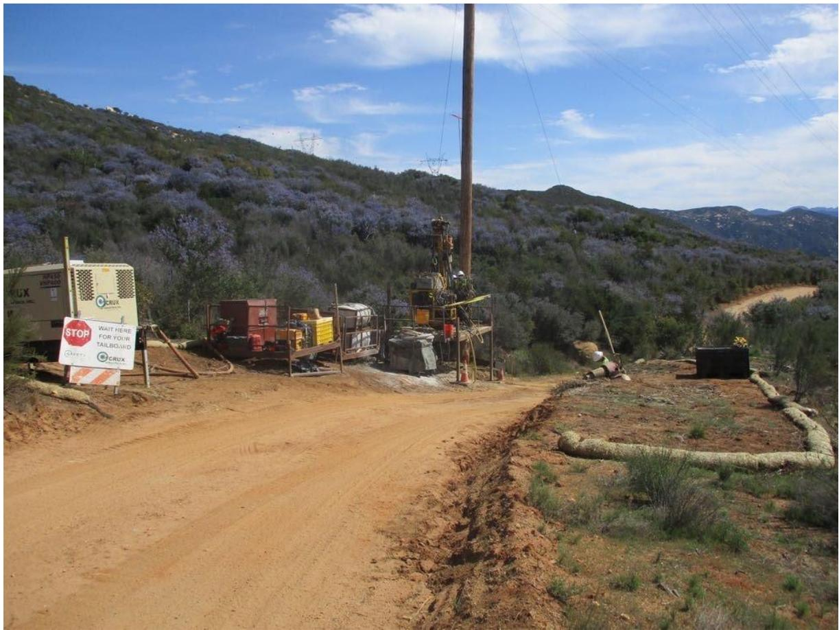
**Photo 1:** During micropile drilling at Pole Z571478 (TL 6923), perimeter erosion control BMPs were observed to be in good condition in accordance with the ECP and SWPPP.
