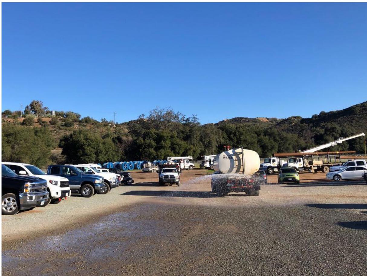
**Photo 3:** Water was applied to the ground at Bookout Staging Yard (TL 625C) to minimize dust emissions during crew egress from the yard in accordance with APM AIR-02.
