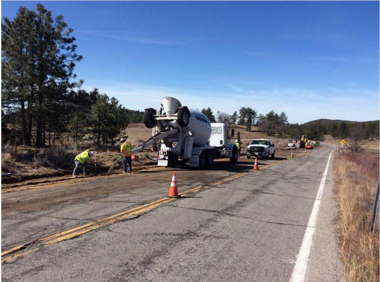
**Photo 2:** Crews were observed trenching, installing conduit, and slurring in the conduit package along Sunrise Highway (C 440). A pilot vehicle was used to lead one-way traffic through the work area in accordance with the Traffic Control Plan and APM TRANS-02.
