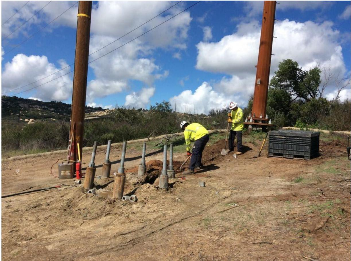
**Photo 1:** During ground rod trenching at Pole Z105011 (TL 6923), a full set of fire tools (5-gallon backpack pump, round point shovel, Pulaski, and 2A10BC fire extinguisher) was observed within 50 feet of the activity in accordance with the CFPPP.
