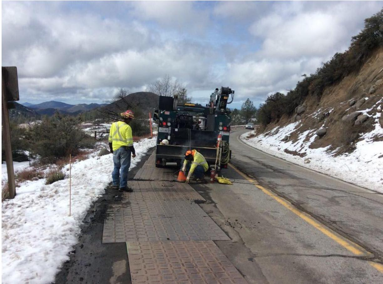
**Photo 4:** In accordance with the CFPPP Fire Matrix for hot work on CNF land with a PAL A, a Designated Fire Patrol was present and a full set of fire tools was observed within 50 feet during welding along Sunrise Highway (C 440).
