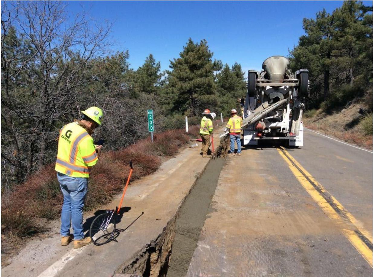
**Photo 2:** Crews were observed slurring in the conduit package along Sunrise Highway (C 440). Crew members were observed displaying hard hat stickers indicating that they had completed project WEAP training in accordance with MM BIO-2.
