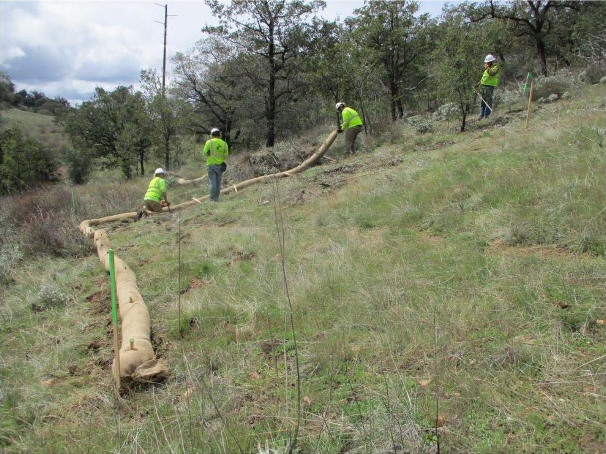
**Photo 6:** A crew was observed installing erosion control BMPs at Pole P259364 (TL 626 Conversion North) in accordance with the ECP and SWPPP.
