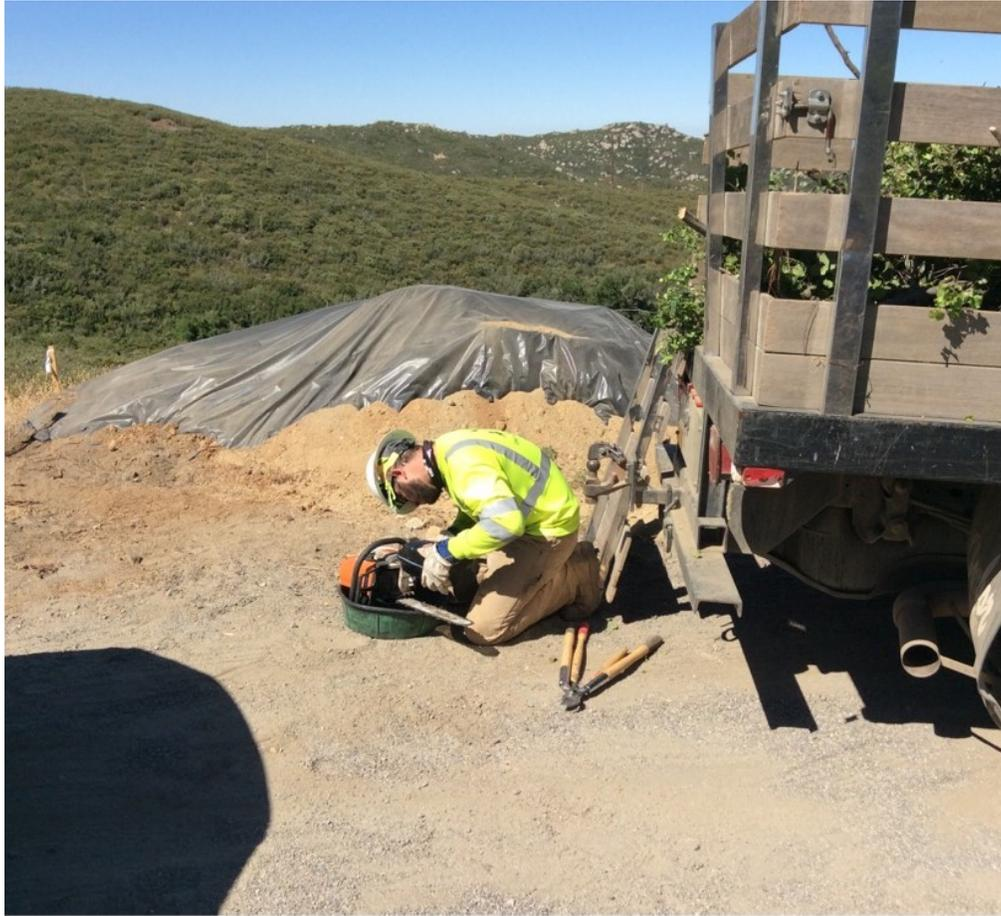
**Photo 5:** A crew member at P259703 (C 79B) was observed using a drip pan while adding oil to the chain saw to prevent leaks or spills from being discharged onto the ground in accordance with MM PHS-2.
