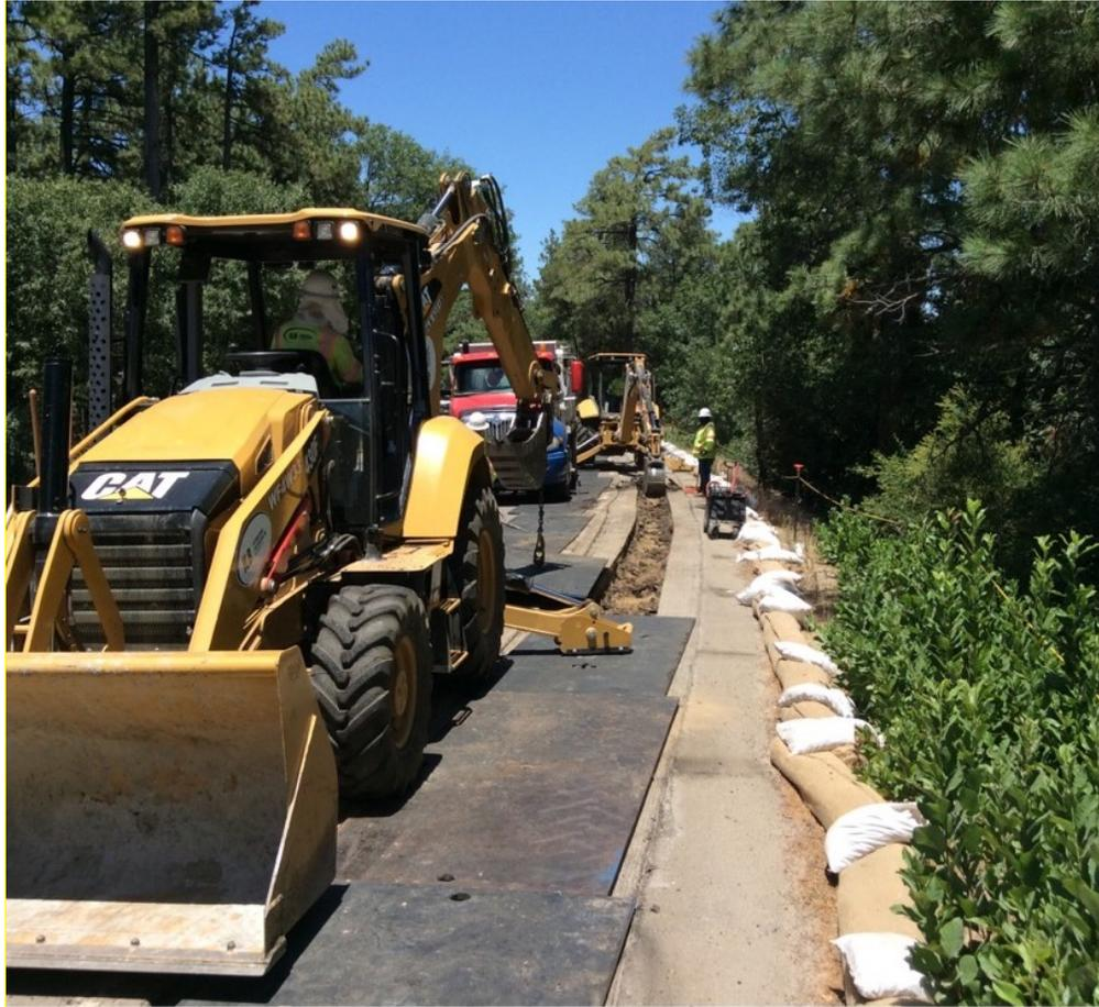
**Photo 6:** A crew was observed stripping asphalt and setting steel plates along C 440. Erosion control BMPs were observed in good condition in accordance with the ECP (MM HYD-1) and SWPPP (MM HYD-1, MM BIO-7). Cultural ESAs were observed avoided by crews in accordance with the HPMP (MM CUL-1) and APM CUL-03.
