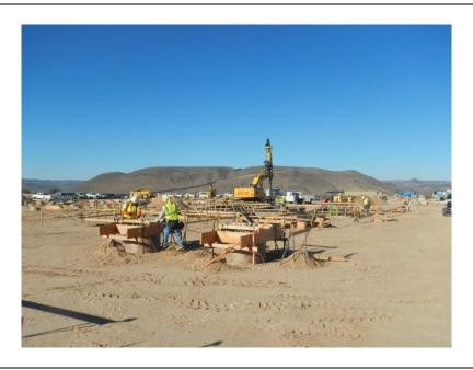
**Photo 1:** Construction crews completing concrete foundations for substation components at the 138/230 kV ECO Substation pad.
