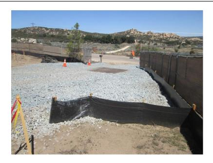
**Photo 4:** Trac-out measures consisting of a rattle plate and rock apron are being maintained at the point of ingress/egress to the Boulevard Substation Rebuild Site along Old Highway 80.
