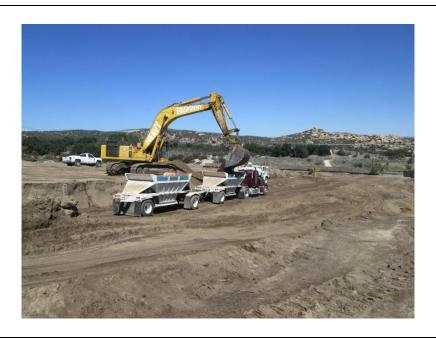
**Photo 3:** An excavator is utilized to load haul trucks to export soil from the Boulevard Substation Rebuild Site.
