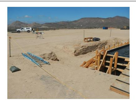
**Photo 2:** Wildlife escape ramps being utilized at the 138/230 kV ECO Substation pad site to prevent wildlife entrapment in accordance with MM-BIO-7A.
