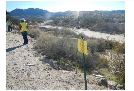
**Photo 4:** Environmentally sensitive areas (ESAs) have been flagged in the field prior to completing geotechnical work in accordance with Mitigation Measure CUL-1.
