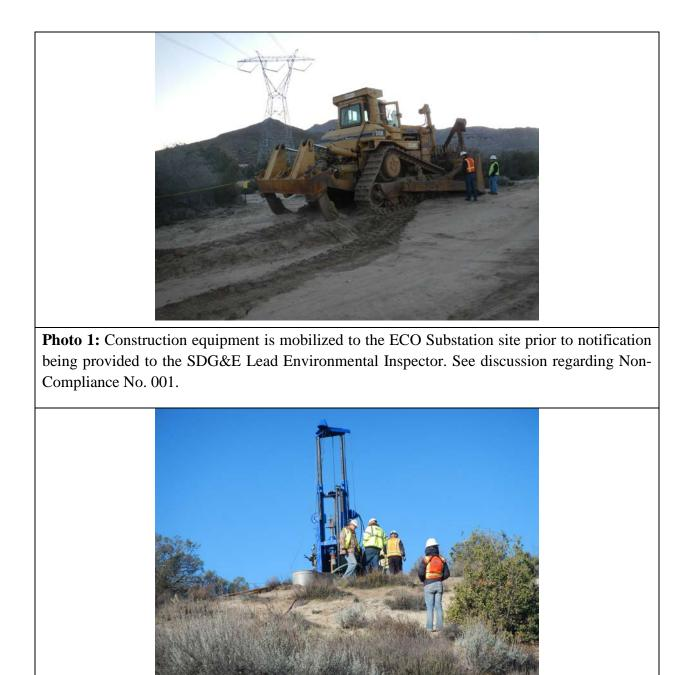
**Photo 2:** SDG&E archaeological and biological monitors observed construction crews using a tracked drill rig to conduct a geotechnical boring at site GEO-11a.
