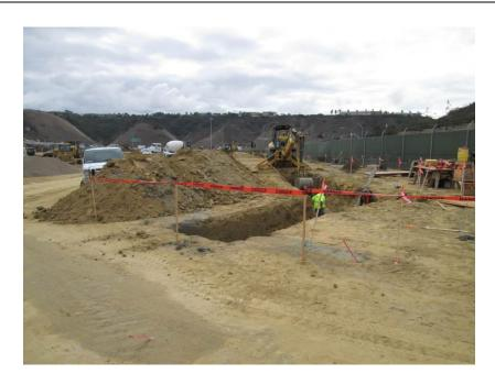
**Photo 1:** Construction continued on the foundation for the perimeter screening wall during this reporting period. The screening wall is being constructed to minimize visual contrast with surrounding areas in accordance with APM-AES-2.
