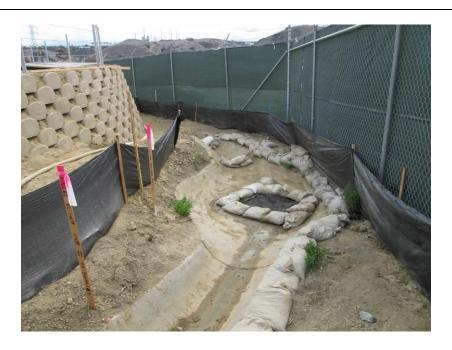
**Photo 3:** In accordance with APM-HYD-1, inlet protection BMP's were being utilized at storm drains located along the project site perimeter and were observed to be maintained in good working order.
