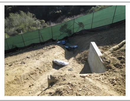
**Photo 2:** In accordance with APM-HYD-1, gravel bag check dams were observed in a drainage canal, and straw wattles, silt fencing, and gravel bags were observed where the canal meets the project site perimeter.
