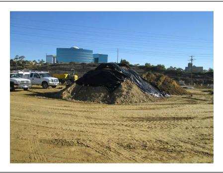
**Photo 3:** Dirt stockpiles were watered and/or covered to minimize or prevent wind erosion and dust creation in accordance with APM-HYD-1
