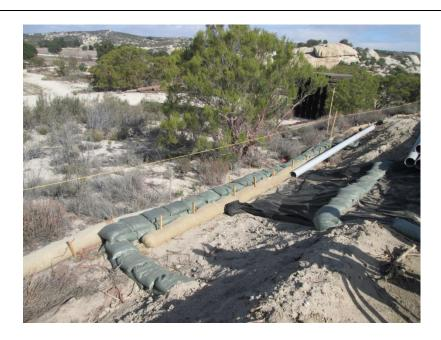
**Photo 3:** Erosion control devices such as straw wattles, gravel bag check dams, and silt fencing were installed along the project right of way in accordance with MM-HYD-1.
