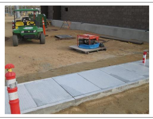
**Photo 8**: In accordance with MM-HAZ-1c, staged equipment, including generators, were equipped with drip pan containment to avoid hazardous materials leakage onto surrounding soil.
