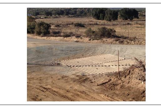
**Photo 1:** Intersections between unpaved access roads and publicly accessed paved roads were equipped with rumble plates to minimize trac-out.
