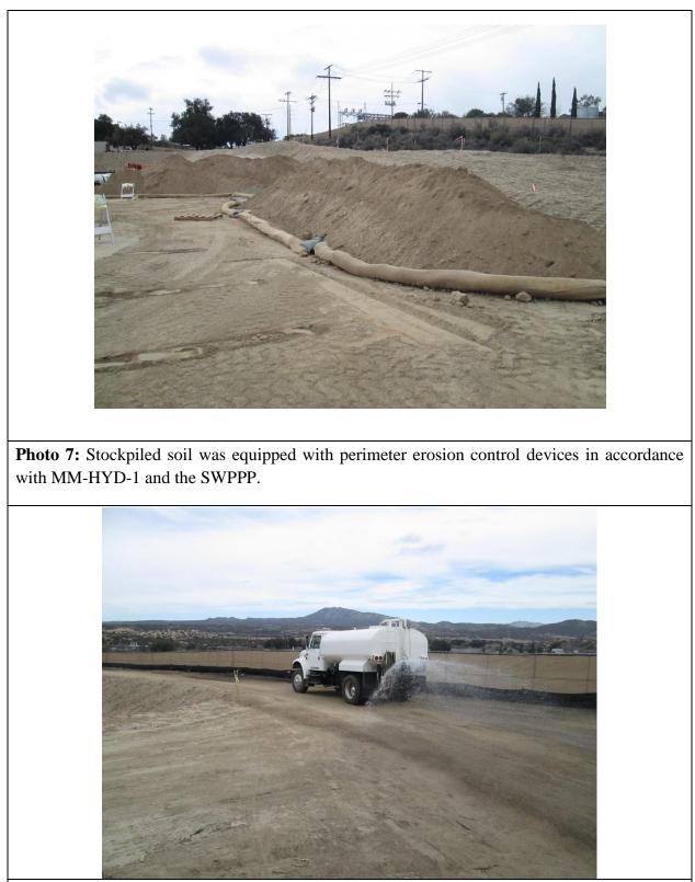
**Photo 8**: In an effort to minimize dust emissions, water trucks were utilized to apply water in areas of active construction at the Boulevard Substation Rebuild site.
