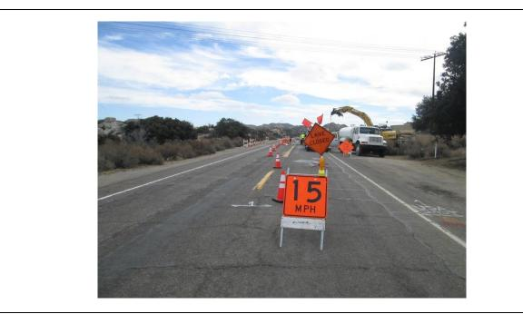
**Photo 5**: In accordance with MM TRA-1, traffic flaggers and posted signage were utilized along Old Highway 80 to ensure safe passage for motorists.
