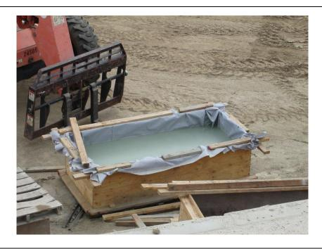
**Photo 6:** As stipulated in the project's Hazardous Materials and Waste Management Plan and MM-HAZ1-a, concrete wash out bins are utilized to contain concrete waste debris.
