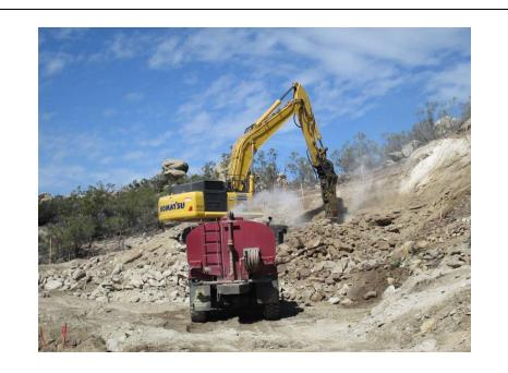
**Photo 3:** As required by MM-BIO-4a and MM-AQ-1, water trucks were utilized to minimize fugitive dust emissions in areas of active construction.
