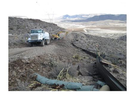
**Photo 4:** Erosion control devices including silt fencing, gravel bags and straw wattles are being utilized along the right-of-way in accordance with MM-HYD-1 and the SWPPP.
