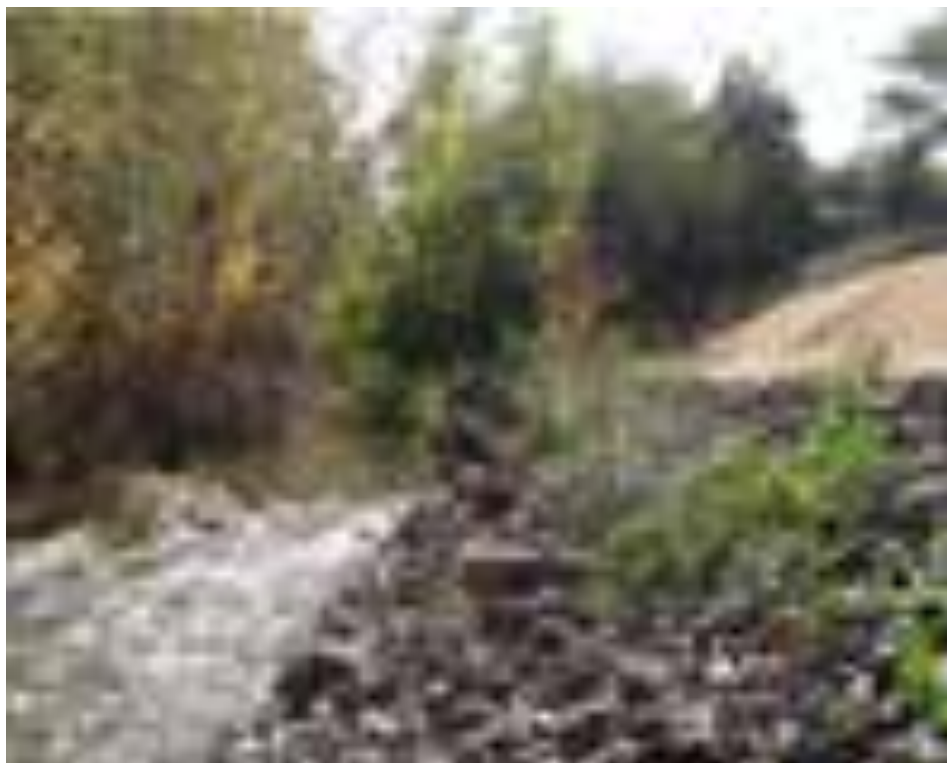
Cobble or gravel armor used for streambank stabilization.
