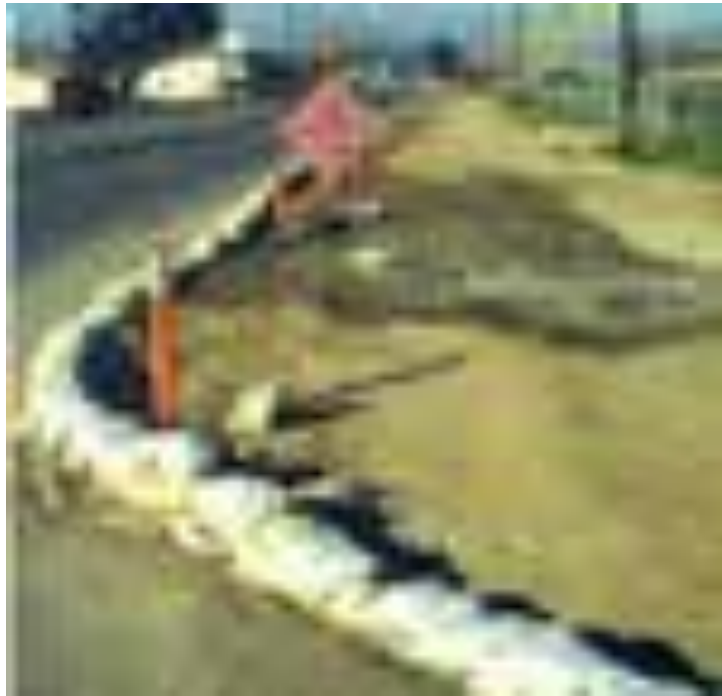
Sand bags used as perimeter control.
