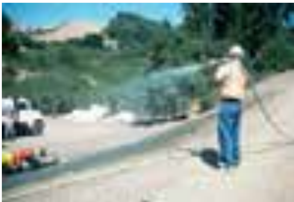
Applying hydroseed.
