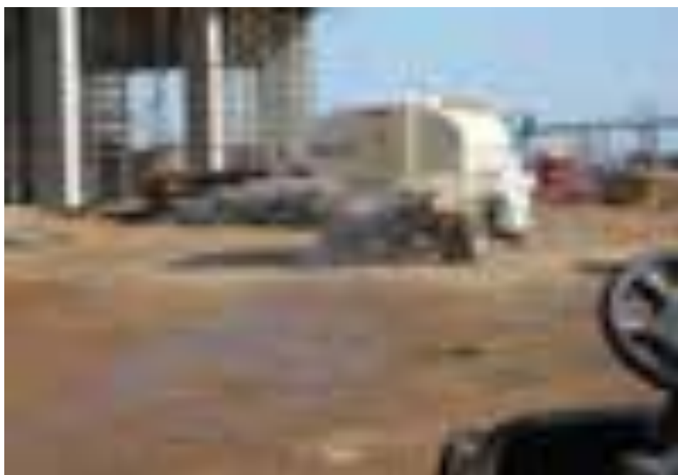
Water being applied for dust control.
