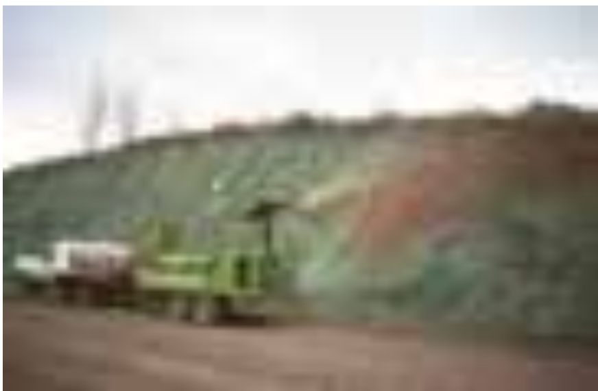
Applying a tackifier using a trailer mounted pump and hose.
