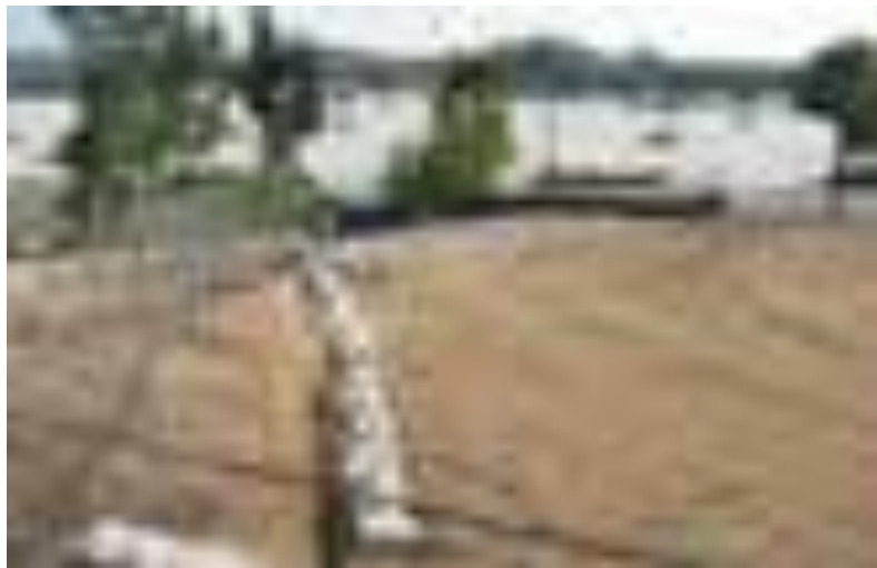
Gravel bags used as perimeter control.
