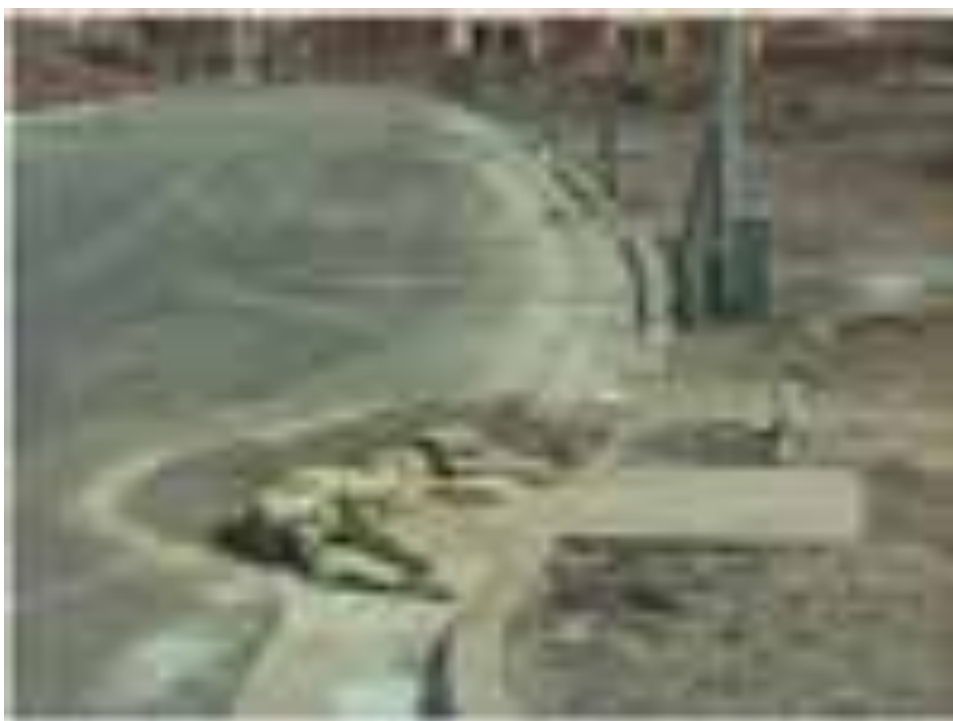
Gravel bag inlet protection.
