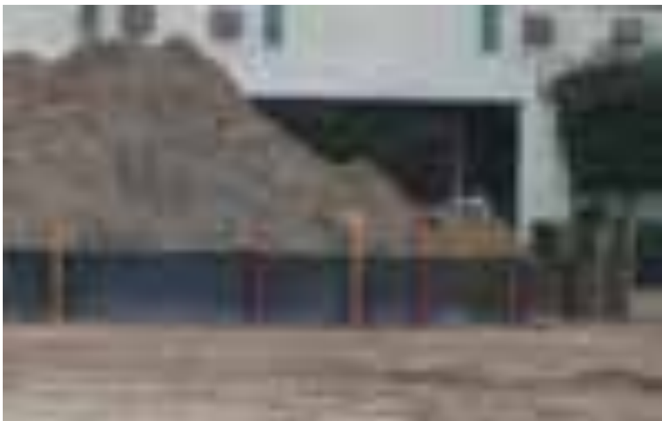
Silt fence used for stockpile perimeter control.
