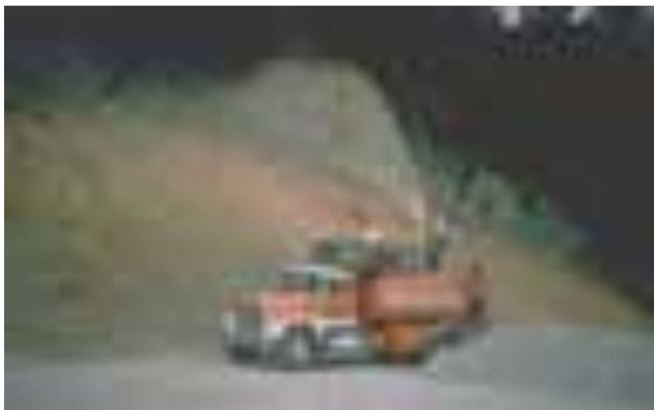
Applying hydraulic mulch.
