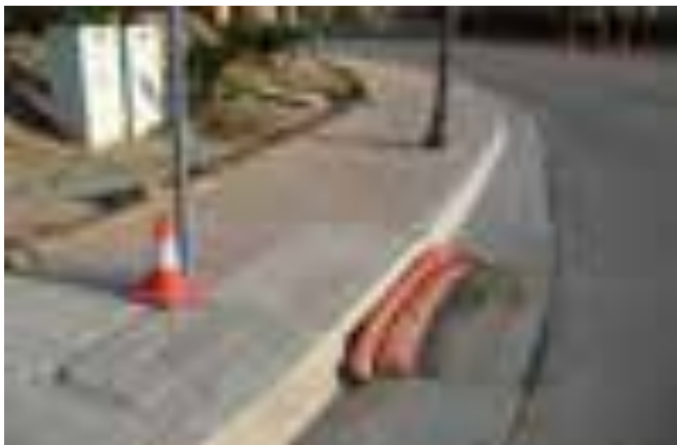
Inlet protection that blocks flow, preventing non-storm water discharges from entering drain.
