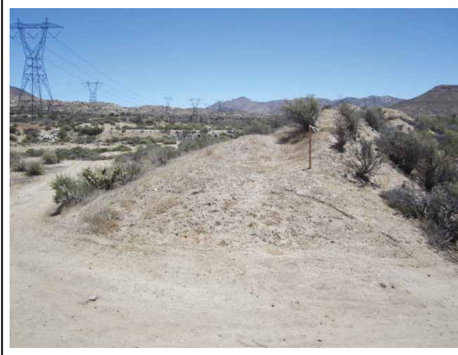
Photograph 7: View of relocated riser pole SP-91B site facing east.
