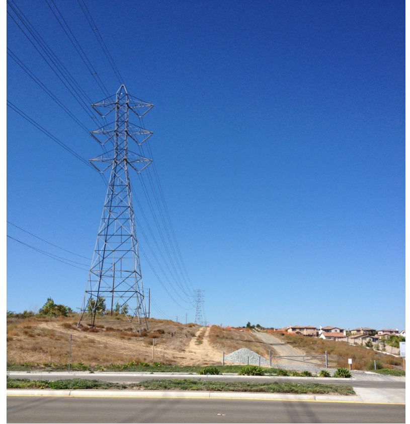
Transmission line corridor looking north
