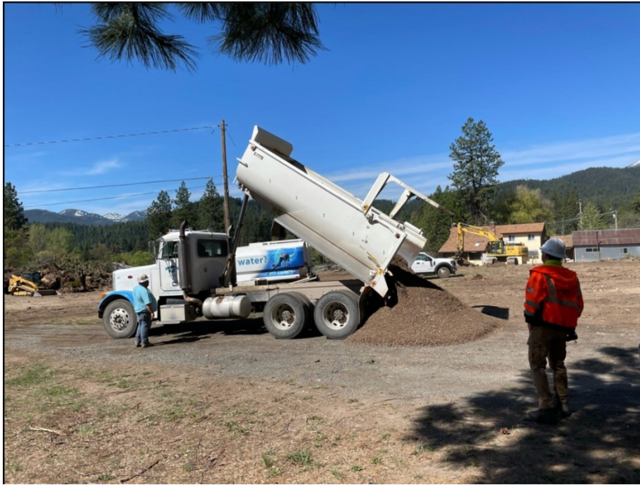
Photo 3: Base gravel for the new substation delivered on site.
