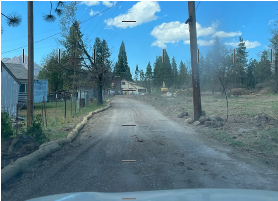
Photo 4: SWPPP BMPs (fiber rolls) were placed along access roads in accordance with APM WQ-1.
