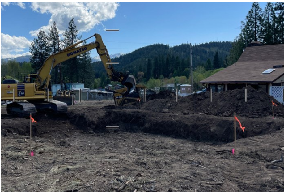
Photo 2: Crews excavated an area on site for a new substation transformer.
