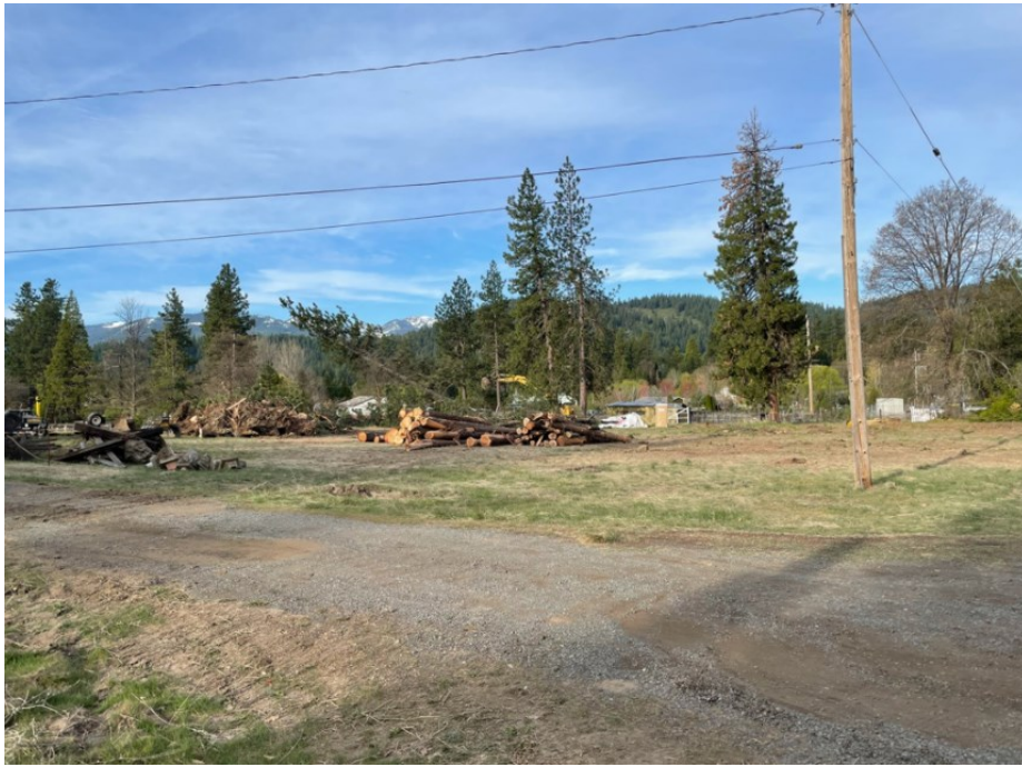
Photo 1: Tree removal at the new substation location was observed.
